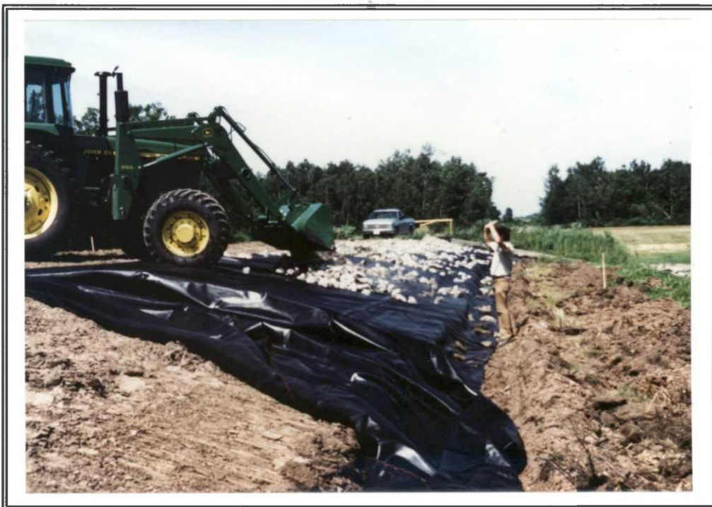
Most of the summer was spent repairing dikes/spillways lost this spring. Oneida dike was repaired in July. Filter fabric was placed on the dike prior to rip rapping. DVT 7-8-93
