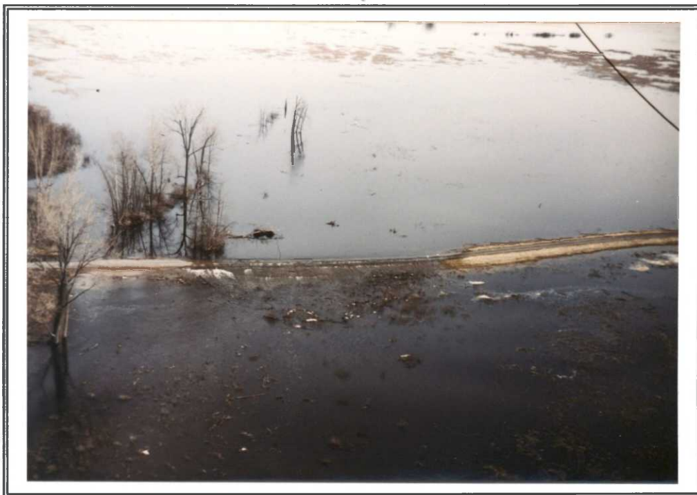
Our new Cayuga Pool water control structure nearly was lost in the spring flooding. The spillway functioned properly but was damaged.
