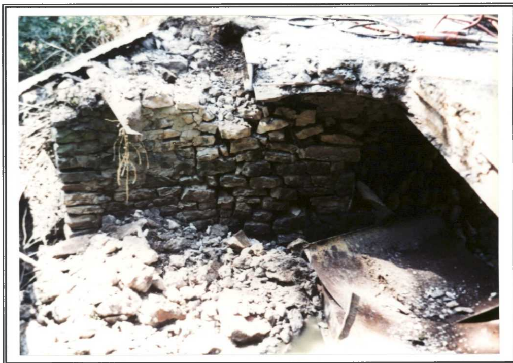
A bridge on Feeder Road was in an impassable state and was replaced.
