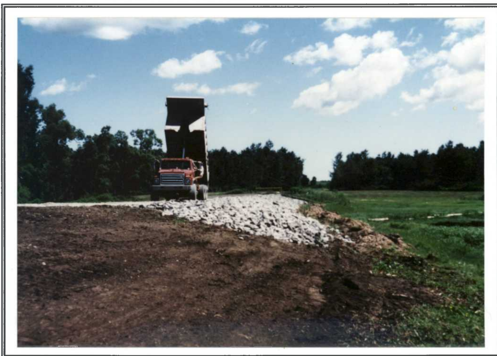
After large stone was placed on the slope, stone was added to the top of the dike. DVT 7-23-93
