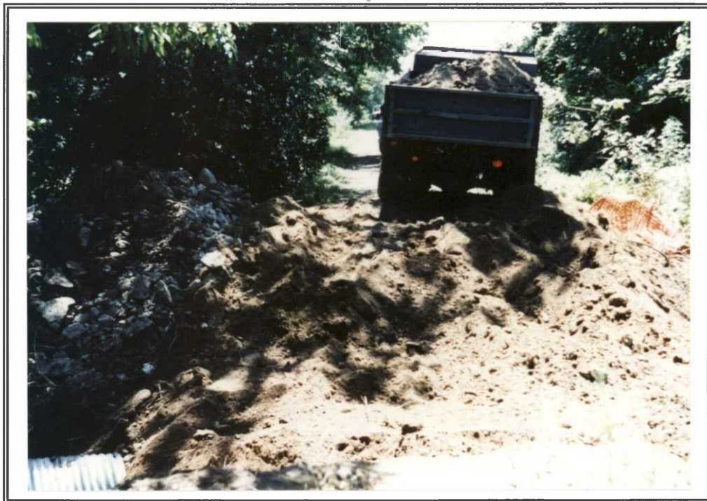
Two four' CMP were installed in it's place.
