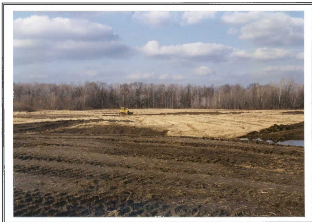
One ditch plug and more than forty "potholes" were constructed in the Forrestel Flats area.
