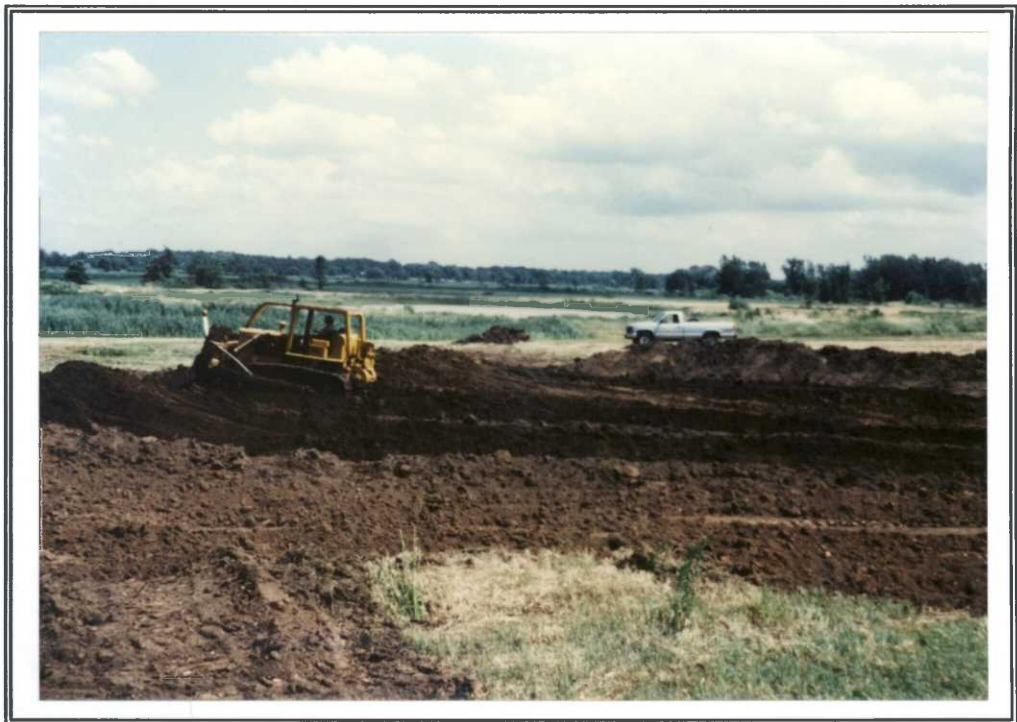
Three ditch plugs were constructed near the Olsen Marsh, south unit, in the surrounding grasslands.
