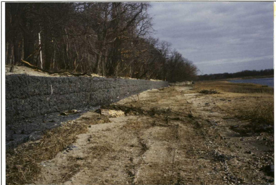
Section of groin put in by the Nassau County Department of Public Works to shore up damaged areas of West Shore Road on the border of the Refuge. RWP-1993
