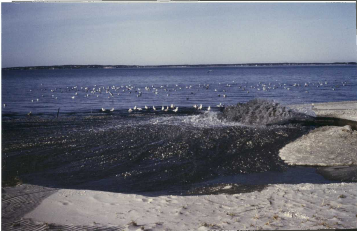
Sediment, largely sand, being deposited from the dredge's outfall pipe on a portion of the Refuge beach. RWP-93
