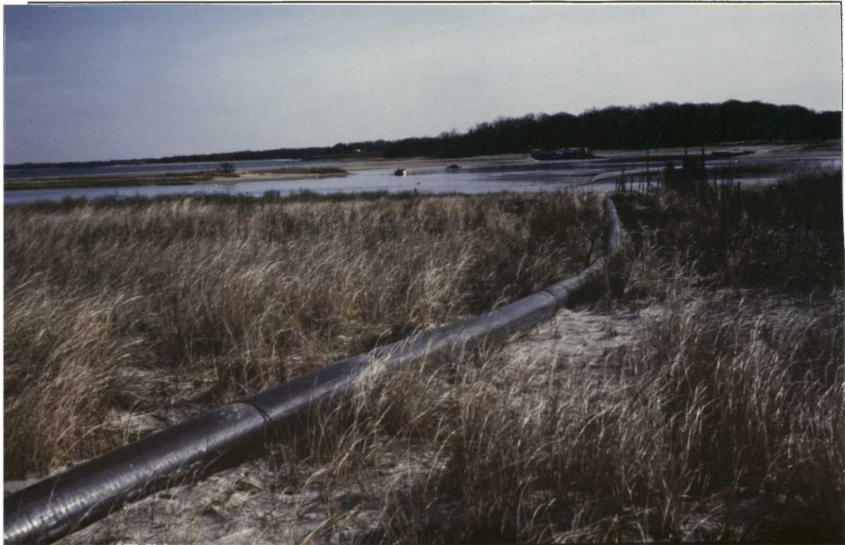
Suffolk County's suction dredge in Noyac Creek and outfall pipe crossing the Refuge. RWP-93
