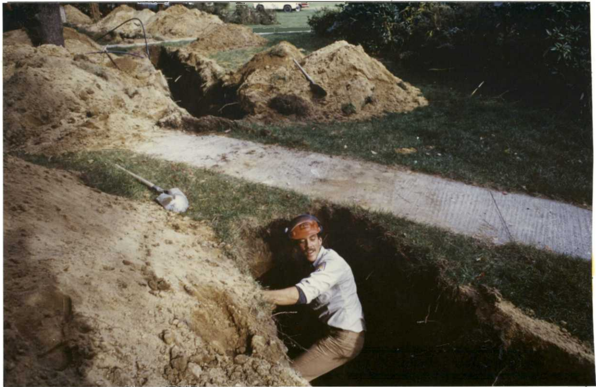
Maintenance Worker Bowden checking out trench for water line. J Hollingsworth - 1993.
