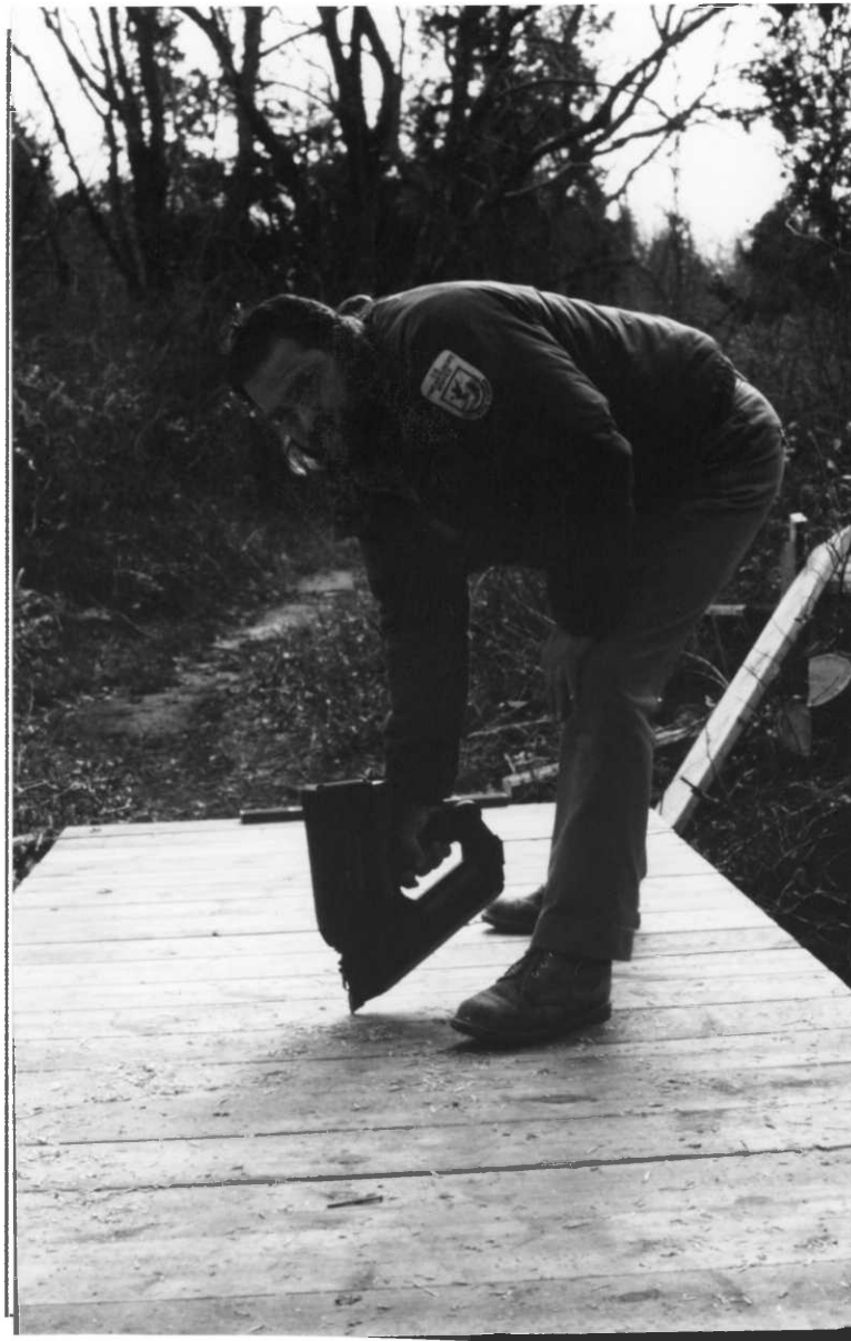
Laborer Woerner employing new nail gun on nature trail bridge. RWP - 93
