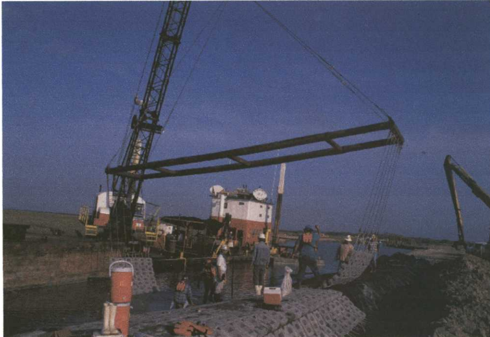
FWS channel being lined with reticulated concrete matting. FGP 6/00
