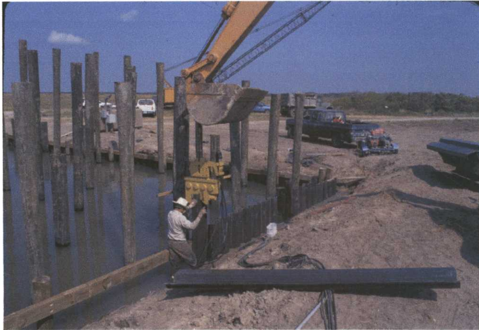
Frank and Will (on excavator) using vibro-hammer to install sheet-piling. FGP Summer/00
