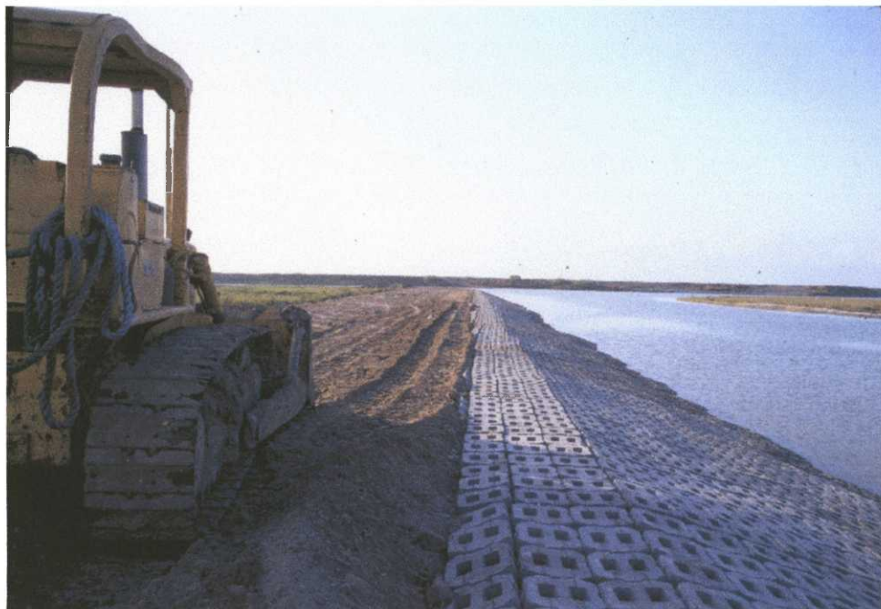
FES channel half completed with concrete matting. FGP 6/00
