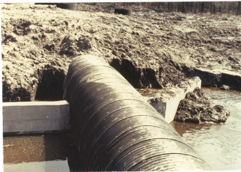
Severe erosion resulting from improperly installed pipes and water control structures on the Cayuga Lake Connector Project - a recurring nightmare throughout 1992. (92-22; TAG)
