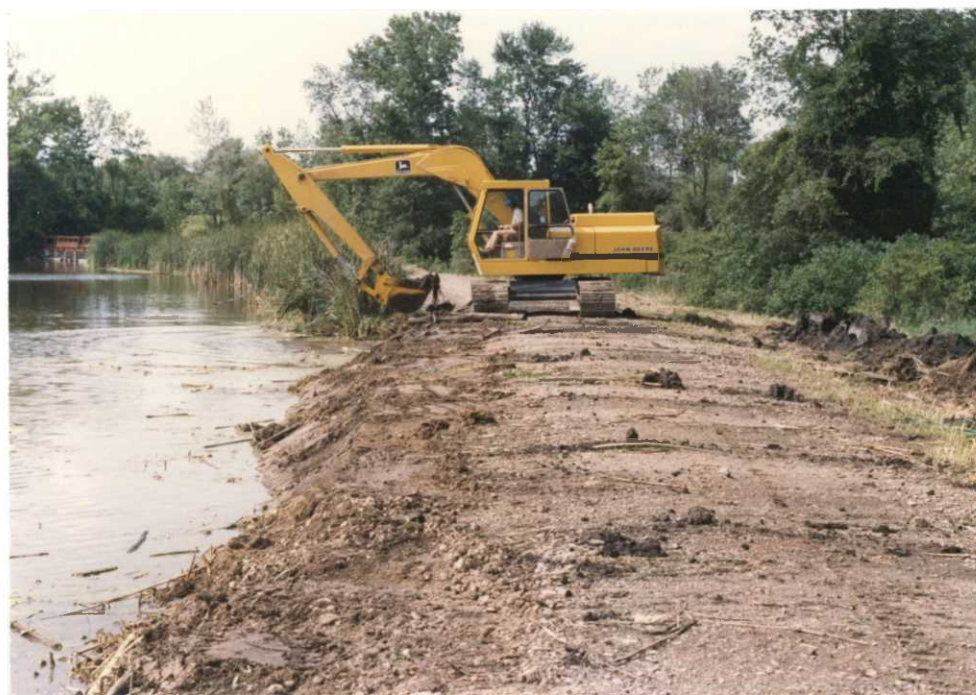
Initial stage of Tschache Pool Dike Repair Project. That's Maintenance Mechanic Steve Flanders operating Montezuma's 690C Hydraulic Excavator. (92-26; TAG)
