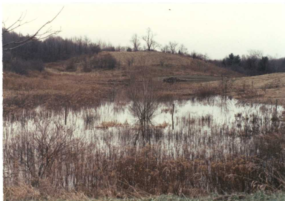
Hadden Restoration Site eight weeks after construction of a low-head dike. The site is completely full, and water is flowing over the spillway. (93-9; ID)
