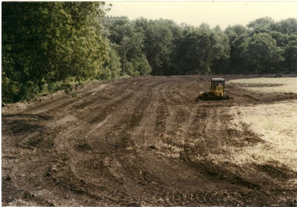
Maintenance Mechanic Flanders restoring the old dike. The pool interior will be managed as a moist soil impoundment primarily for shorebirds. (95-23; TAG)
