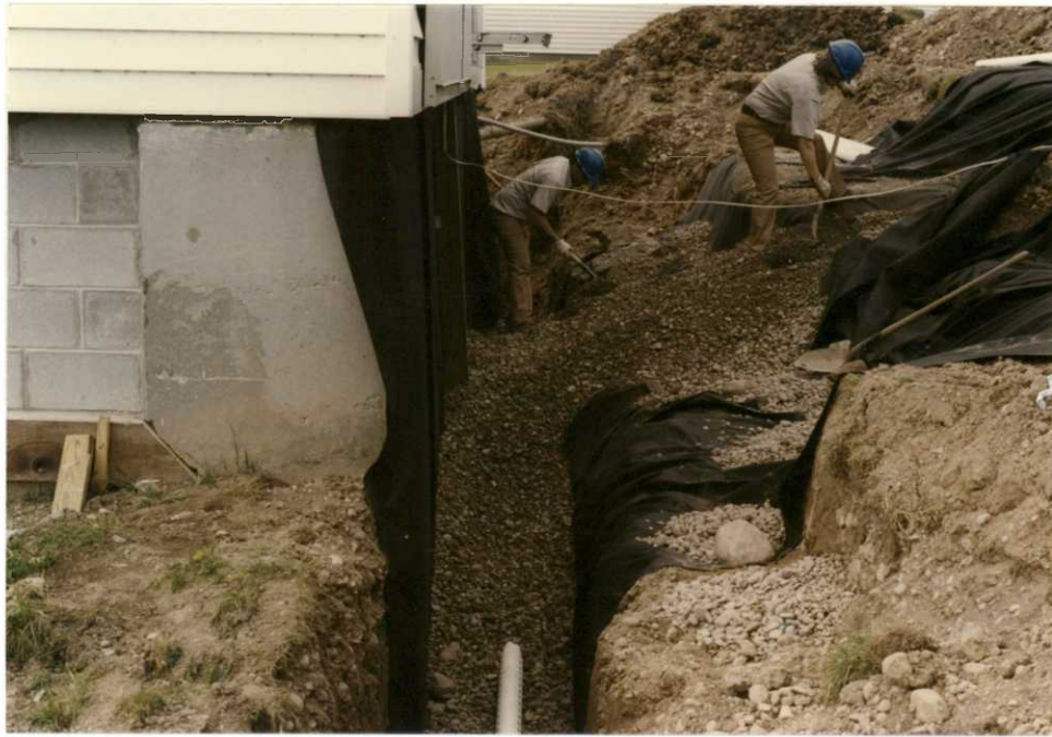
Flanders and Dates improving drainage around the barn. Also note Norsen has blocked up window. (95-25; REL)
