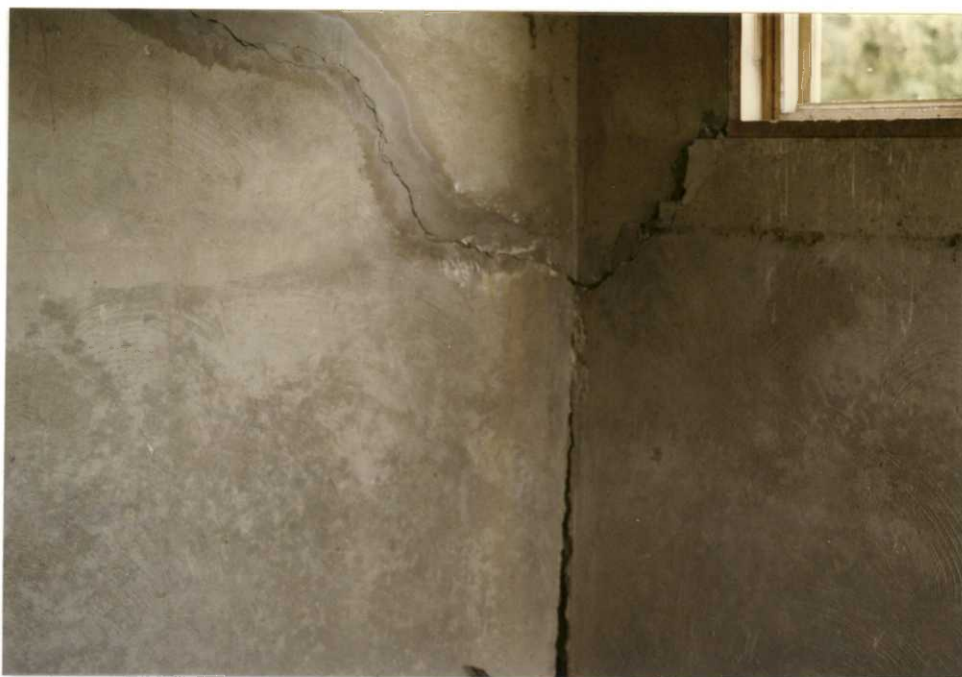
Years of poor drainage around the barn resulted in the foundation shifting badly. (95-24; MJN)
