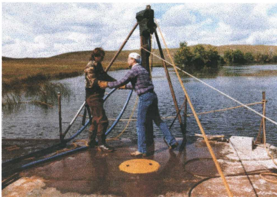
Figure 12. French and Stopak jetting pilings on the new fishing float. 96CRL12-LKM
