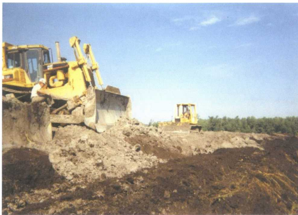
"Dirt Crew" profiling borrowed fill to contour dike core. (99-21; SLF)
