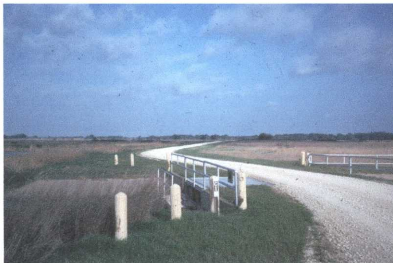
Figure 50. The resulting road surface provides all weather access for visitors to the Refuge, and does not require constant grading, as did the previous surface.
