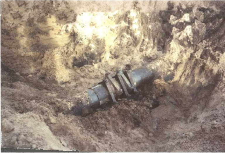
Figure 54. The pipeline company repaired the leak, and cleaned up the site. The Refuge fire crew burned the area to remove any remaining oil misted vegetation.
