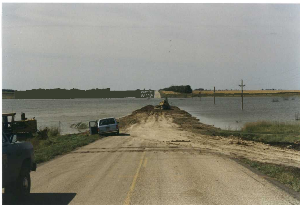
Highway 10 was overtopped in 1993. Repairs were initiated in 1994. A four foot grade raise made the road barely usable. HJH
