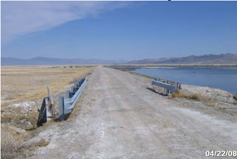
Photo # 3870 - MP 1.59 - Bridge
