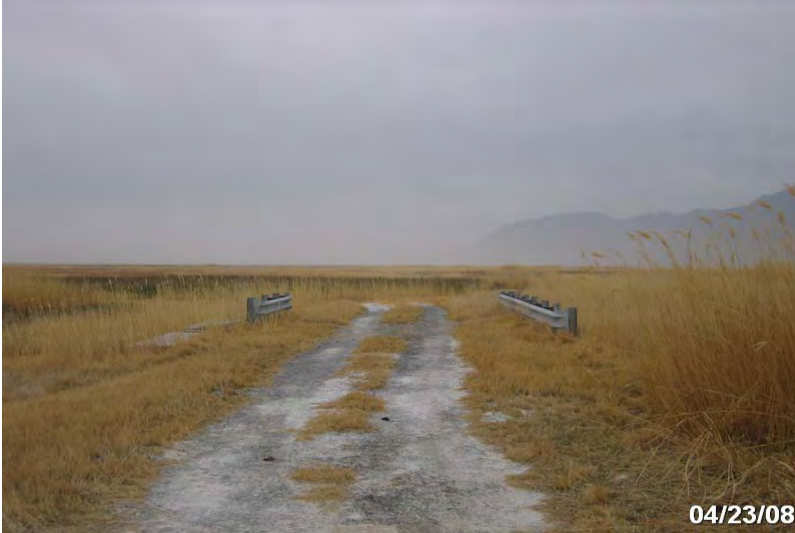
Photo # 3988 - MP 0.03 - Bridge
