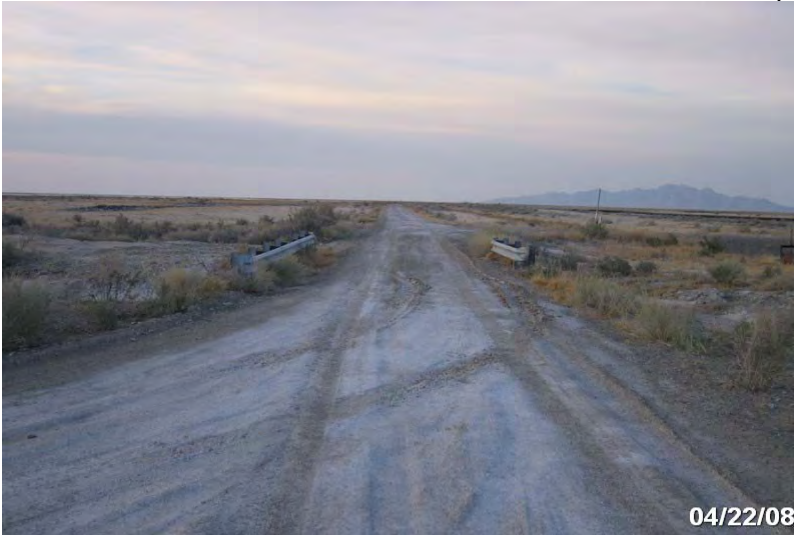
Photo # 3953 - MP 1.00 - Begin Section 002
