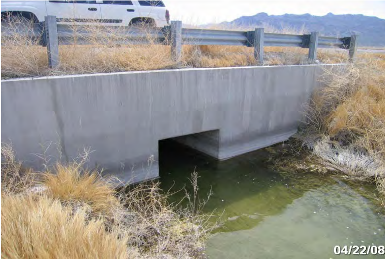
Photo # 3860 - MP 0.32 - Bridge
