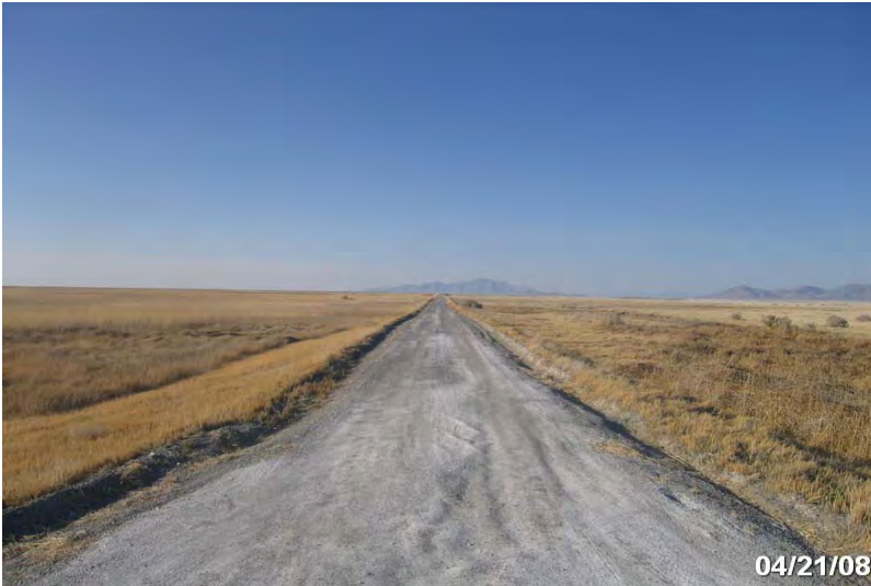
Photo # 3748 - MP 3.37 - Begin Section 005
