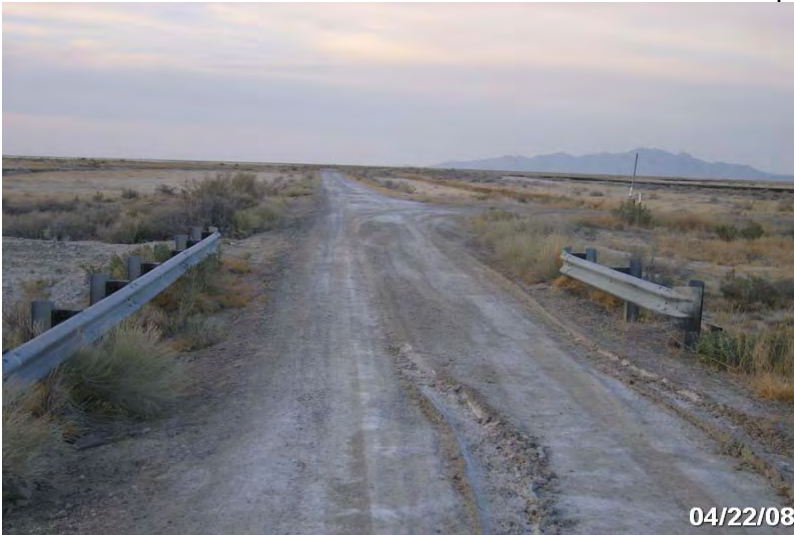
Photo # 3956 - MP 1.01 - Bridge
