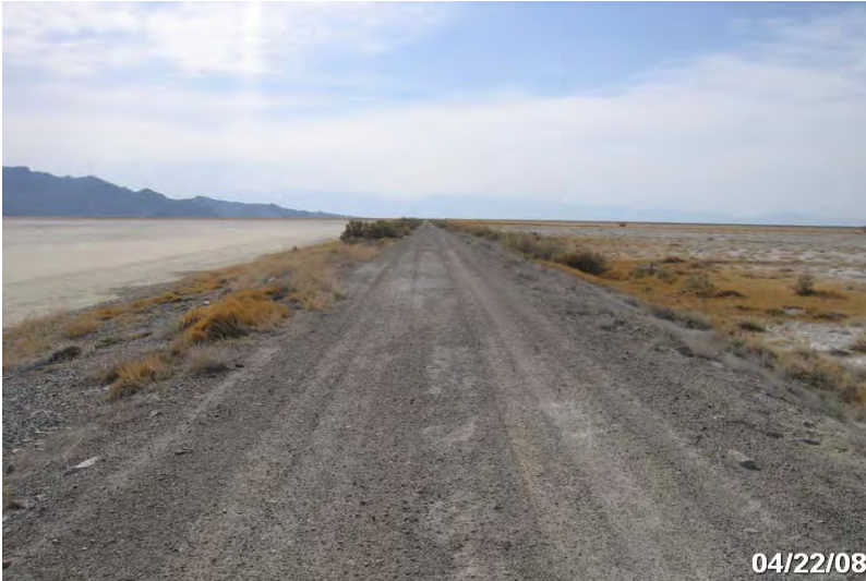
Photo # 3897 - MP 2.00 - Begin Section 003
