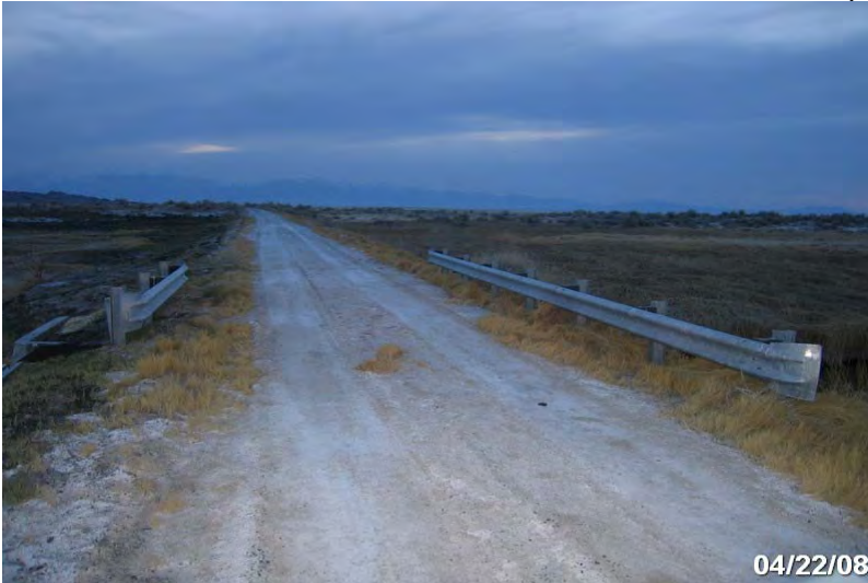
Photo # 3968 - MP 4.20 - Bridge
