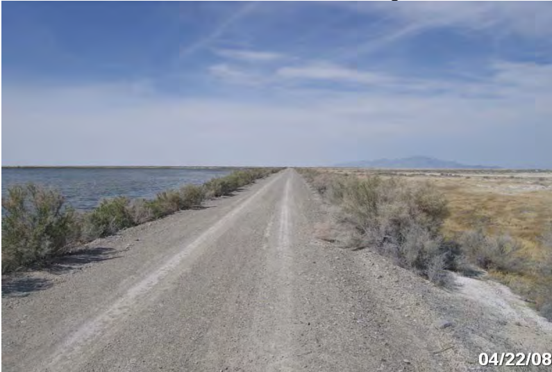
Photo # 3873 - MP 1.02 - Begin Section 002
