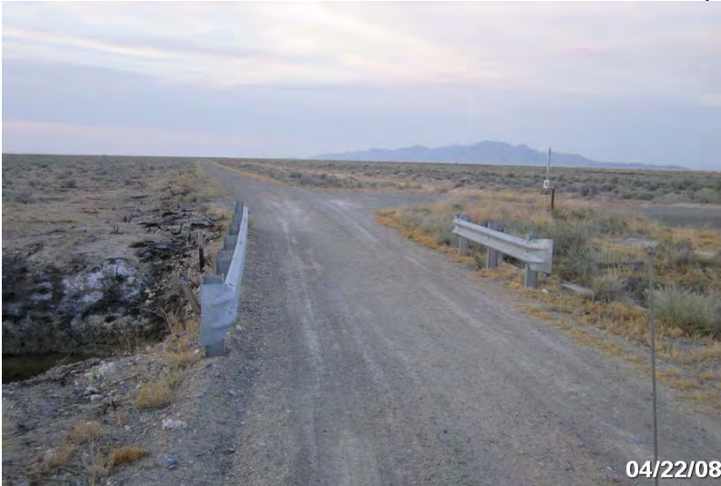
Photo # 3960 - MP 2.21 - Bridge
