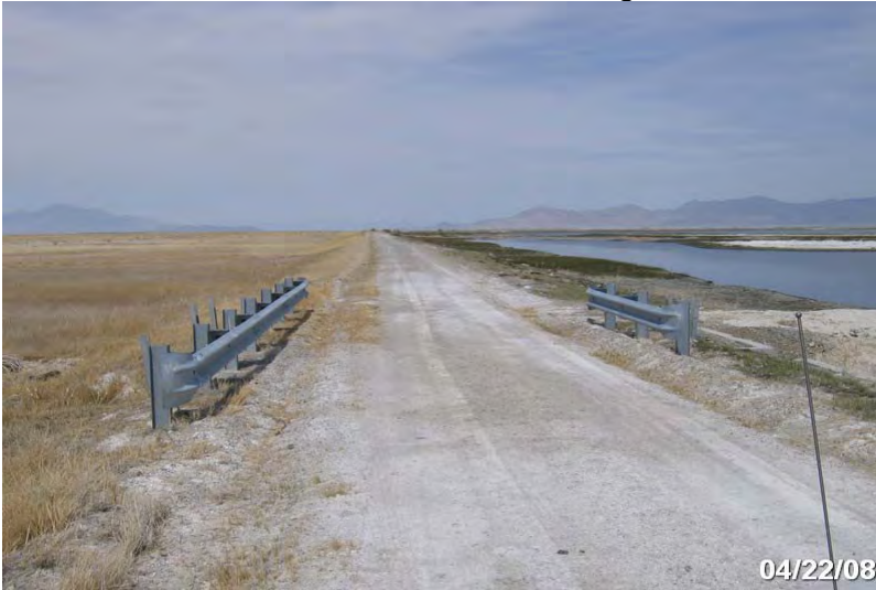
Photo # 3866 - MP 2.12 - Bridge
