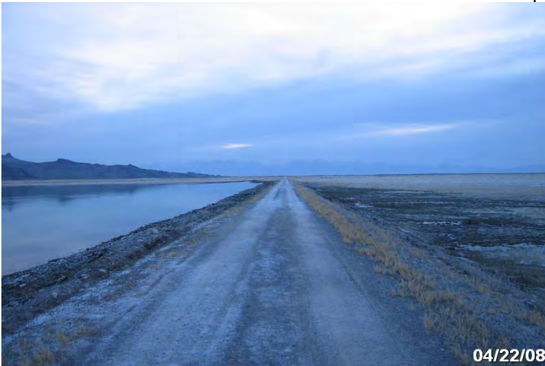
Photo # 3967 - MP 3.59 - Begin Section 005
