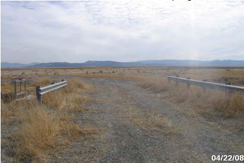
Photo # 3796 - MP 0.01 - Bridge
