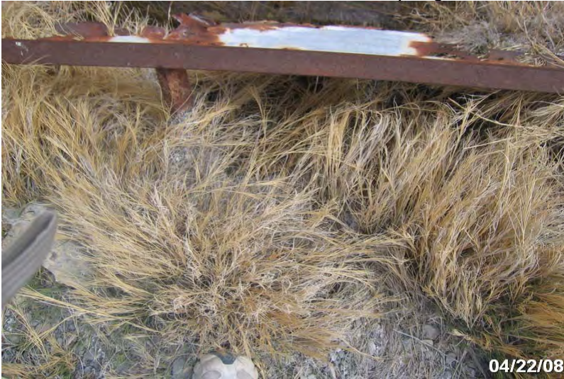
Photo # 3806 - MP 0.62 - Culvert Deficiency
