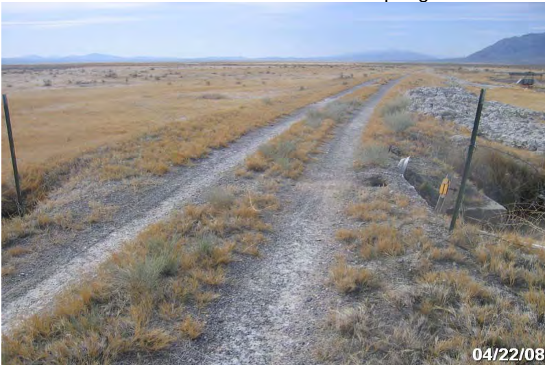
Photo # 3799 - MP 0.05 - Bridge
