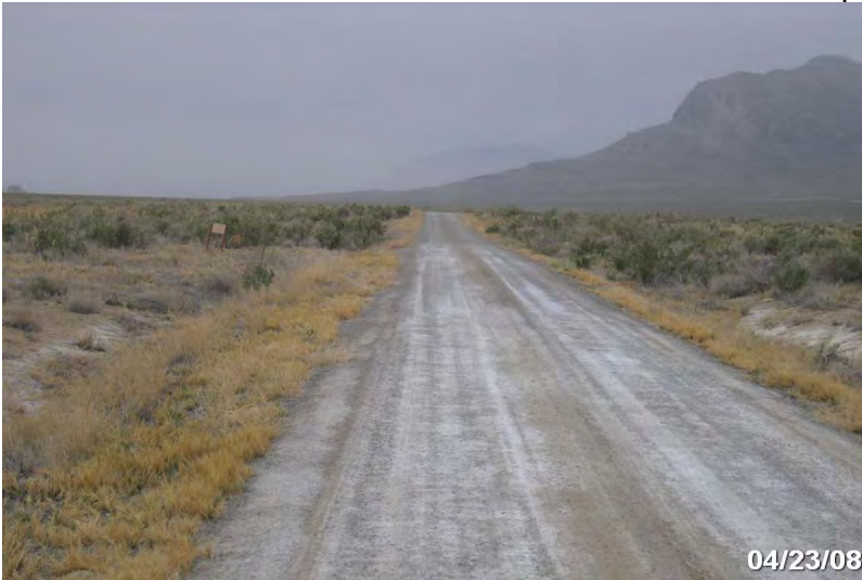
Photo # 3979 - MP 7.33 - Begin Section 009
