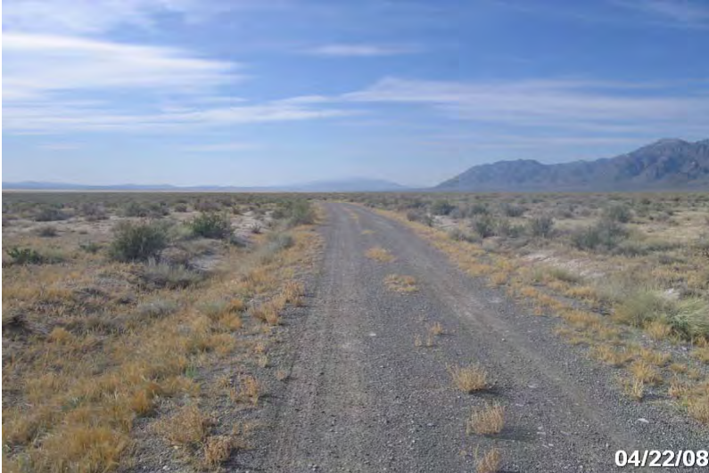
Photo # 3792 - MP 1.00 - Begin Section 002
