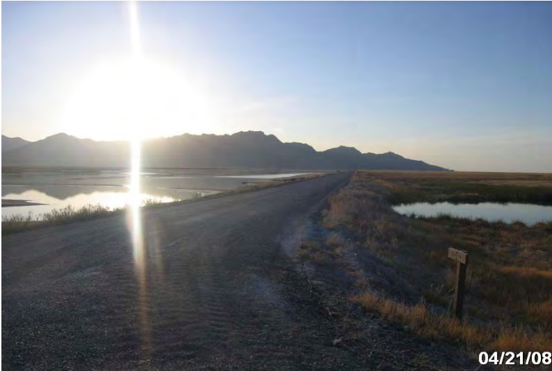
Photo # 3771 - MP 6.83 - Begin Section 009
