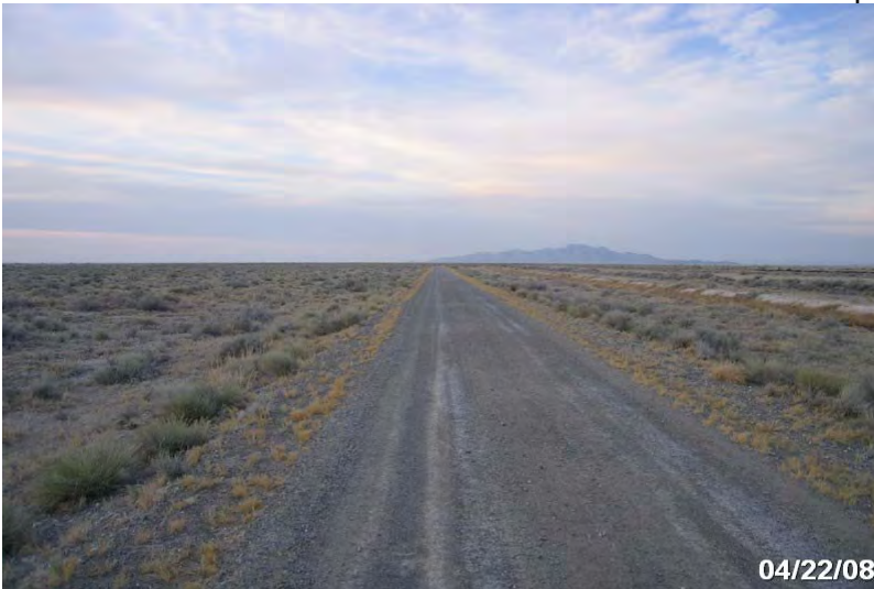
Photo # 3959 - MP 2.01 - Begin Section 003
