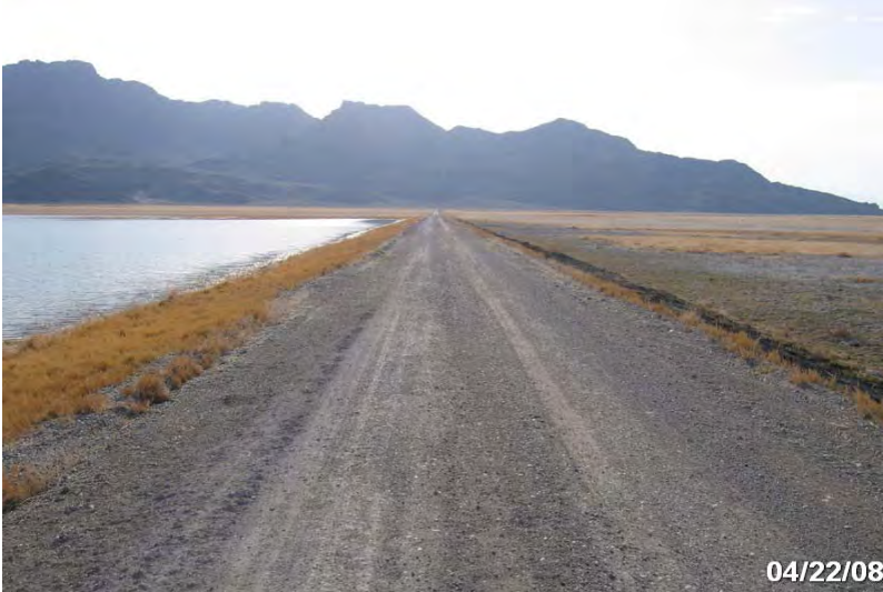
Photo # 3923 - MP 1.00 - Begin Section 002
