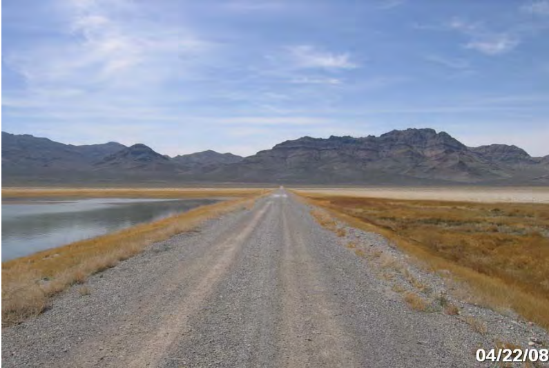
Photo # 3857 - MP 1.00 - Begin Section 002
