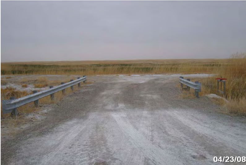
Photo # 3985 - MP 0.01 - Bridge
