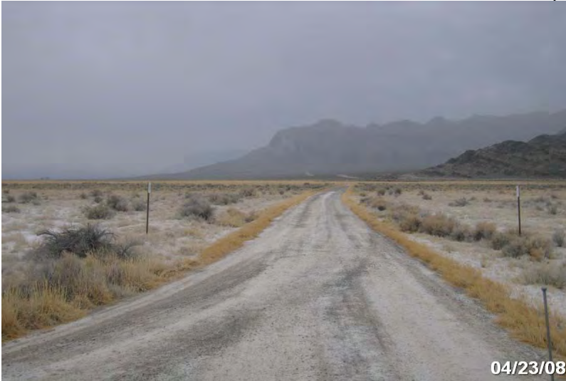
Photo # 3978 - MP 6.32 - Begin Section 008
