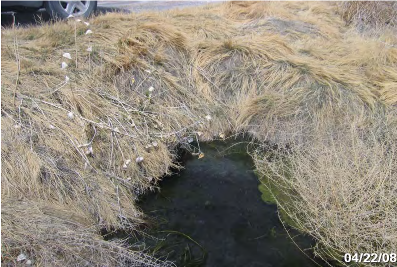
Photo # 3847 - MP 0.12 - Bridge
