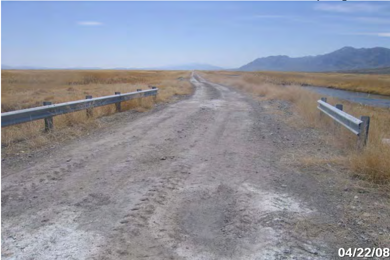
Photo # 3843 - MP 0.01 - Bridge
