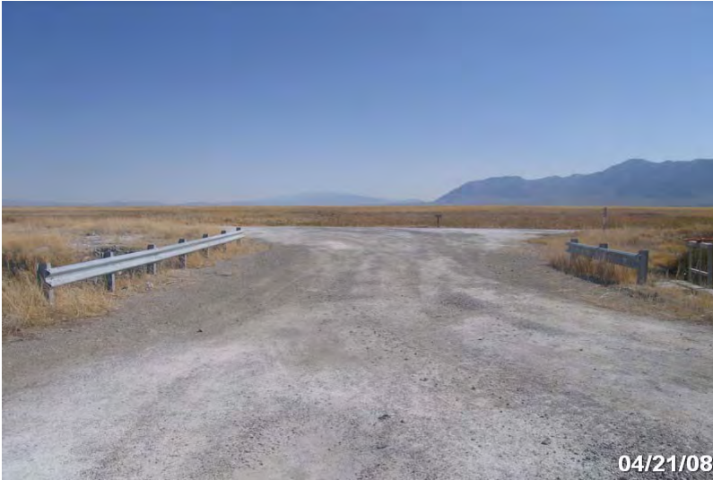
Photo # 3734 - MP 1.99 - Begin Section 004
