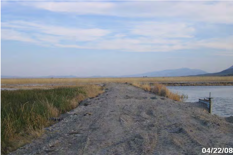
Photo # 3942 - MP 0.59 - Begin Section 002
