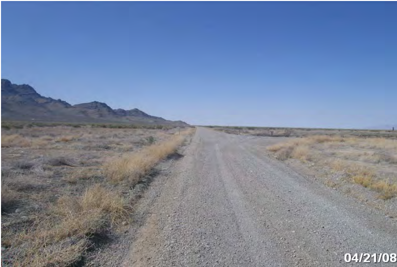
Photo # 3722 - MP 0.81 - Begin Section 002
