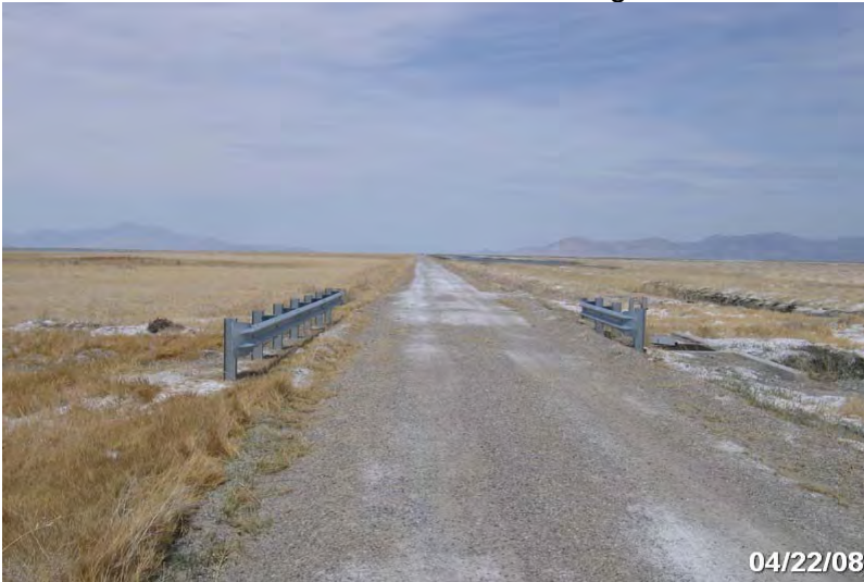
Photo # 3863 - MP 2.88 - Bridge
