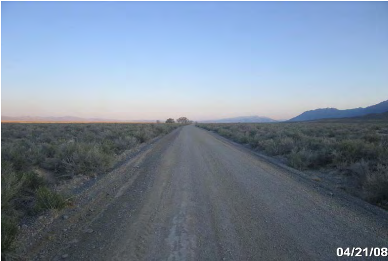
Photo # 3779 - MP 8.66 - Begin Section 011
