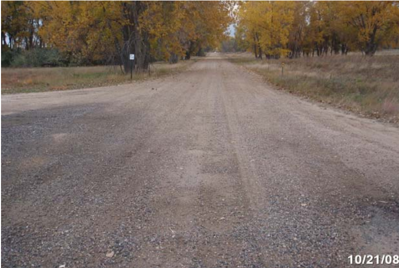
Photo # 1908 - MP 2.01 - Begin Section 003
