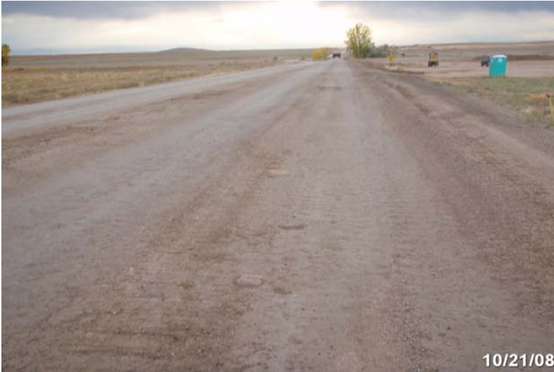
Photo # 1925 - MP 3.75 - Begin Section 008
