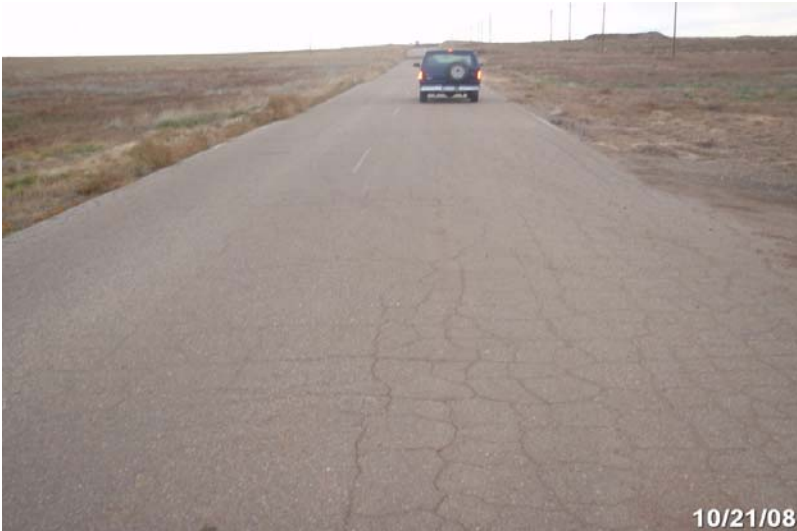
Photo # 1921 - MP 2.42 - Begin Section 004
