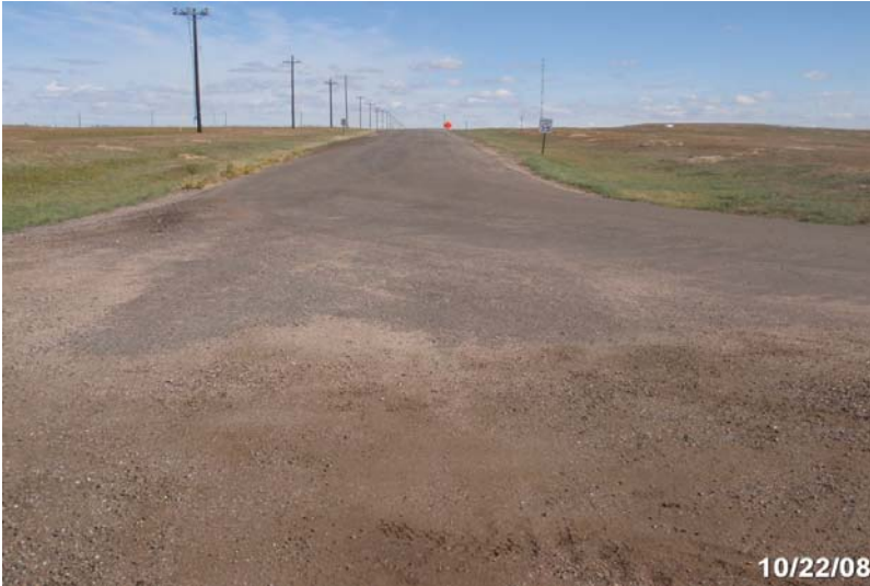
Photo # 2020 - MP 0.80 - Begin Section 002
