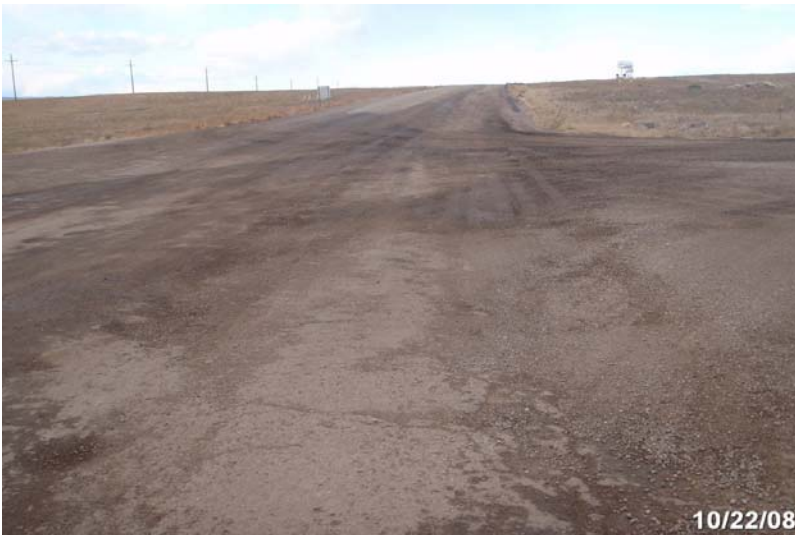
Photo # 2045 - MP 0.98 - Begin Section 002
