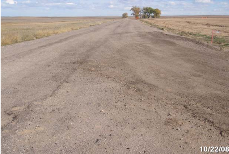
Photo # 2025 - MP 2.16 - Begin Section 005
