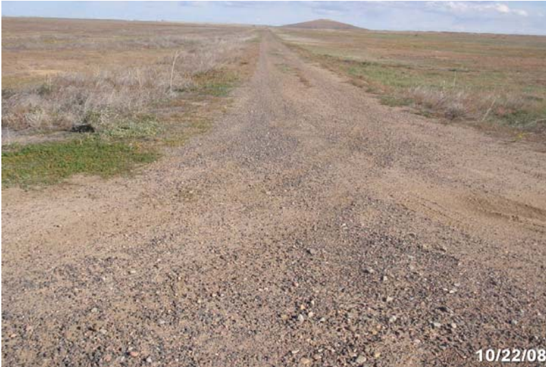
Photo # 2028 - MP 3.77 - Begin Section 008
