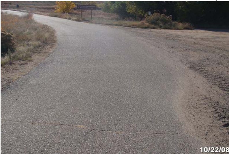
Photo # 1974 - MP 0.26 - Begin Section 003
