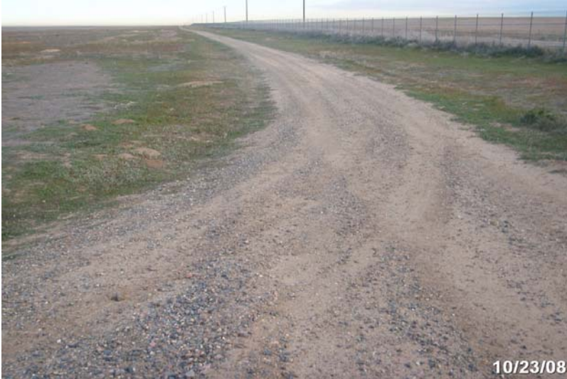
Photo # 2069 - MP 1.94 - Begin Section 003
