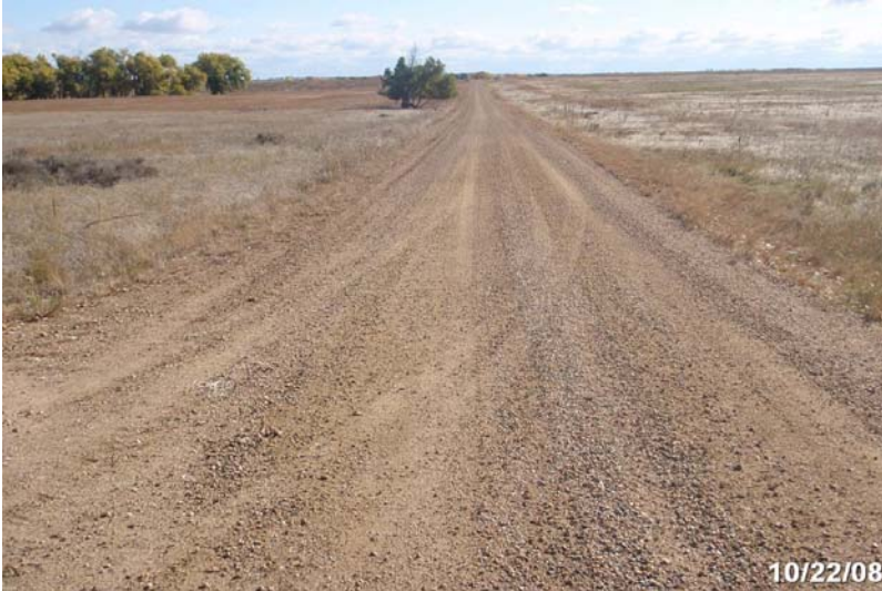
Photo # 1982 - MP 3.01 - Begin Section 004
