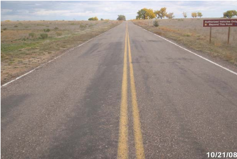
Photo # 1904 - MP 0.98 - Begin Section 002
