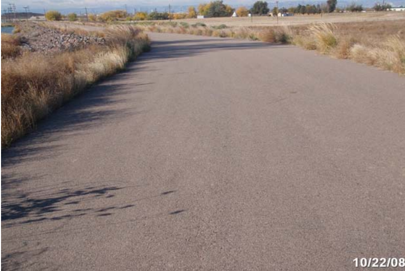
Photo # 1968 - MP 1.16 - Begin Section 002
