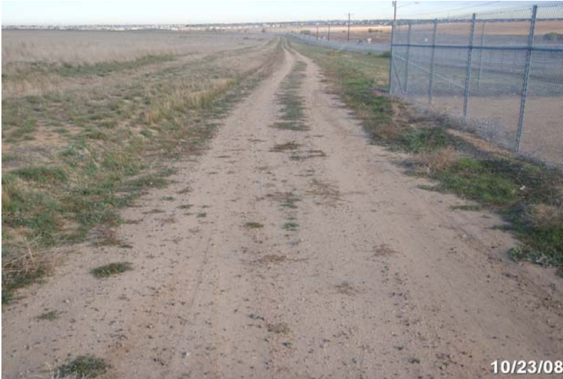
Photo # 2071 - MP 3.95 - Begin Section 005
