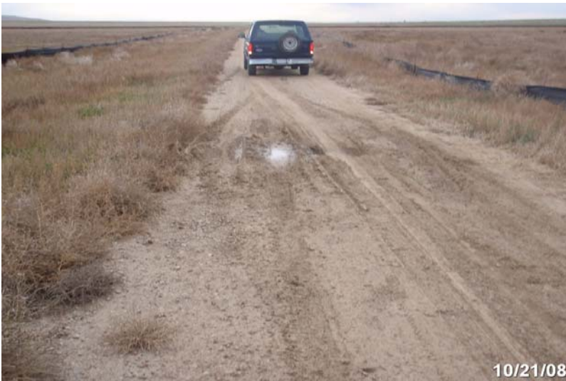
Photo # 1927 - MP 4.61 - Begin Section 007
