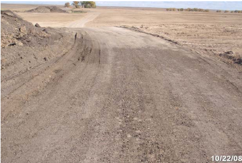
Photo # 2024 - MP 2.06 - Begin Section 004
