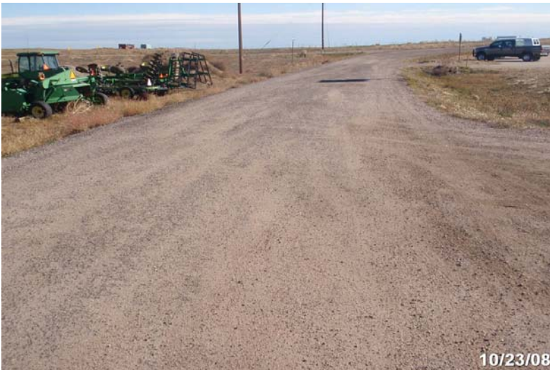
Photo # 2101 - MP 0.18 - Begin Section 002
