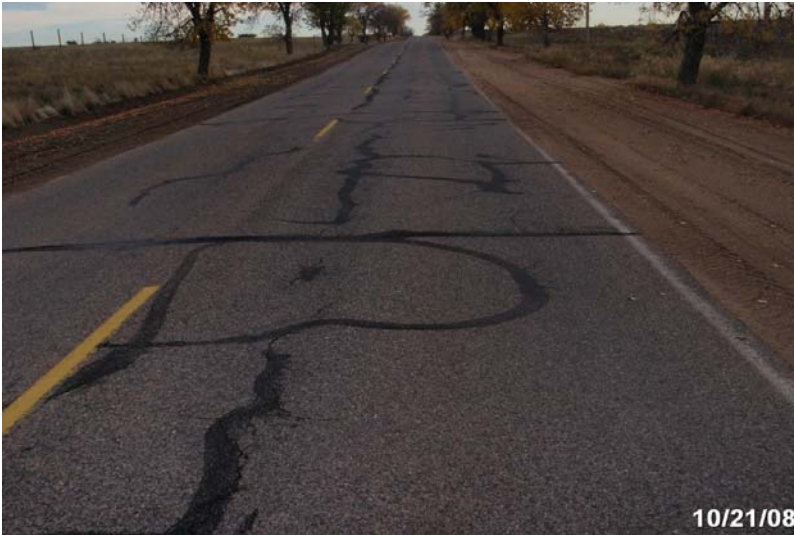
Photo # 1869 - MP 0.99 - Begin Section 002
