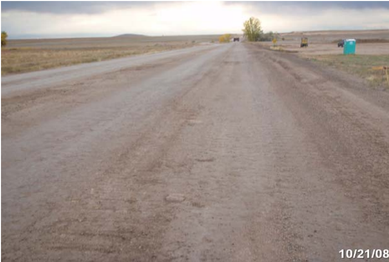
Photo # 1925 - MP 3.63 - Begin Section 006
