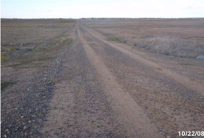
Photo # 2041 - MP 2.00 - Begin Section 004
