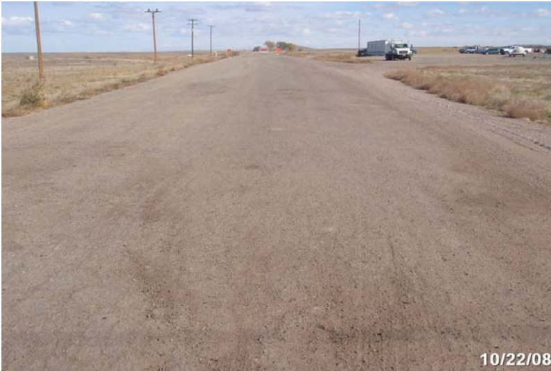
Photo # 2023 - MP 1.80 - Begin Section 003
