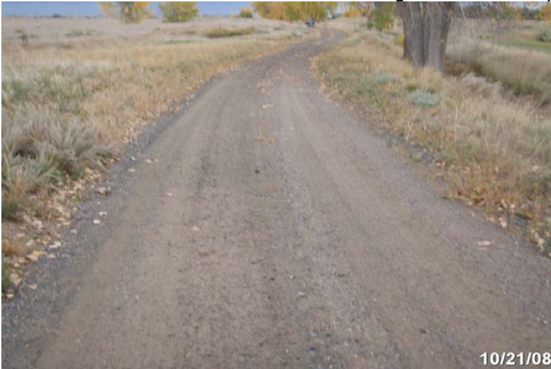
Photo # 1950 - MP 1.03 - Begin Section 002
