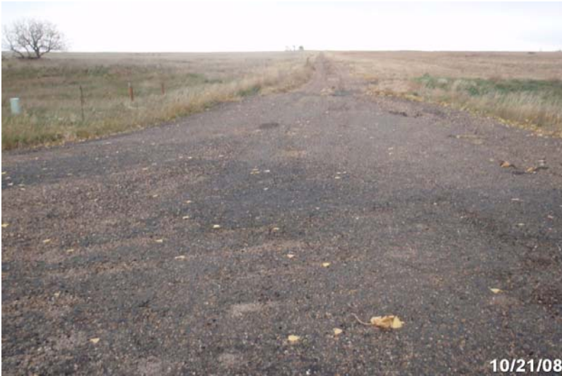
Photo # 1936 - MP 0.99 - Begin Section 002
