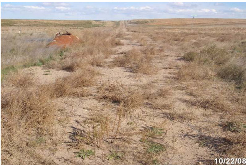
Photo # 2027 - MP 2.78 - Begin Section 007
