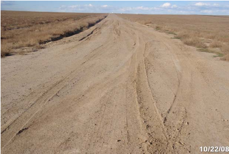
Photo # 2036 - MP 1.00 - Begin Section 002
