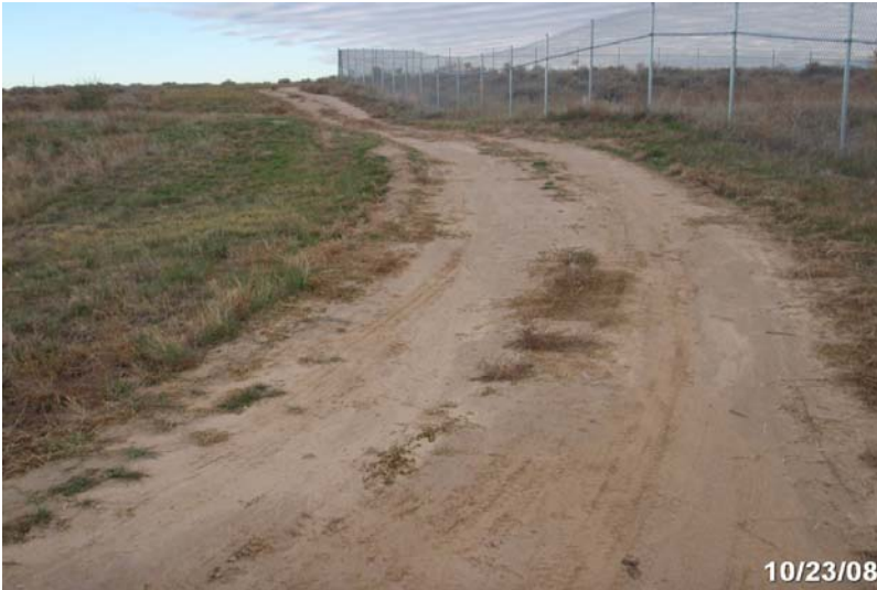
Photo # 2061 - MP 3.27 - Begin Section 004
