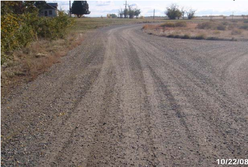
Photo # 1971 - MP 0.11 - Begin Section 002
