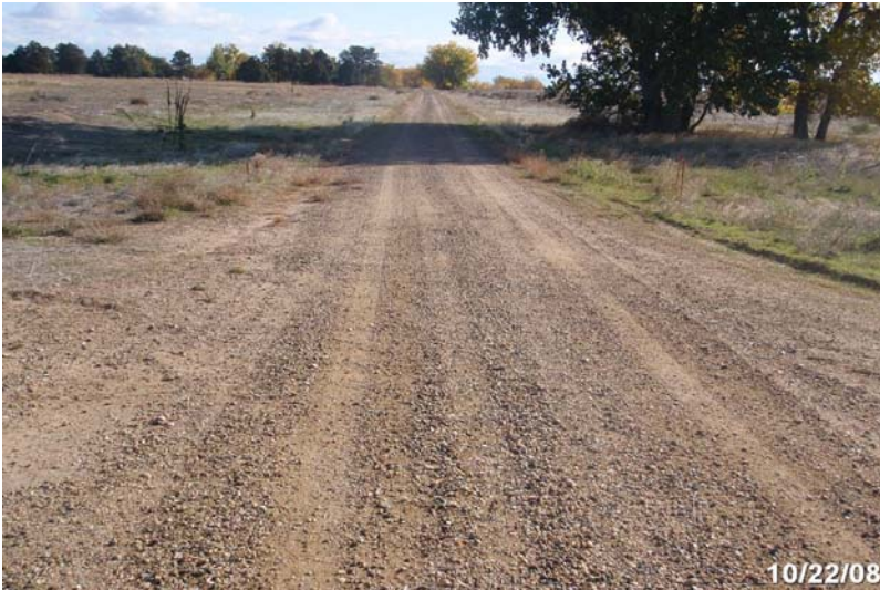
Photo # 1985 - MP 3.99 - Begin Section 005
