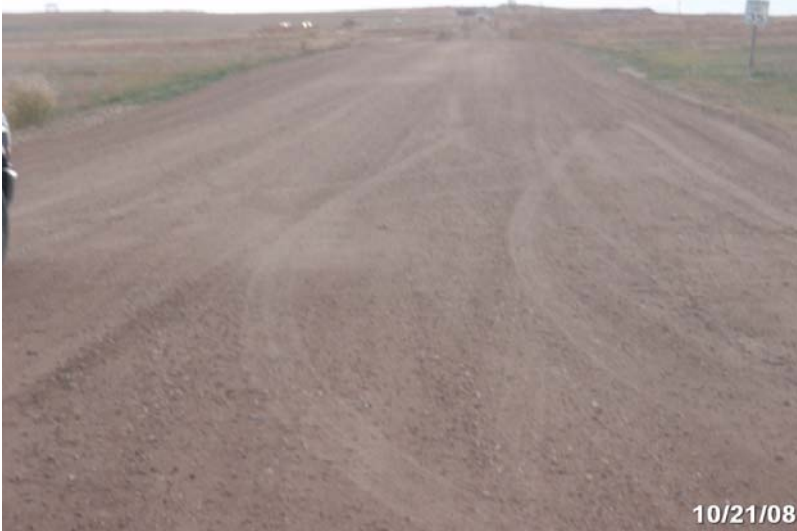
Photo # 1918 - MP 1.63 - Begin Section 003
