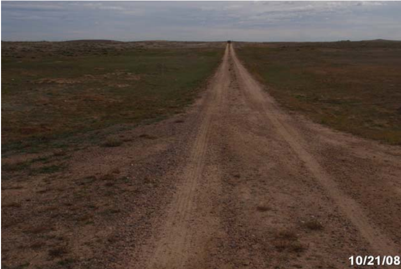
Photo # 1892 - MP 0.62 - Begin Section 002
