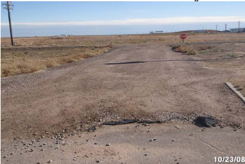
Photo # 2096 - MP 0.06 - Begin Section 002
