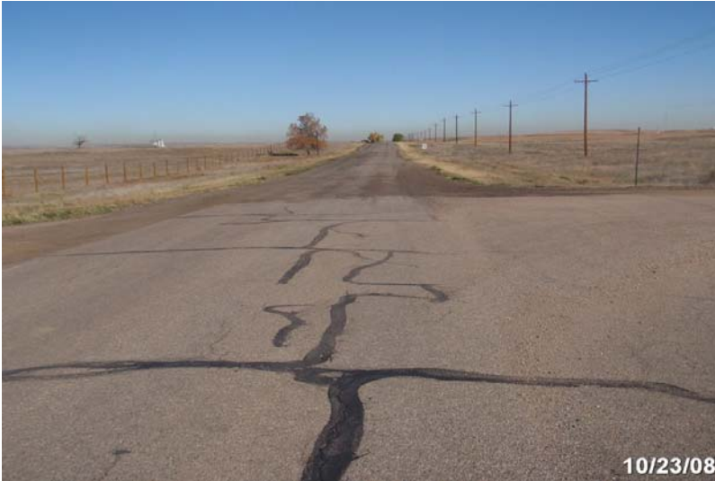
Photo # 2082 - MP 1.00 - Begin Section 002
