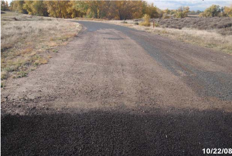
Photo # 1959 - MP 0.54 - Begin Section 002
