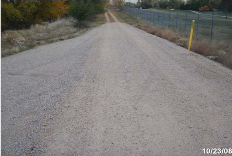
Photo # 2059 - MP 2.25 - Begin Section 003
