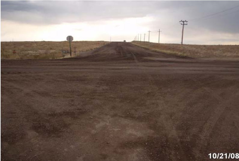
Photo # 1922 - MP 2.62 - Begin Section 005
