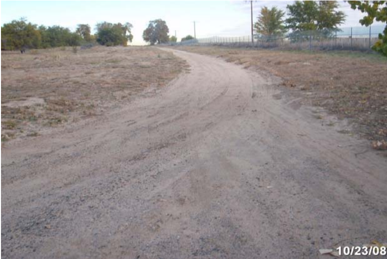
Photo # 2066 - MP 0.94 - Begin Section 002
