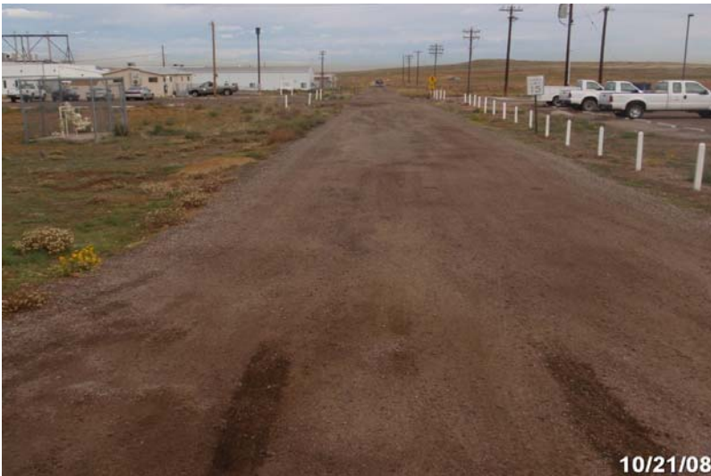
Photo # 1872 - MP 0.50 - Begin Section 002
