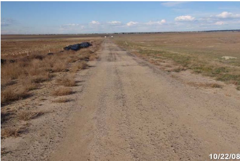
Photo # 2037 - MP 1.62 - Begin Section 003
