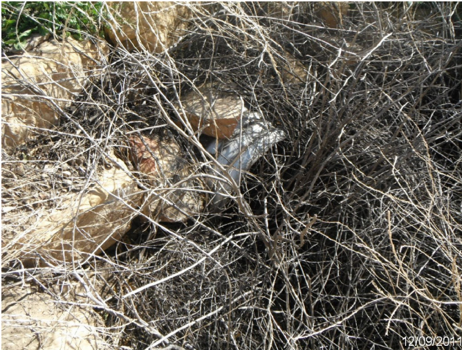
Photo: HOMO_C4_0146 Route: 300-002-1.03 Metal Culvert 35ft long 24in dia. 3ft deep Asset# 10001464
