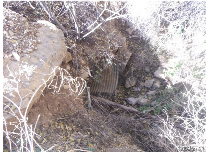
Photo: HOMO_C4_0135 Route: 400-001-0.57 Metal Culvert 30ft long 48in dia. 3ft deep Asset# NA
