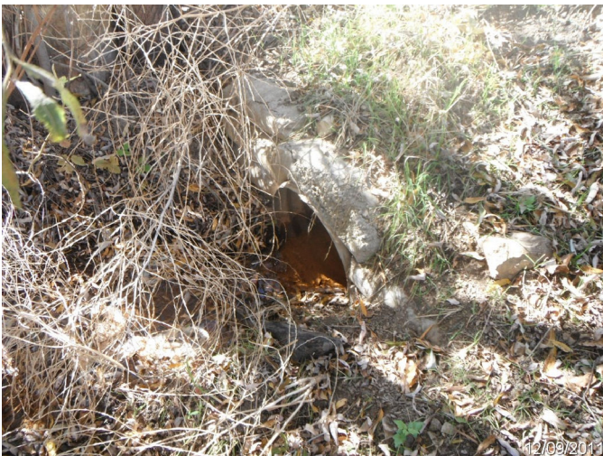
Photo: HOMO_C4_0150 Route: 300-003-2.7 Metal Culvert 25ft long 18in dia. 1ft deep Asset# 10001464
