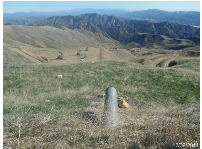
Photo: HOMO_C4_0160 Route: 402-001-0.14 Metal Culvert 20ft long 18in dia. 1ft deep Asset# NA
