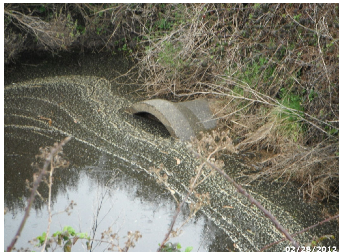
Photo: HUBA_C4_1685 Route: 400-004-2.58 Concrete Culvert 30ft long 48in dia. 4ft deep Asset# 10000105
