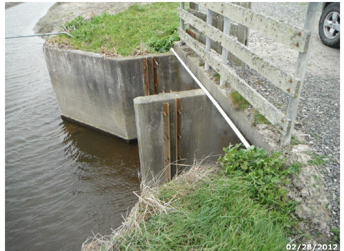
Photo: HUBA_C4_1701 Route: 401-001-0.3 Concrete WCS Flashboard Riser 20ft long 1ft deep 5x10 Box Culvert Asset# 10036313
