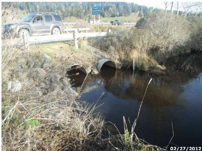
Photo: HUBA_C4_1594 Route: 010-002-1.08 Metal WCS Flashboard Riser 40ft long 48in dia. 3ft deep Asset# NA
