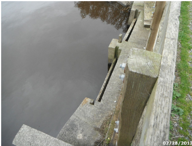
Photo: HUBA_C4_1678 Route: 400-001-0.52 Concrete WCS Flashboard Riser 15ft long 1ft deep 4x4 Box Culvert Asset# 10036311
