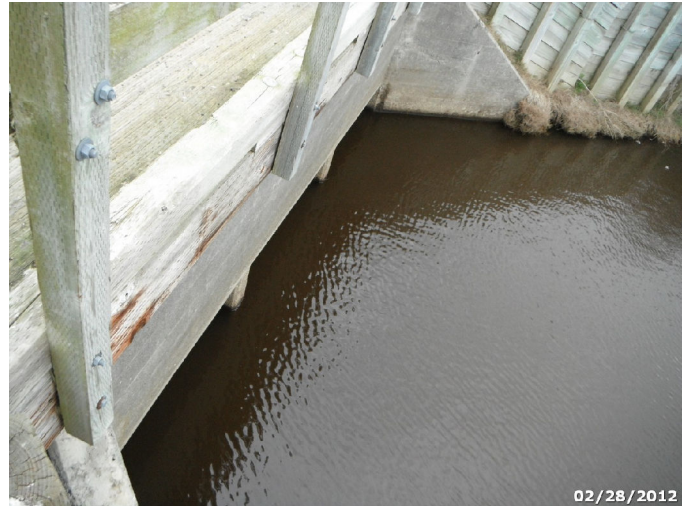
Photo: HUBA_C4_1707 Route: 403-001-0.1 Concrete WCS Flashboard Riser 12ft long 1ft deep 5x10 Box Culvert Asset# 10036310
