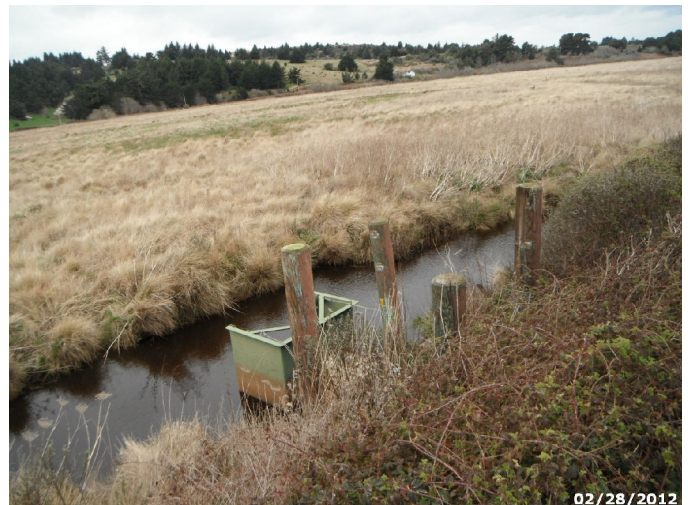
Photo: HUBA_C4_1722 Route: 402-002-1.46 Metal WCS Flap Gate/Full-Round Riser 60ft long 48in dia. 10ft deep Asset# NA 8-013
