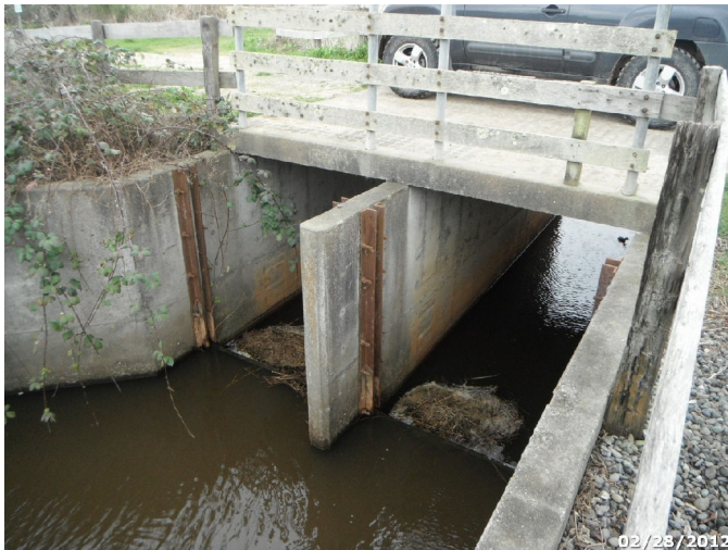
Photo: HUBA_C4_1695 Route: 401-002-0.7 Concrete WCS Flashboard Riser 20ft long 1ft deep 5x10 Box Culvert Asset# 10036309
