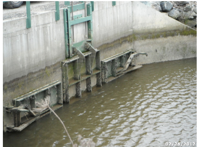
Photo: HUBA_C4_1713 Route: 403-002-1.13 Concrete WCS Other 25ft long 1ft deep 5x12 Box Culvert Asset# 10061429
