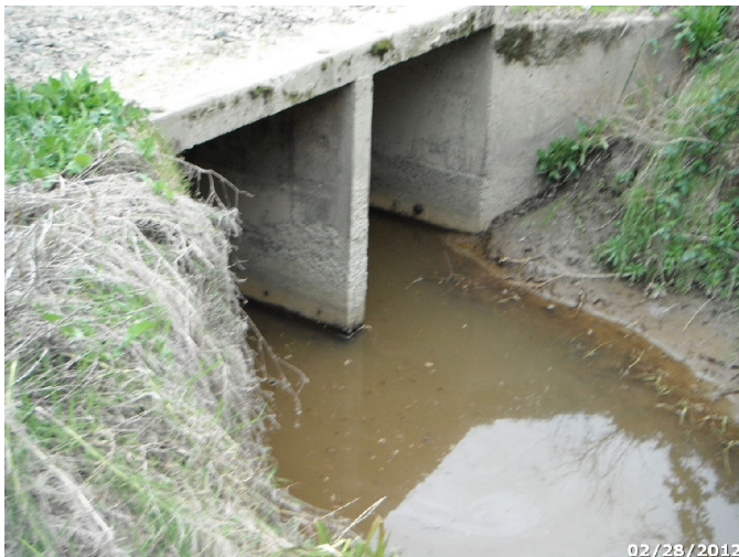
Photo: HUBA_C4_1716 Route: 403-003-1.96 Concrete WCS Flashboard Riser 20ft long 1ft deep 6x10 Box Culvert Asset# 10036312
