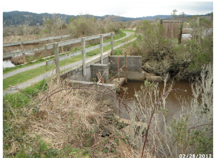
Photo: HUBA_C4_1677 Route: 400-001-0.52 Concrete WCS Flashboard Riser 15ft long 1ft deep 4x4 Box Culvert Asset# 10036311 8-007
