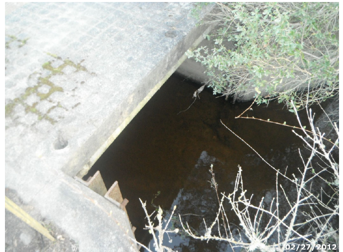
Photo: HUBA_C4_1592 Route: 010-002-0.63 Concrete Culvert Box 24ft long 6ft x 10ft 1ft deep Asset# NA
