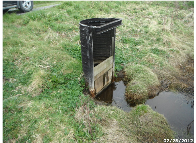
Photo: HUBA_C4_1675 Route: 400-001-0.3 Metal WCS Flashboard Riser 50ft long 24in dia. 2ft deep Asset# NA
