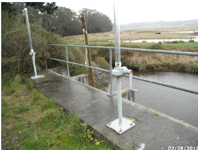
Photo: HUBA_C4_1683 Route: 400-003-2.6 Metal WCS Flashboard Riser 30ft long 1ft deep 6x10 Box Culvert Asset# NA
