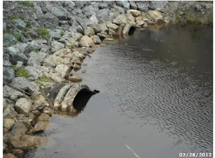
Photo: HUBA_C4_1673 Route: 400-001-0.05 Plastic Culvert 40ft long 48in dia. 2ft deep Asset# 10000105
