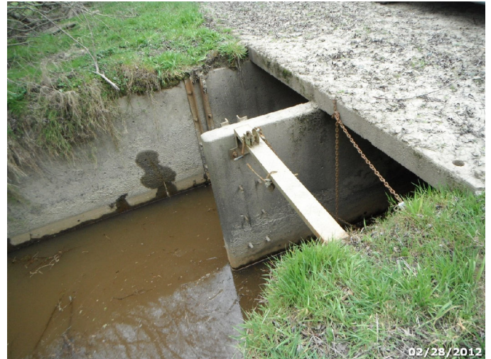
Photo: HUBA_C4_1715 Route: 403-003-1.96 Concrete WCS Flashboard Riser 20ft long 1ft deep 6x10 Box Culvert Asset# 10036312
