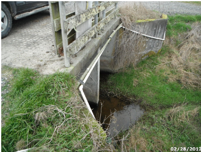
Photo: HUBA_C4_1700 Route: 401-001-0.3 Concrete WCS Flashboard Riser 20ft long 1ft deep 5x10 Box Culvert Asset# 10036315
