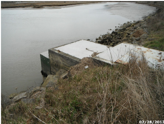
Photo: HUBA_C4_1719 Route: 402-001-0.55 Concrete WCS Other 25ft long 36in dia. 1ft deep Unknown type Asset# NA
