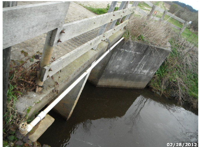
Photo: HUBA_C4_1696 Route: 401-002-0.7 Concrete WCS Flashboard Riser 20ft long 1ft deep 5x10 Box Culvert Asset# 10036309
