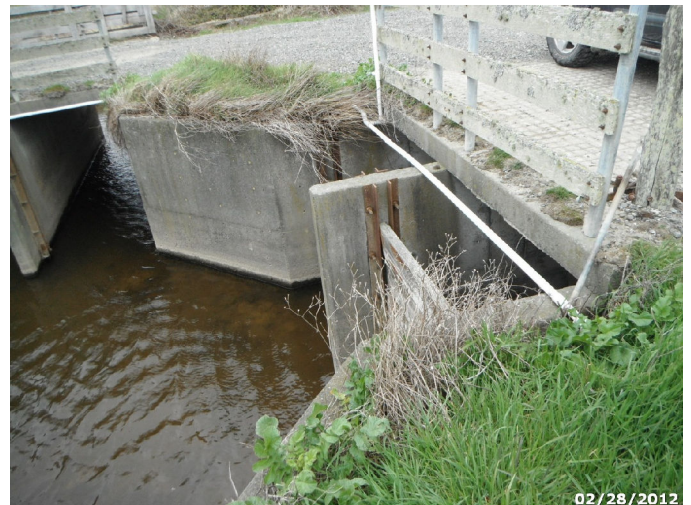
Photo: HUBA_C4_1699 Route: 401-001-0.3 Concrete WCS Flashboard Riser 20ft long 1ft deep 5x10 Box Culvert Asset# 10036315
