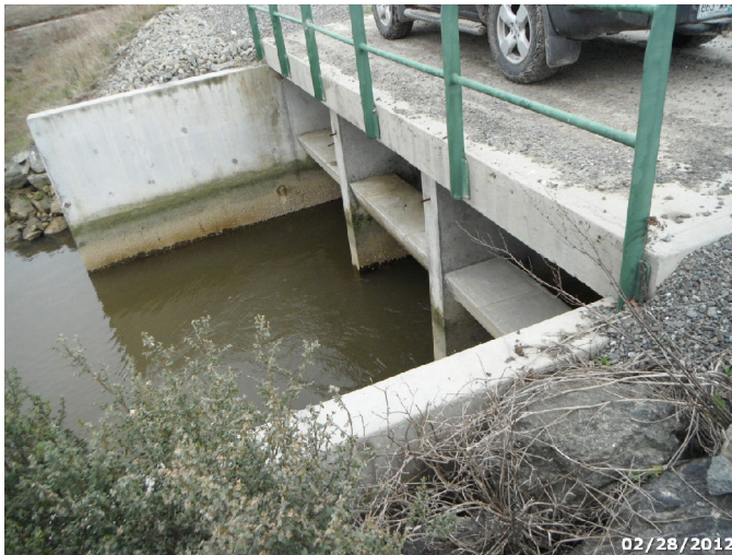
Photo: HUBA_C4_1712 Route: 403-002-1.13 Concrete WCS Other 25ft long 1ft deep 5x12 Box Culvert Asset# 10061429
