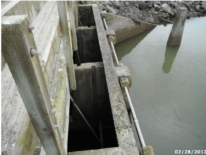
Photo: HUBA_C4_1708 Route: 403-001-0.1 Concrete WCS Flashboard Riser 12ft long 1ft deep 5x10 Box Culvert Asset# 10036310
