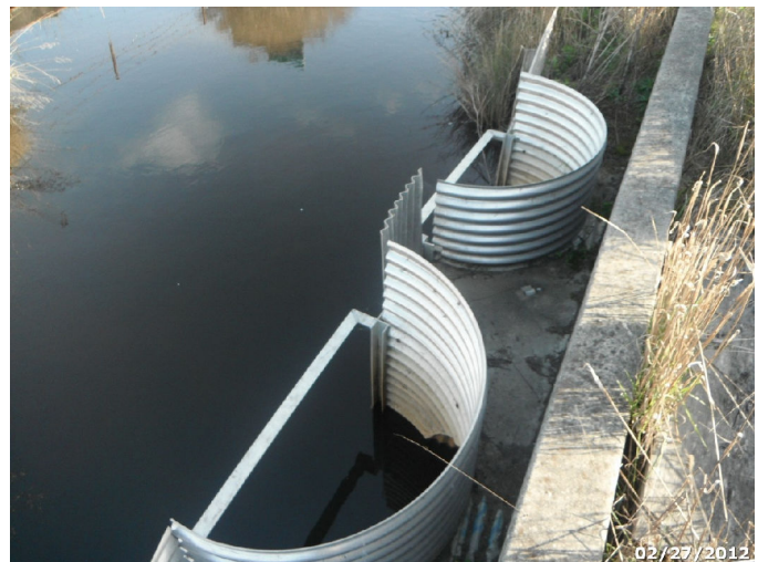
Photo: HUBA_C4_1595 Route: 010-002-1.08 Metal WCS Flashboard Riser 40ft long 48in dia. 3ft deep Asset# NA
