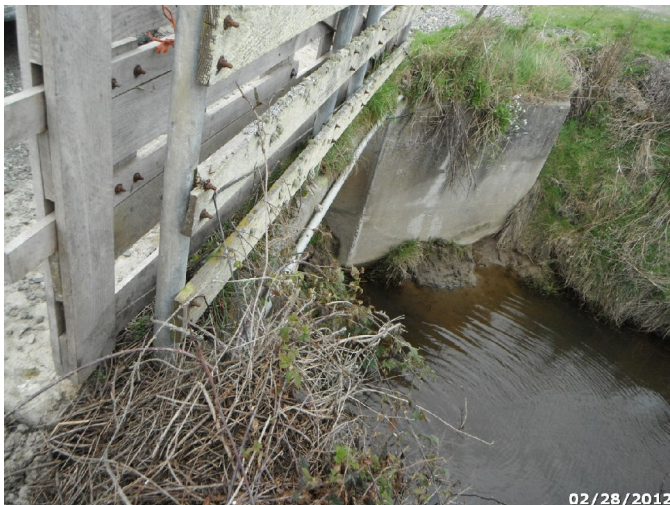
Photo: HUBA_C4_1702 Route: 401-001-0.3 Concrete WCS Flashboard Riser 20ft long 1ft deep 5x10 Box Culvert Asset# 10036313
