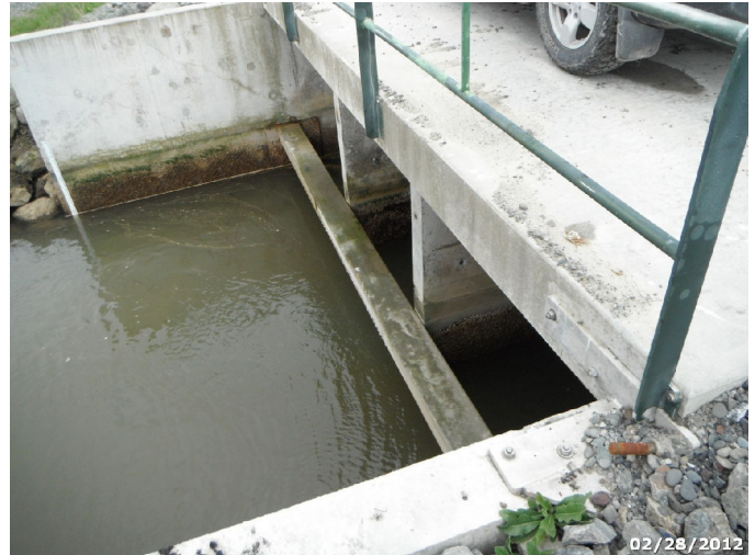
Photo: HUBA_C4_1709 Route: 403-001-0.4 Concrete WCS Other 12ft long 1ft deep 5x10 Box Culvert Asset# 10061428
