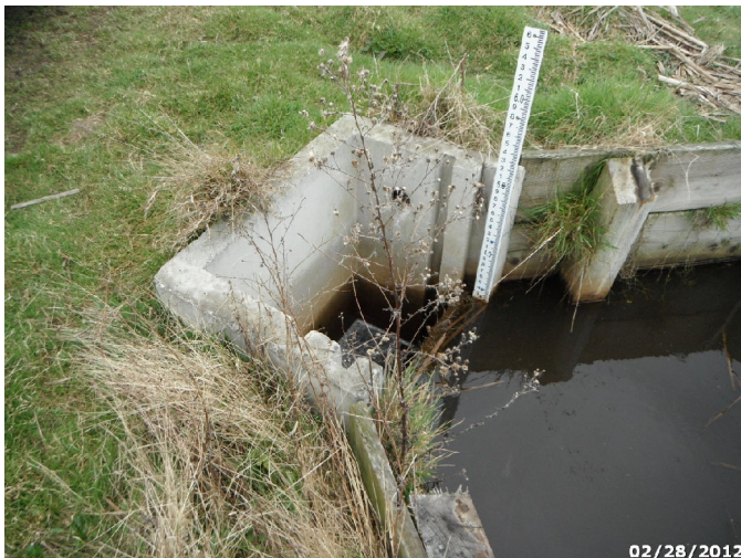
Photo: HUBA_C4_1689 Route: 400-004-3.13 Plastic WCS Flashboard Riser 40ft long 24in dia. 2ft deep Asset# NA
