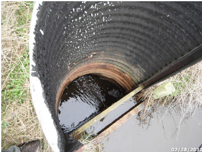
Photo: HUBA_C4_1687 Route: 400-004-3.02 Metal WCS Flashboard Riser 30ft long 24in dia. 1ft deep Asset# NA
