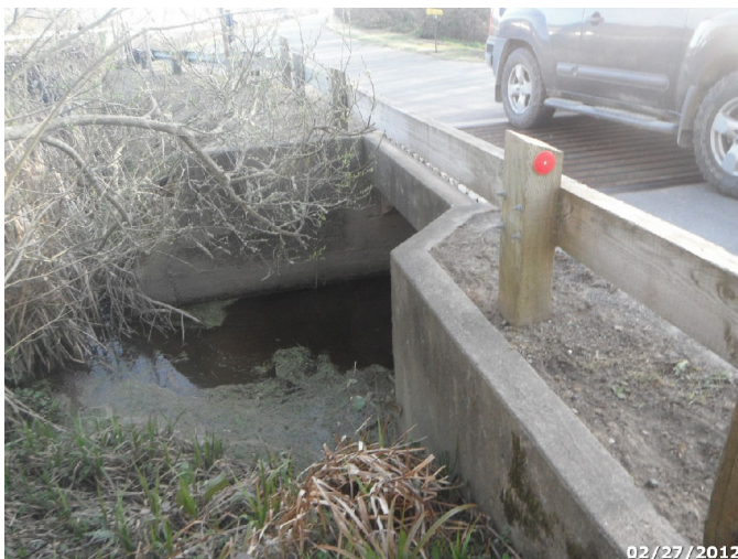
Photo: HUBA_C4_1593 Route: 010-002-0.63 Concrete Culvert Box 24ft long 6ft x 10ft 1ft deep Asset# NA
