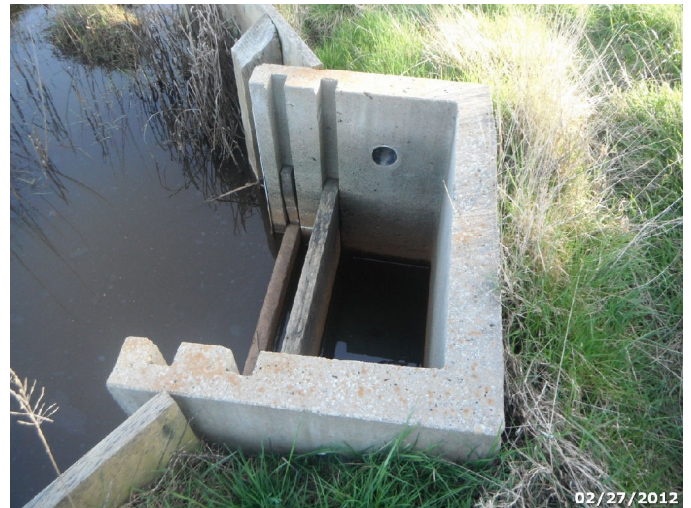
Photo: HUBA_C4_1599 Route: 102-001-0.21 Metal WCS Flashboard Riser 40ft long 24in dia. 3ft deep Asset# NA
