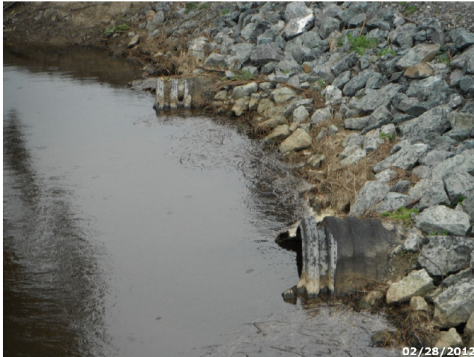
Photo: HUBA_C4_1674 Route: 400-001-0.05 Plastic Culvert 40ft long 48in dia. 2ft deep Asset# 10000105
