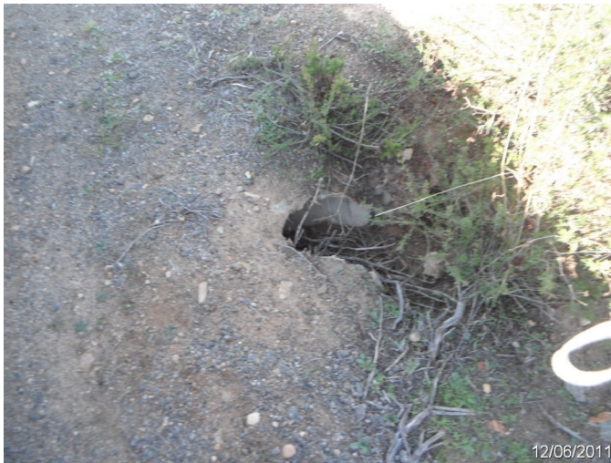
Photo: SADI_C4_0150 Route: 400-001-0.21 Concrete Culvert 25ft long 12in dia. 1ft deep Asset# 10001887
