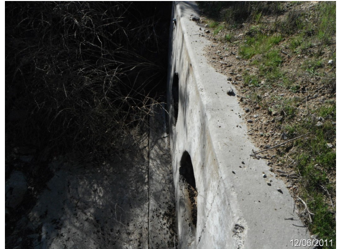
Photo: SADI_C4_0159 Route: 401-001-0.3 Metal Culvert 30ft long 15in dia. 2ft deep Asset# 10001877
