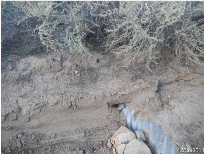
Photo: SADI_C4_0123 Route: 405-002-0.41 Metal Culvert 15ft long 18in dia. 1ft deep Asset# 10001929
