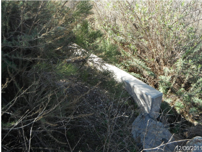
Photo: SADI_C4_0160 Route: 401-001-0.3 Metal Culvert 30ft long 15in dia. 2ft deep Asset# 10001877
