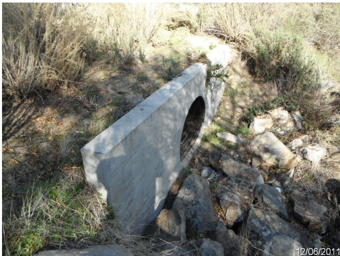
Photo: SADI_C4_0162 Route: 401-001-0.55 Metal Culvert 30ft long 48in dia. 1ft deep Asset# 10001877
