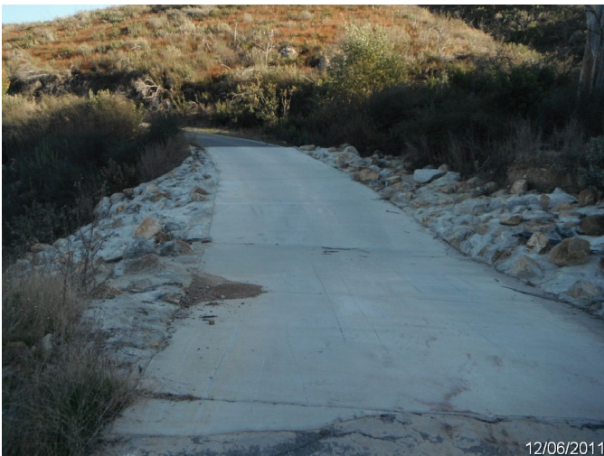
Photo: SADI_C4_0176 Route: 403-003-1.3 Concrete Low Water Xing 61.0ft long 15.0ft wide Asset# NA
