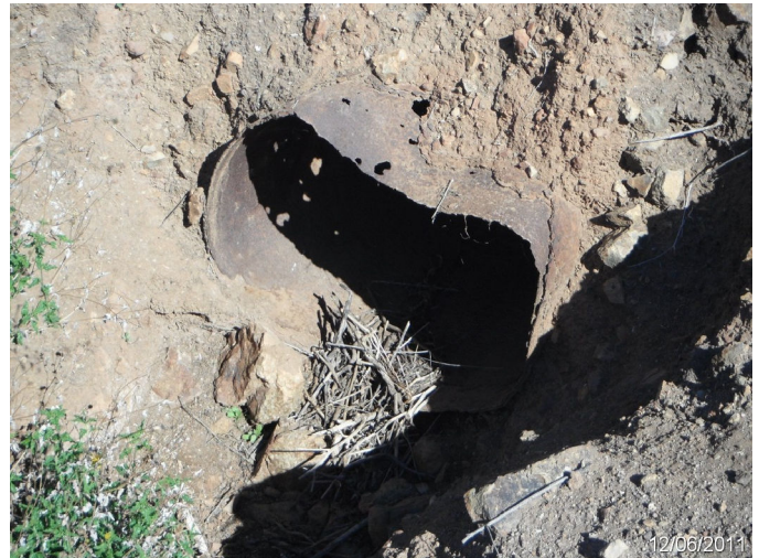
Photo: SADI_C4_0147 Route: 400-001-0.12 Metal Culvert 30ft long 36in dia. 3ft deep Asset# 10001887
