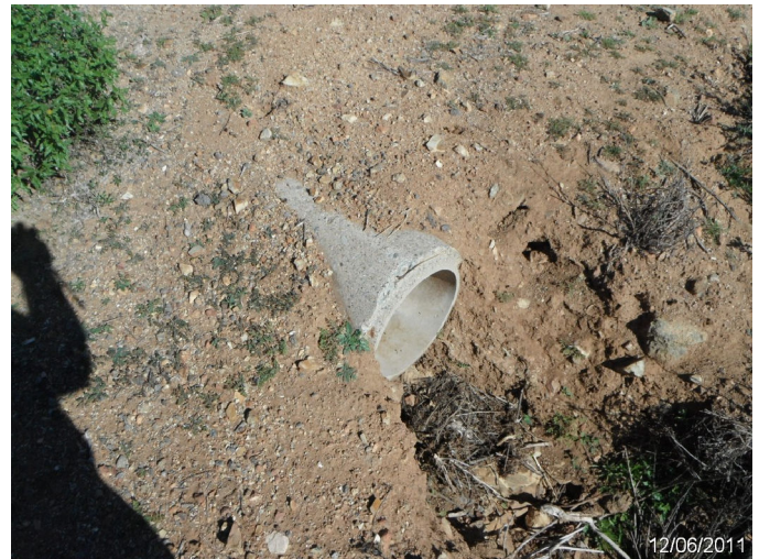
Photo: SADI_C4_0151 Route: 400-001-0.21 Concrete Culvert 25ft long 12in dia. 1ft deep Asset# 10001887
