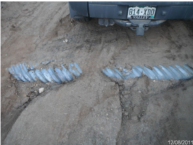
Photo: SADI_C4_0121 Route: 405-002-0.3 Deficiency Culvert Replace Asset# 10001929
