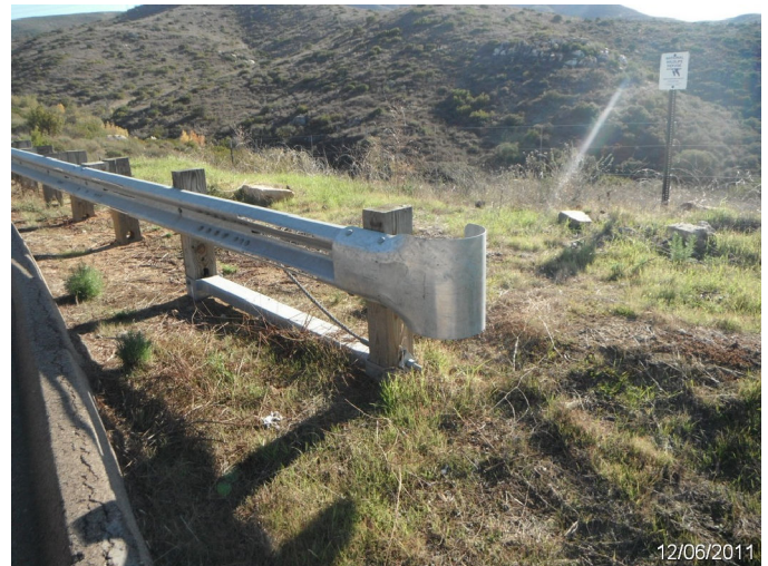
Photo: SADI_C4_0171 Route: 100-001-0.42 Guard_Guide_Rail Guardrail Galvanized_Steel 899.0 ft long Asset# 10001862
