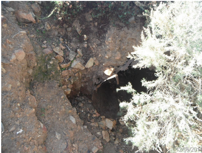
Photo: SADI_C4_0146 Route: 400-001-0.12 Metal Culvert 30ft long 36in dia. 3ft deep Asset# 10001887
