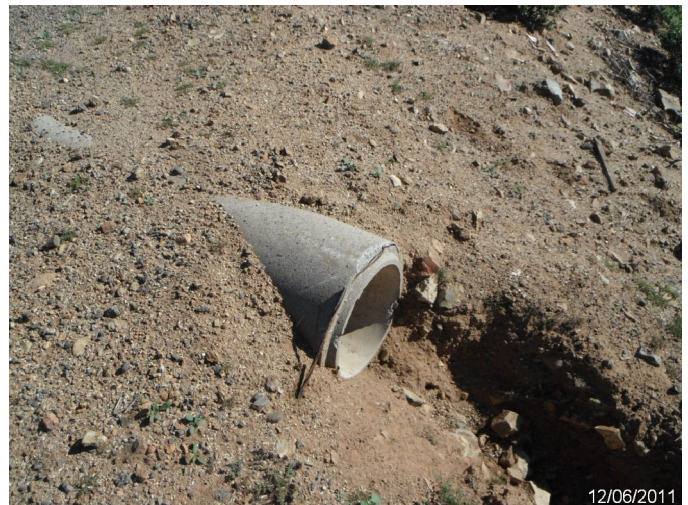
Photo: SADI_C4_0149 Route: 400-001-0.15 Concrete Culvert 25ft long 12in dia. 1ft deep Asset# 10001887
