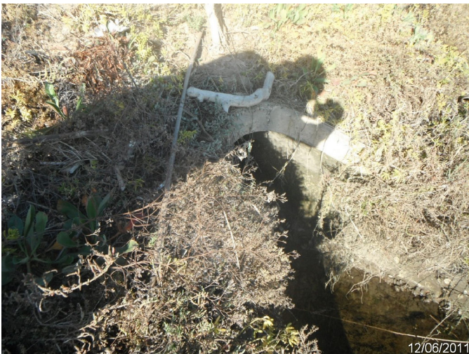
Photo: SDBA_C4_0025 Route: 300-001-0.16 Concrete Culvert 26ft long 48in dia. 4ft deep Asset# NA
