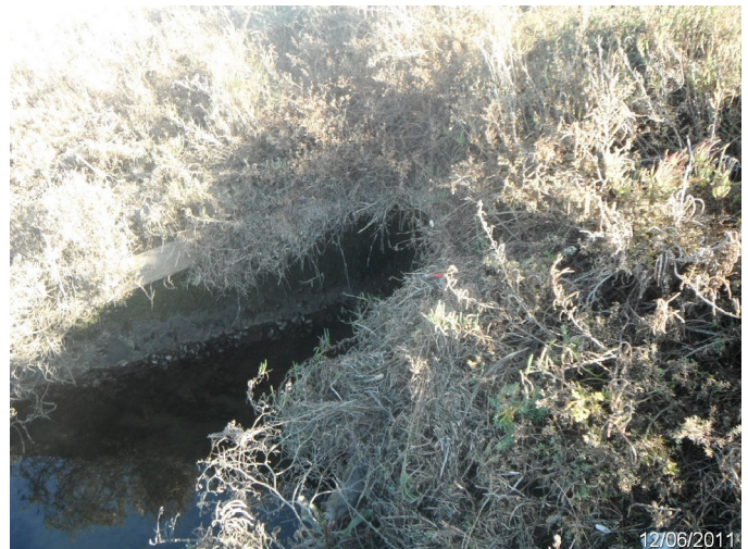
Photo: SDBA_C4_0026 Route: 300-001-0.16 Concrete Culvert 26ft long 48in dia. 4ft deep Asset# NA
