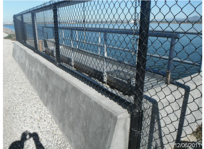
Photo: SDBA_C4_0011 Route: 400-003-2.63 Concrete WCS Flashboard Riser 25ft long 0in dia. 1ft deep 5x4 Box Asset# 10065493
