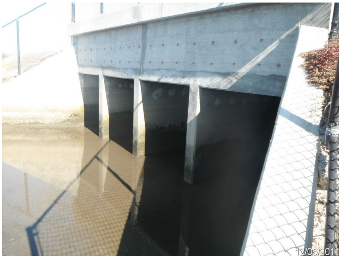
Photo: SDBA_C4_0012 Route: 400-003-2.63 Concrete WCS Flashboard Riser 25ft long 0in dia. 1ft deep 5x4 Box Asset# 10065493
