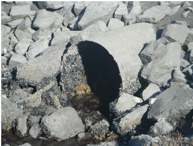
Photo: SEBE_C4_0140 Route: 406-001-0.0 Metal Culvert 61ft long 48in dia. 7ft deep Asset# 10048167
