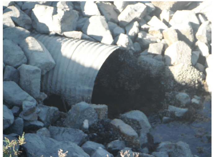
Photo: SEBE_C4_0141 Route: 406-001-0.0 Metal Culvert 61ft long 48in dia. 7ft deep Asset# 10048167
