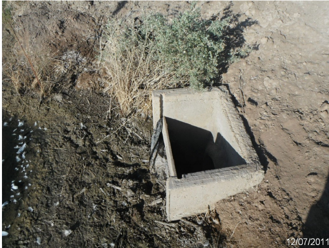
Photo: SASE_C4_0066 Route: 402-002-1.62 Plastic WCS Flashboard Riser 40ft long 18in dia. 2ft deep Asset# 10000660
