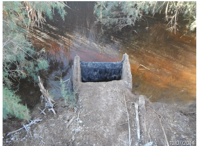
Photo: SASE_C4_0052 Route: 401-001-0.63 Plastic WCS Flashboard Riser 30ft long 18in dia. 1ft deep Asset# 10000671
