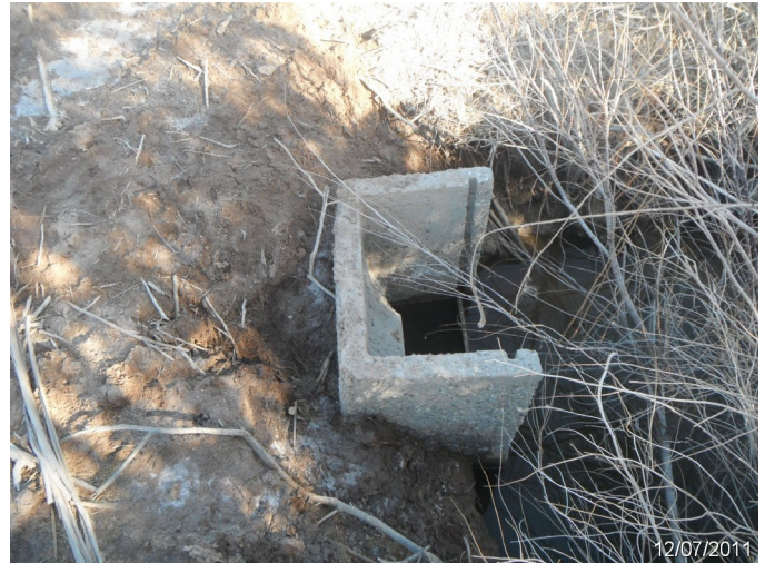
Photo: SASE_C4_0059 Route: 402-001-0.5 Plastic WCS Flashboard Riser 35ft long 18in dia. 2ft deep Asset# 10000660
