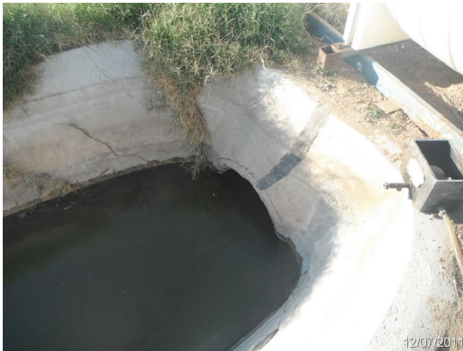
Photo: SASE_C4_0086 Route: 404-001-0.59 Concrete Culvert 25ft long 36in dia. 1ft deep Asset# 10000644
