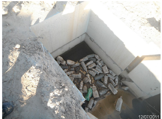
Photo: SASE_C4_0101 Route: 405-002-1.52 Plastic WCS Flashboard Riser 30ft long 12in dia. 3ft deep Asset# 10000665 8-014
