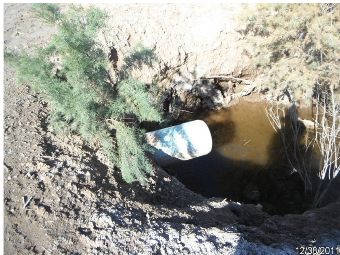
Photo: SASE_C4_0311 Route: 102-001-0.36 Plastic WCS Flashboard Riser 40ft long 18in dia. 2ft deep Asset# NA
