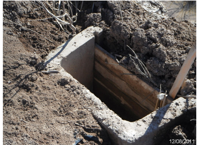
Photo: SASE_C4_0268 Route: 411-003-0.49 Concrete WCS Flashboard Riser 25ft long 12in dia. 2ft deep Asset# 10000655
