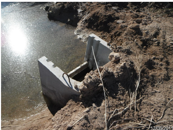
Photo: SASE_C4_0317 Route: 412-002-1.15 Plastic WCS Flashboard Riser 50ft long 18in dia. 3ft deep Asset# 10000694
