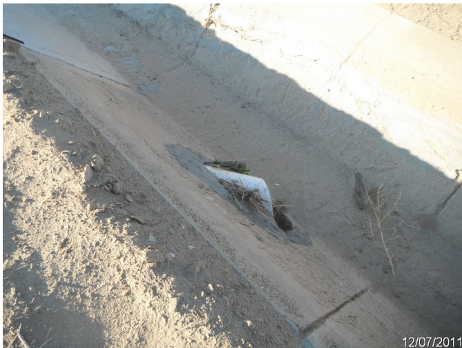
Photo: SASE_C4_0094 Route: 405-001-0.78 Plastic WCS Flashboard Riser 60ft long 12in dia. 2ft deep Asset# 10000665
