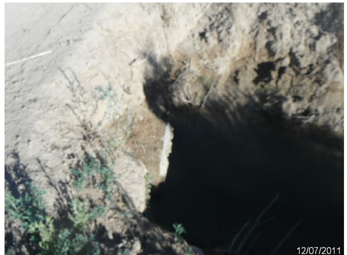
Photo: SASE_C4_0063 Route: 402-002-1.06 Concrete Culvert 15ft long 36in dia. 1ft deep Asset# 10000660
