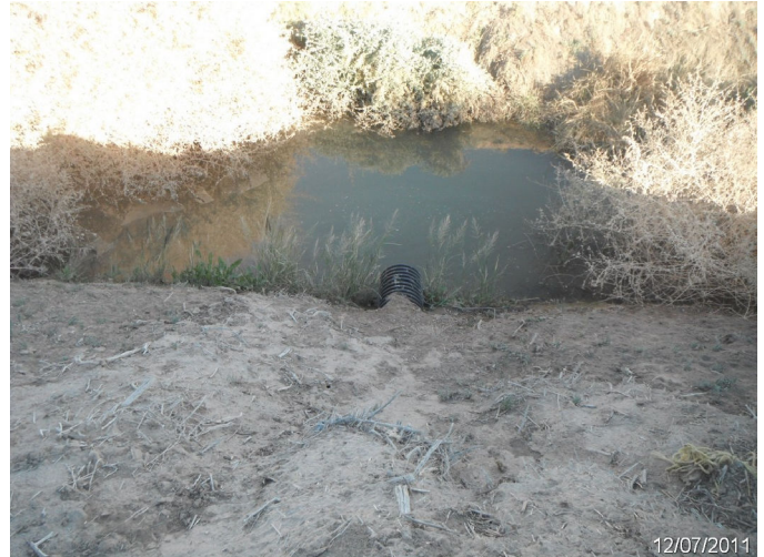
Photo: SASE_C4_0082 Route: 404-001-0.4 Plastic WCS Flashboard Riser 60ft long 12in dia. 20ft deep Unable to locate inlet Asset# 10000644
