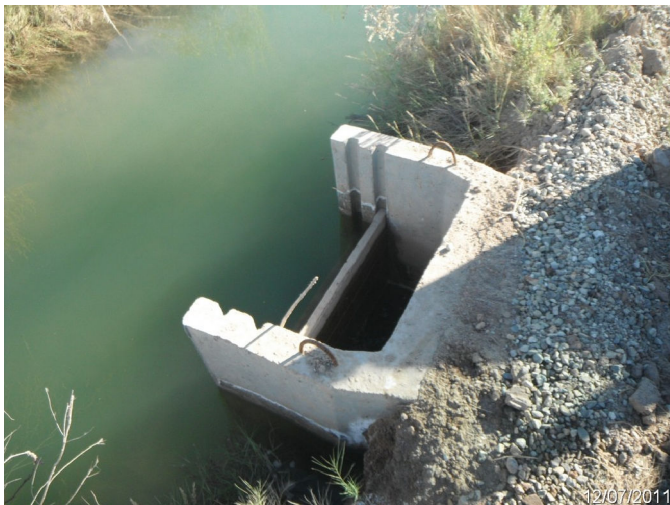
Photo: SASE_C4_0049 Route: 400-002-1.81 Plastic WCS Flashboard Riser 20ft long 18in dia. 2ft deep Asset# 10000670
