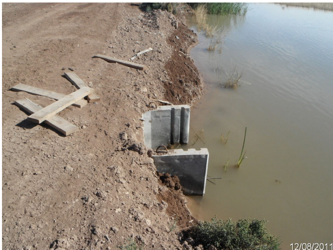
Photo: SASE_C4_0293 Route: 411-002-0.58 Plastic WCS Flashboard Riser 40ft long 18in dia. 3ft deep Asset# 10000655
