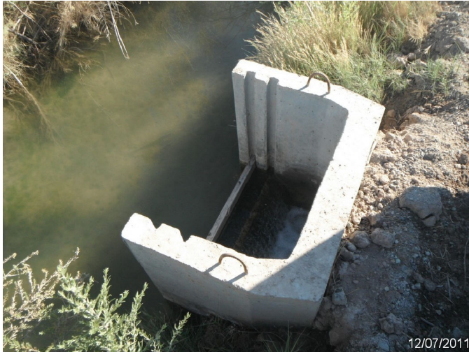
Photo: SASE_C4_0047 Route: 400-002-1.69 Plastic WCS Flashboard Riser 20ft long 18in dia. 2ft deep Asset# 10000670
