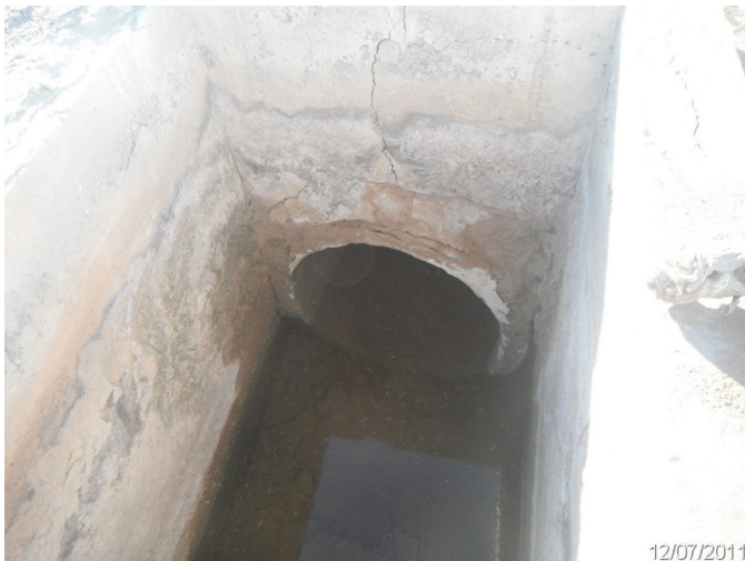
Photo: SASE_C4_0077 Route: 403-001-0.99 Metal Culvert 50ft long 48in dia. 1ft deep Asset# 10000672
