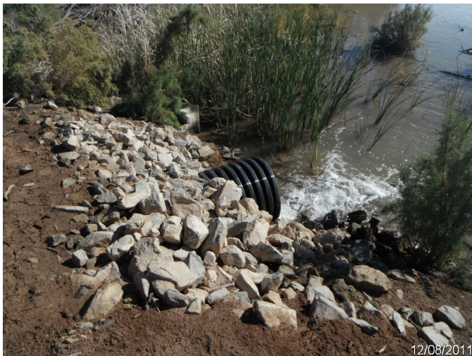
Photo: SASE_C4_0332 Route: 410-003-1.51 Plastic WCS Flashboard Riser 25ft long 24in dia. 2ft deep Asset# 10000656
