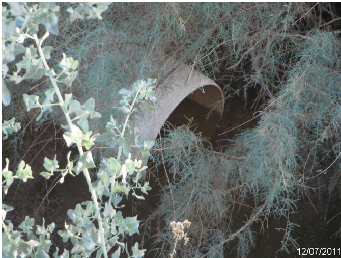
Photo: SASE_C4_0213 Route: 408-001-0.13 Plastic WCS Flashboard Riser 20ft long 12in dia. 6ft deep Asset# 10000695
