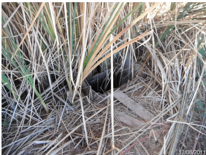
Photo: SASE_C4_0312 Route: 102-001-0.36 Plastic WCS Flashboard Riser 40ft long 18in dia. 2ft deep Asset# NA
