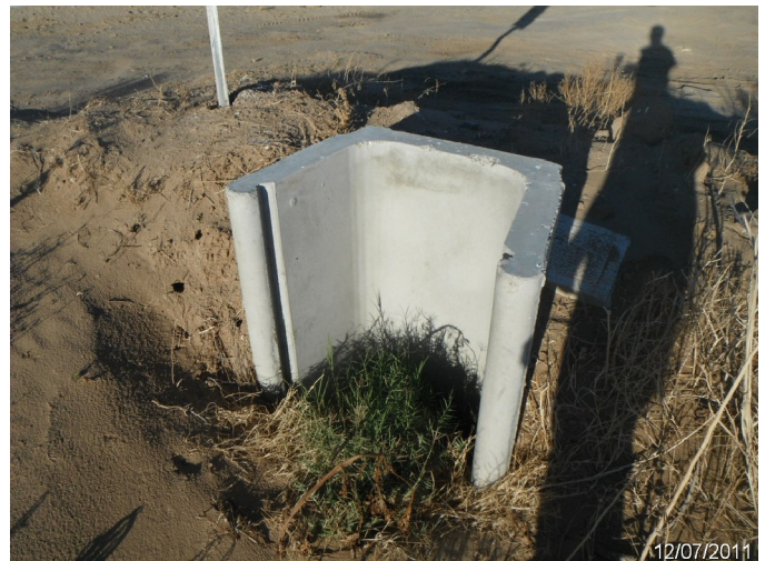
Photo: SASE_C4_0095 Route: 405-001-0.78 Plastic WCS Flashboard Riser 60ft long 12in dia. 2ft deep Asset# 10000665 8-013
