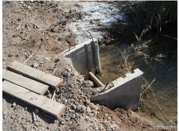
Photo: SASE_C4_0282 Route: 411-003-0.84 Plastic WCS Flashboard Riser 30ft long 18in dia. 3ft deep Asset# 10000655
