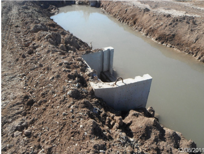
Photo: SASE_C4_0330 Route: 410-003-1.3 Plastic WCS Flashboard Riser 20ft long 18in dia. 2ft deep Asset# 10000656
