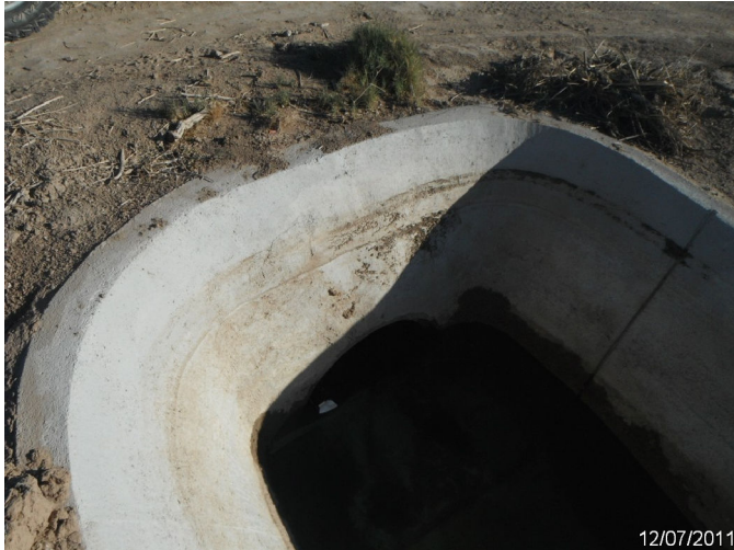
Photo: SASE_C4_0081 Route: 404-001-0.37 Concrete Culvert 20ft long 36in dia. 1ft deep Asset# 10000644
