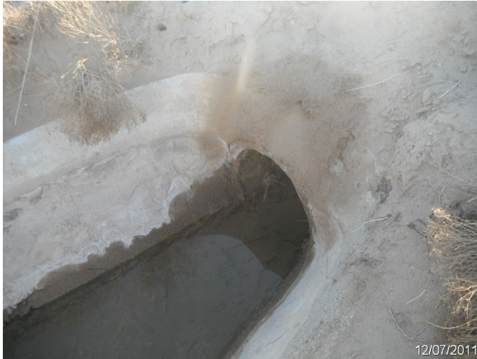
Photo: SASE_C4_0092 Route: 405-001-0.64 Concrete WCS Flap Gate/Full-Round Riser 30ft long 36in dia. 2ft deep Asset# 10000665
