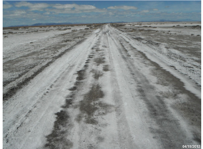
Photo: STIL_C4_1217 Route: 104-009-8.47 Other 1218 Problem area 2 road needs to be built up to prevent wind and water from washing it out
