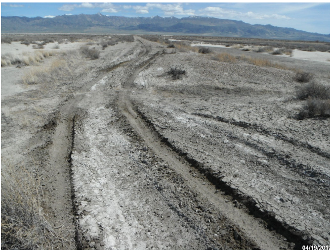
Photo: STIL_C4_1245 Route: 416-003-2.7 Problem Area Road Washed out
