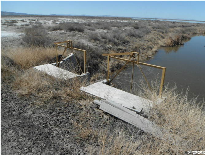
Photo: STIL_C4_1305 Route: 104-007-6.82 Plastic WCS Flap Gate/Full-Round Riser 40ft long 48in dia. 2ft deep Asset# NA
