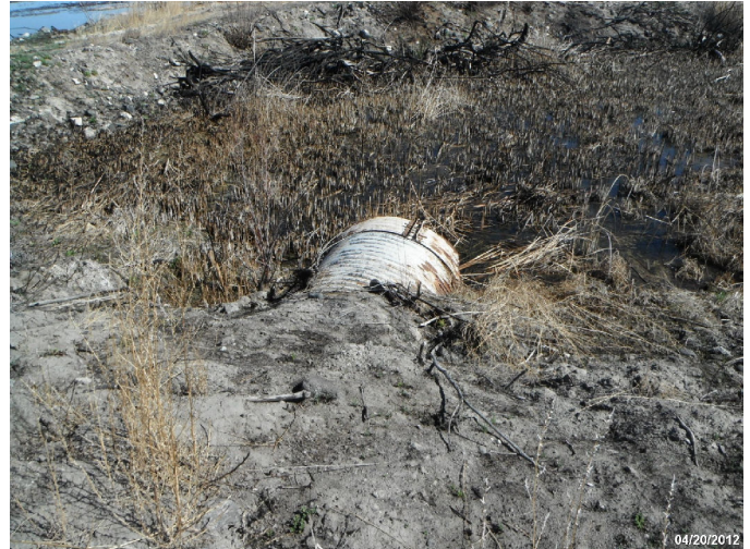
Photo: STIL_C4_1269 Route: 104-001-0.31 Metal WCS Flashboard Riser 35ft long 48in dia. 2ft deep Asset# NA
