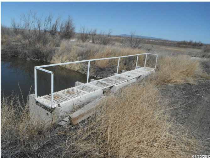
Photo: STIL_C4_1292 Route: 109-003-2.47 Plastic WCS Flashboard Riser 45ft long 48in dia. 2ft deep Asset# NA
