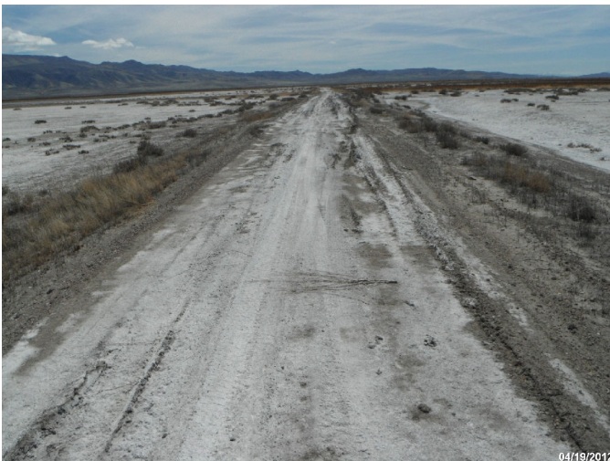
Photo: STIL_C4_1219 Route: 104-009-8.7 Other 1220, Problem area 2 road needs to be built up
