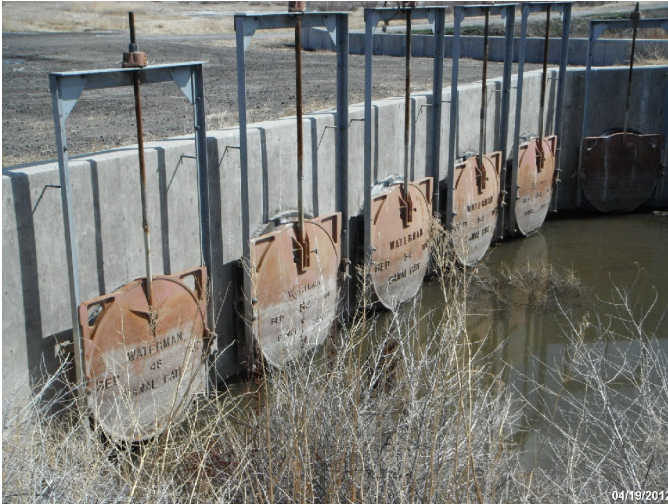
Photo: STIL_C4_1173 Route: 101-001-0.01 Plastic WCS Screw Gate 90ft long 48in dia. 3ft deep Asset# NA
