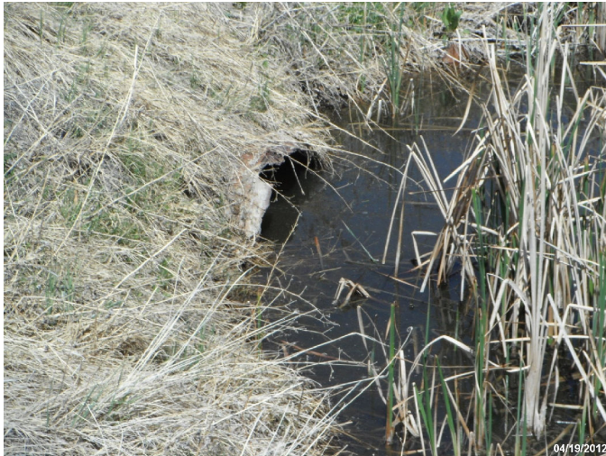
Photo: STIL_C4_1224 Route: 104-009-8.83 Metal WCS Flashboard Riser 35ft long 36in dia. 3ft deep Asset# NA
