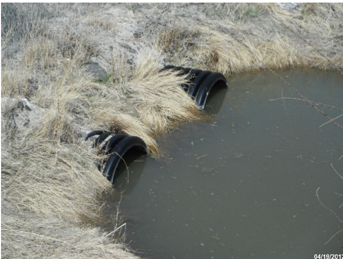
Photo: STIL_C4_1193 Route: 101-005-4.79 Plastic WCS Flashboard Riser 40ft long 24in dia. 4ft deep Asset# NA
