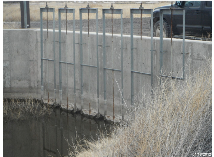
Photo: STIL_C4_1026 Route: 107-001-0.19 Metal WCS Screw Gate 65ft long 24in dia. 8ft deep Asset# NA
