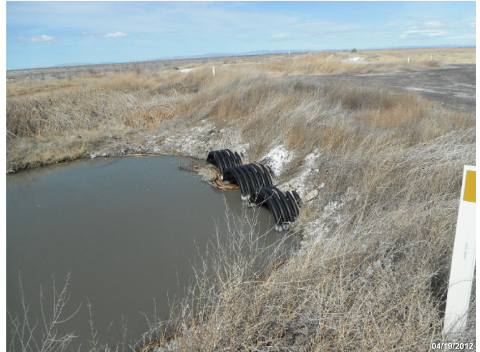
Photo: STIL_C4_1181 Route: 101-004-3.35 Plastic WCS Flashboard Riser 60ft long 36in dia. 3ft deep Asset# NA
