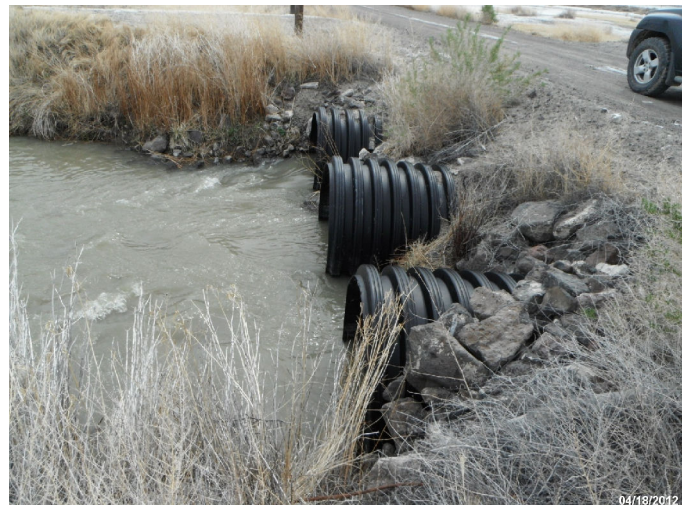
Photo: STIL_C4_1042 Route: 103-005-4.4 Plastic Culvert 35ft long 60in dia. 2ft deep Asset# NA
