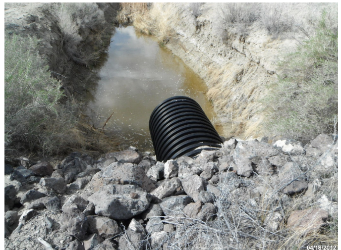
Photo: STIL_C4_1137 Route: 010-003-2.7 Plastic WCS Flap Gate/Full-Round Riser 40ft long 60in dia. 4ft deep Asset# NA
