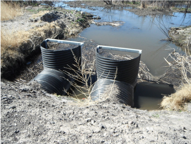
Photo: STIL_C4_1268 Route: 104-001-0.27 Metal WCS Flashboard Riser 35ft long 48in dia. 2ft deep Asset# NA
