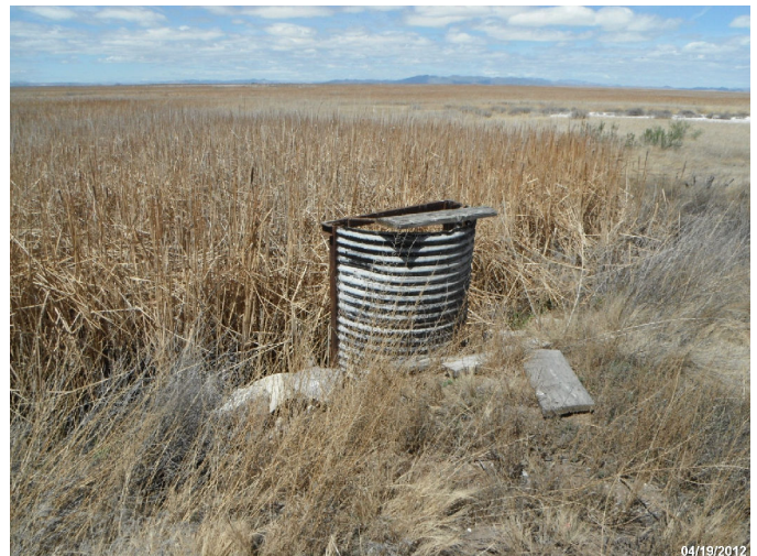
Photo: STIL_C4_1223 Route: 104-009-8.83 Metal WCS Flashboard Riser 35ft long 36in dia. 3ft deep Asset# NA 8-018
