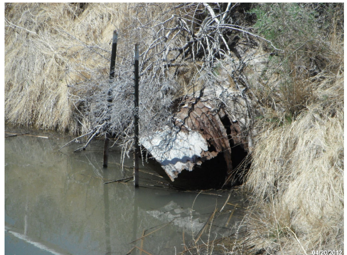
Photo: STIL_C4_1310 Route: 104-008-7.7 Metal Culvert 40ft long 48in dia. 4ft deep Asset# NA
