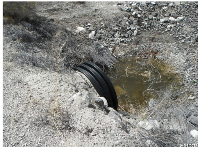
Photo: STIL_C4_1108 Route: 410-002-1.87 Plastic WCS Flap Gate/Full-Round Riser 30ft long 60in dia. 2ft deep Asset# NA
