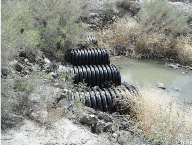
Photo: STIL_C4_1115 Route: 412-001-0.34 Plastic WCS Flap Gate/Full-Round Riser 40ft long 60in dia. 4ft deep Asset# NA
