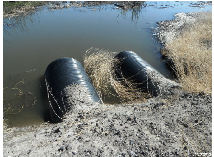
Photo: STIL_C4_1267 Route: 104-001-0.27 Metal WCS Flashboard Riser 35ft long 48in dia. 2ft deep Asset# NA
