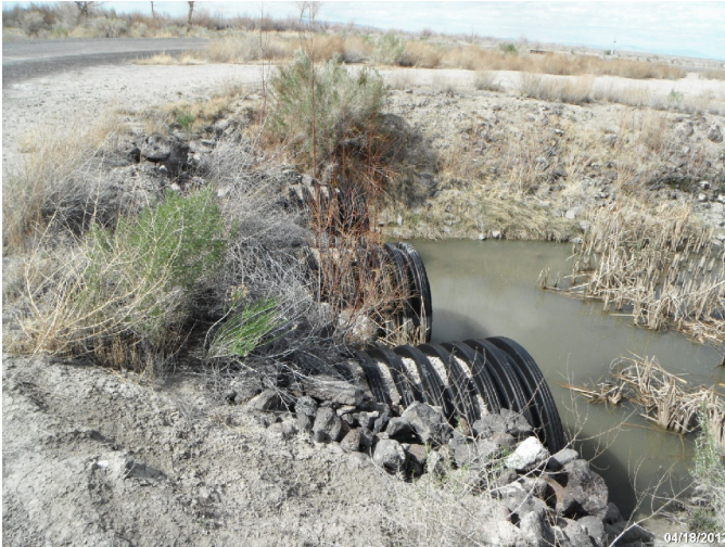
Photo: STIL_C4_1134 Route: 010-001-0.28 Plastic Culvert 40ft long 36in dia. 2ft deep Asset# NA
