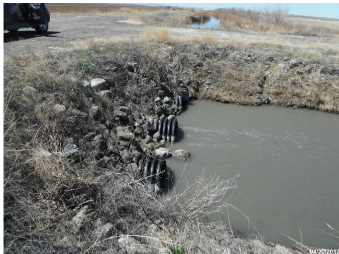
Photo: STIL_C4_1312 Route: 951 Plastic WCS Flap Gate/Full-Round Riser 40ft long 24in dia. 3ft deep Asset# NA
