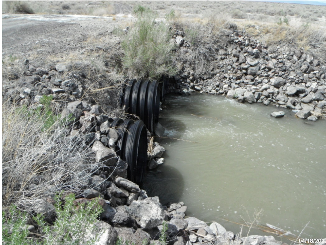
Photo: STIL_C4_1112 Route: 411-001-0.01 Plastic WCS Flap Gate/Full-Round Riser 40ft long 60in dia. 1ft deep Asset# NA
