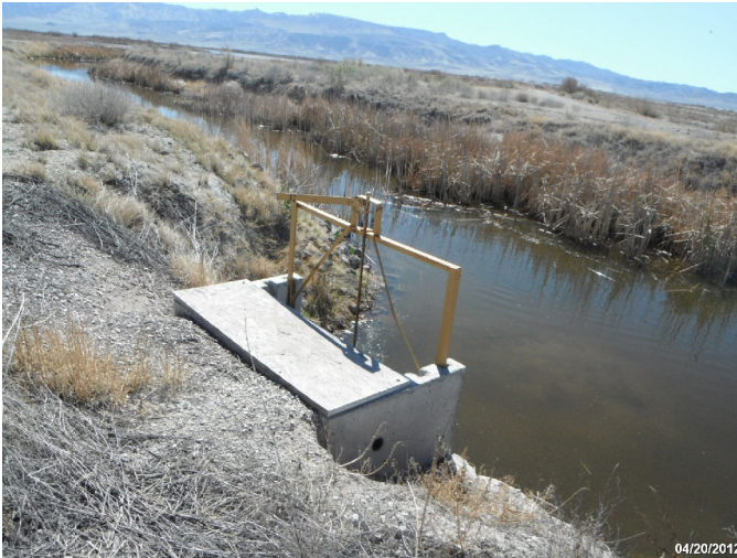
Photo: STIL_C4_1284 Route: 104-004-3.41 Plastic WCS Flap Gate/Full-Round Riser 40ft long 48in dia. 2ft deep Asset# NA
