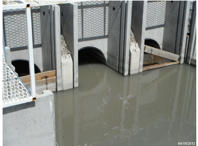
Photo: STIL_C4_1215 Route: 104-009-8.07 Plastic WCS Flashboard Riser 60ft long 36in dia. 2ft deep Asset# NA
