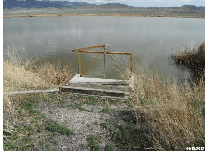
Photo: STIL_C4_1143 Route: 010-005-3.92 Plastic WCS Flap Gate/Full-Round Riser 50ft long 60in dia. 3ft deep Asset# NA
