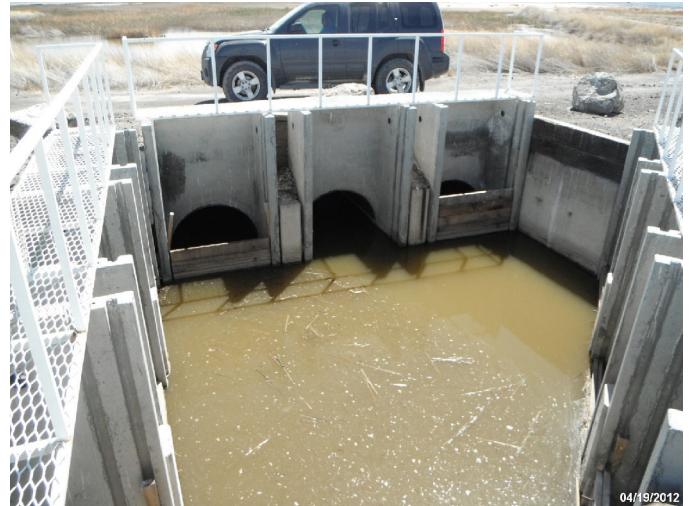
Photo: STIL_C4_1227 Route: 105-001-0.0 Plastic WCS Flashboard Riser 50ft long 36in dia. 3ft deep Asset# NA
