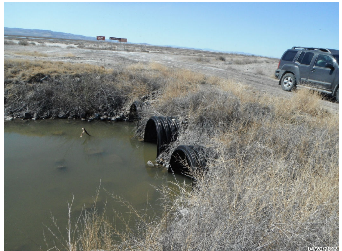
Photo: STIL_C4_1293 Route: 109-003-2.47 Plastic WCS Flashboard Riser 45ft long 48in dia. 2ft deep Asset# NA 8-025
