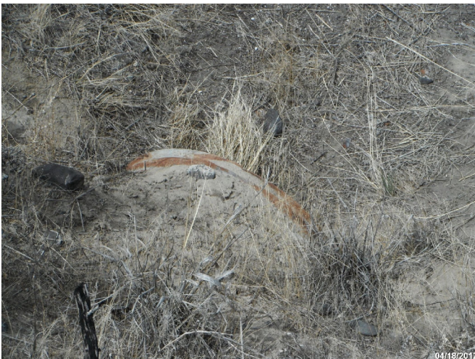
Photo: STIL_C4_1089 Route: 408-003-2.16 Metal WCS Flashboard Riser 30ft long 36in dia. 3ft deep Asset# NA
