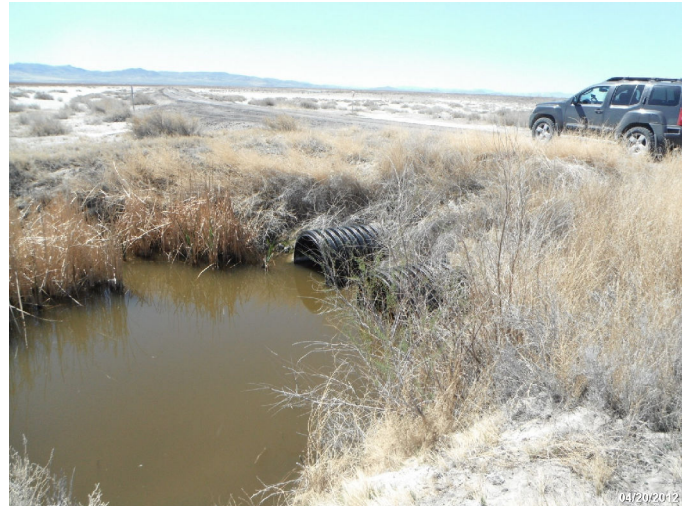
Photo: STIL_C4_1306 Route: 104-007-6.82 Plastic WCS Flap Gate/Full-Round Riser 40ft long 48in dia. 2ft deep Asset# NA
