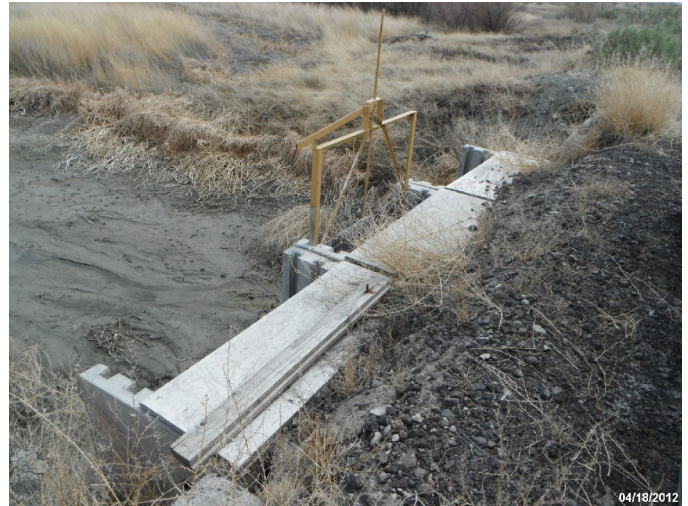
Photo: STIL_C4_1104 Route: 410-001-0.49 Plastic WCS Flap Gate/Full-Round Riser 30ft long 48in dia. 4ft deep Asset# NA
