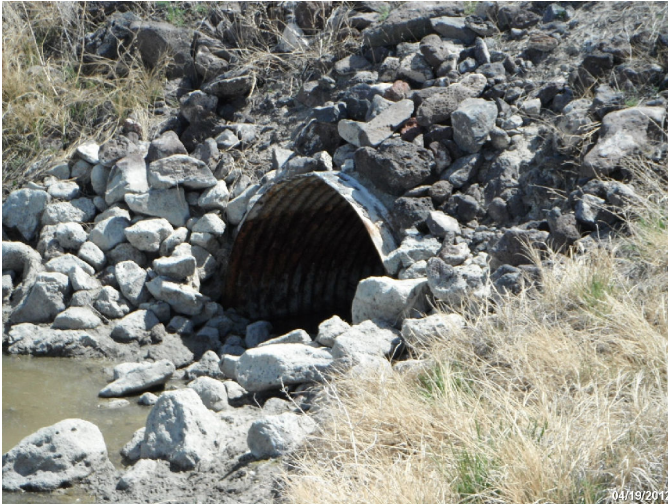
Photo: STIL_C4_1203 Route: 102-004-3.55 Metal Culvert 40ft long 48in dia. 3ft deep Asset# NA
