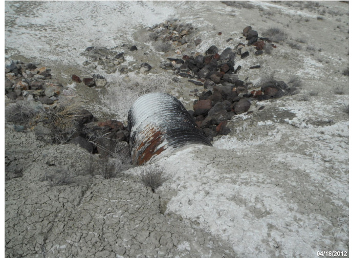
Photo: STIL_C4_1069 Route: 405-001-0.01 Metal WCS Flashboard Riser 70ft long 60in dia. 8ft deep Asset# NA
