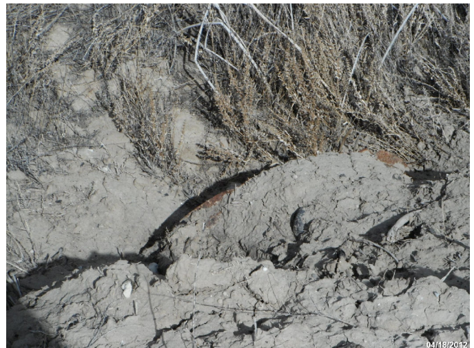
Photo: STIL_C4_1096 Route: 408-004-3.76 Metal WCS Flashboard Riser 30ft long 36in dia. 3ft deep Asset# NA 8-045
