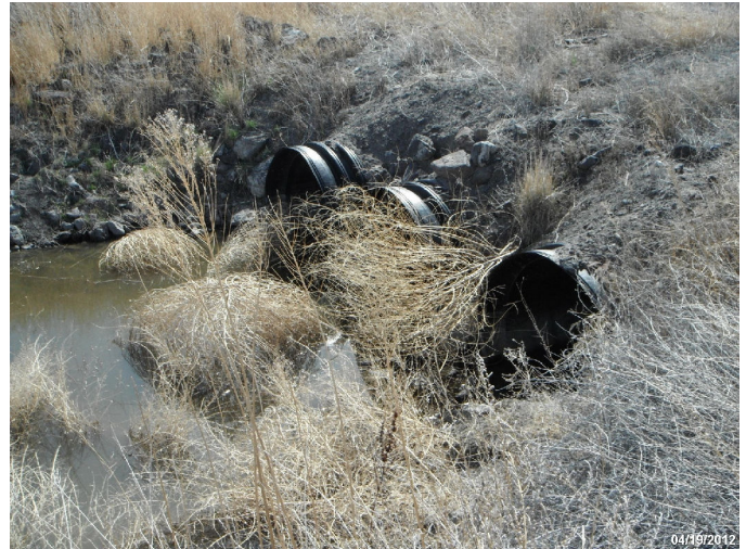
Photo: STIL_C4_1172 Route: 101-001-0.01 Plastic WCS Screw Gate 90ft long 48in dia. 3ft deep Asset# NA
