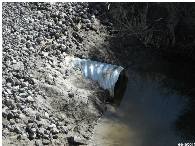
Photo: STIL_C4_1167 Route: 950 Metal Culvert 60ft long 24in dia. 9ft deep Asset# NA
