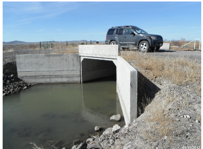
Photo: STIL_C4_1160 Route: 300-001-0.03 Concrete WCS Screw Gate 40ft long Nonein dia. 2ft deep 6 x 10 box Asset# NA 8-033
