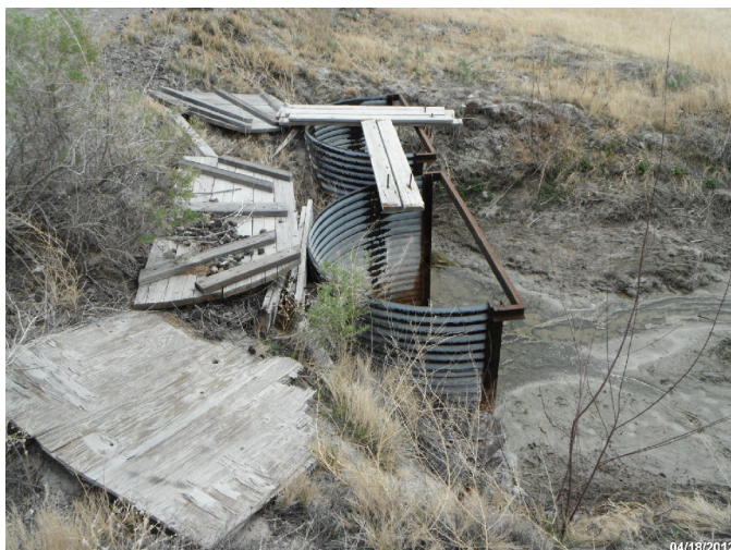
Photo: STIL_C4_1054 Route: 103-003-2.01 Metal WCS Flashboard Riser 40ft long 48in dia. 4ft deep Asset# NA
