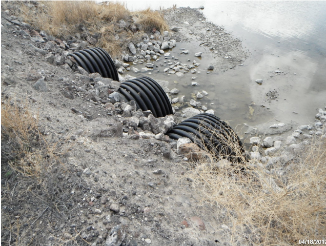
Photo: STIL_C4_1105 Route: 410-001-0.49 Plastic WCS Flap Gate/Full-Round Riser 30ft long 48in dia. 4ft deep Asset# NA
