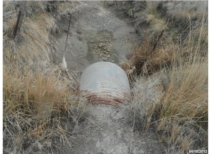
Photo: STIL_C4_1019 Route: 100-003-2.48 Metal WCS Flashboard Riser 50ft long 48in dia. 2ft deep Asset# NA
