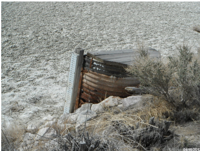
Photo: STIL_C4_1063 Route: 404-001-0.58 Metal WCS Flashboard Riser 50ft long 36in dia. 6ft deep Asset# NA
