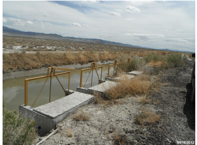
Photo: STIL_C4_1114 Route: 412-001-0.34 Plastic WCS Flap Gate/Full-Round Riser 40ft long 60in dia. 4ft deep Asset# NA
