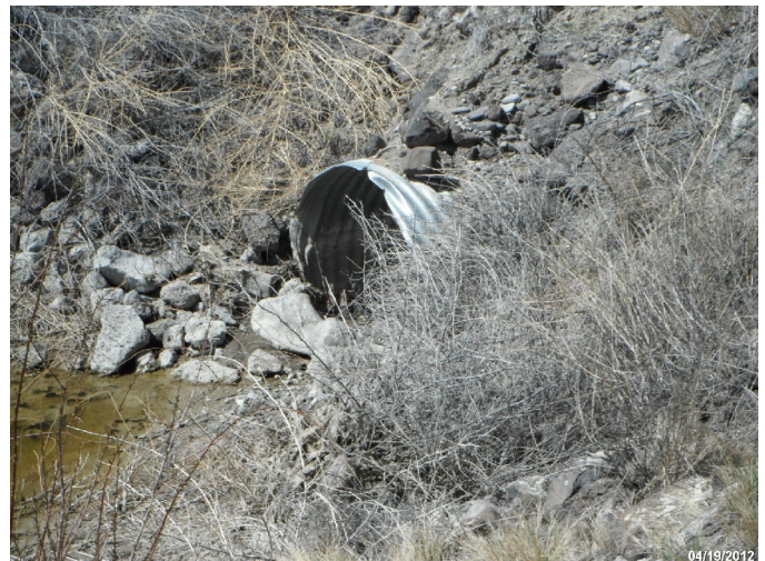
Photo: STIL_C4_1200 Route: 102-003-2.12 Metal Culvert 40ft long 48in dia. 6ft deep Asset# NA
