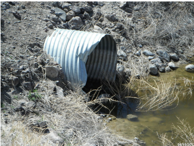
Photo: STIL_C4_1199 Route: 102-003-2.12 Metal Culvert 40ft long 48in dia. 6ft deep Asset# NA
