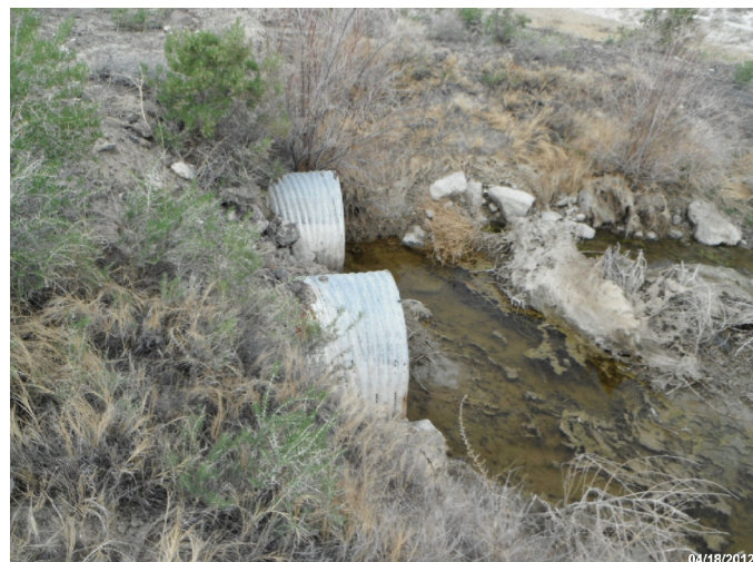
Photo: STIL_C4_1055 Route: 103-003-2.01 Metal WCS Flashboard Riser 40ft long 48in dia. 4ft deep Asset# NA 8-011
