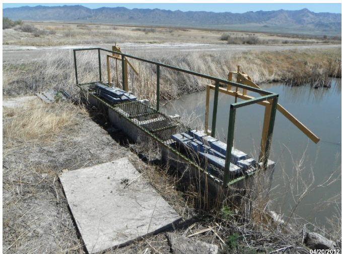
Photo: STIL_C4_1311 Route: 951 Plastic WCS Flap Gate/Full-Round Riser 40ft long 24in dia. 3ft deep Asset# NA
