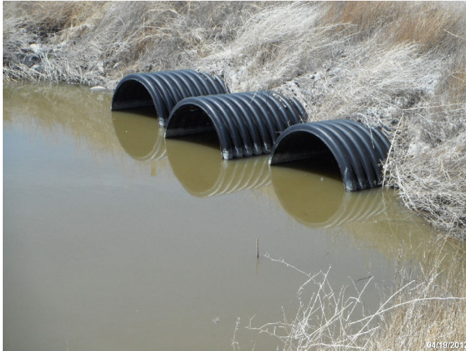
Photo: STIL_C4_1228 Route: 105-001-0.0 Plastic WCS Flashboard Riser 50ft long 36in dia. 3ft deep Asset# NA
