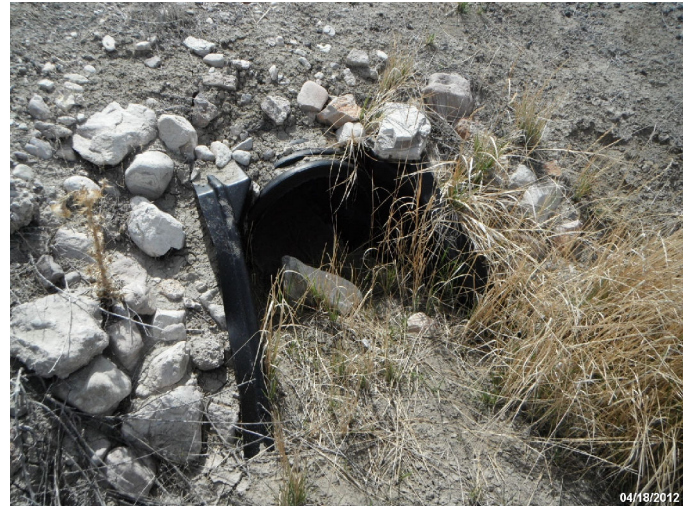
Photo: STIL_C4_1131 Route: 943 Plastic Culvert 30ft long 18in dia. 1ft deep Asset# 10036681
