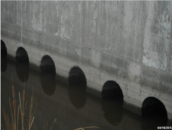
Photo: STIL_C4_1027 Route: 107-001-0.19 Metal WCS Screw Gate 65ft long 24in dia. 8ft deep Asset# NA
