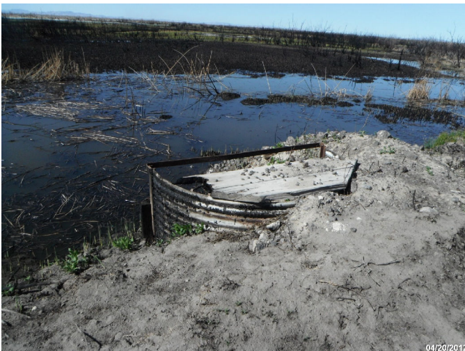
Photo: STIL_C4_1270 Route: 104-001-0.31 Metal WCS Flashboard Riser 35ft long 48in dia. 2ft deep Asset# NA
