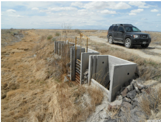
Photo: STIL_C4_1095 Route: 408-004-3.51 Plastic WCS Flashboard Riser 45ft long 48in dia. 3ft deep Asset# NA
