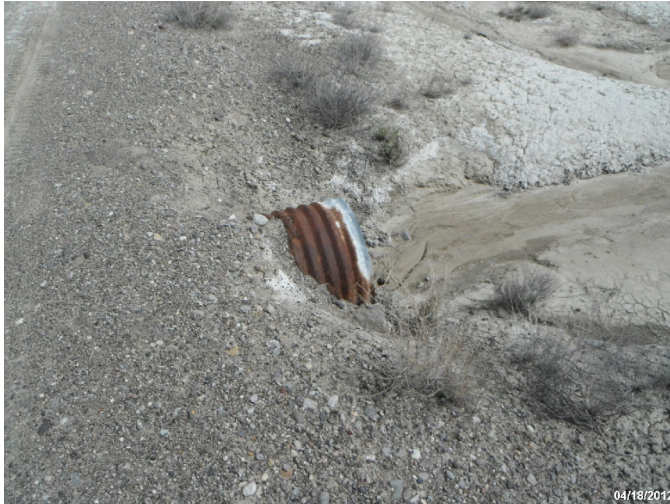
Photo: STIL_C4_1061 Route: 404-001-0.24 Metal Culvert 20ft long 24in dia. 1ft deep Asset# NA
