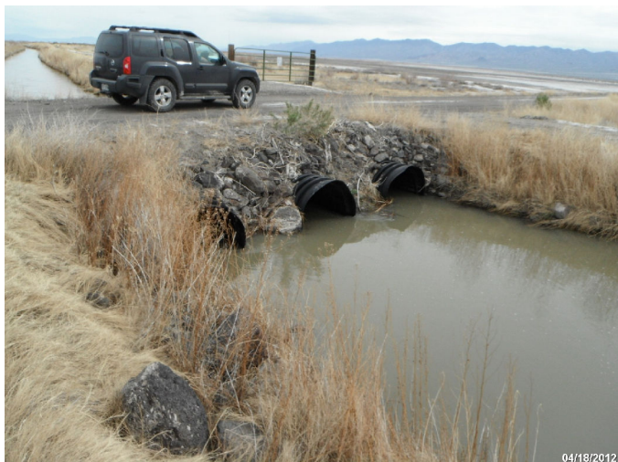
Photo: STIL_C4_1043 Route: 103-005-4.4 Plastic Culvert 35ft long 60in dia. 2ft deep Asset# NA
