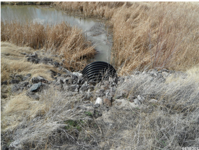
Photo: STIL_C4_1144 Route: 010-005-3.92 Plastic WCS Flap Gate/Full-Round Riser 50ft long 60in dia. 3ft deep Asset# NA
