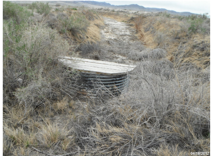
Photo: STIL_C4_1050 Route: 103-003-2.23 Metal WCS Flashboard Riser 35ft long 48in dia. 7ft deep Asset# NA
