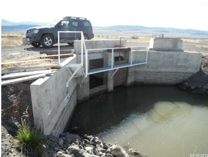
Photo: STIL_C4_1159 Route: 300-001-0.03 Concrete WCS Screw Gate 40ft long Nonein dia. 2ft deep 6 x 10 box Asset# NA
