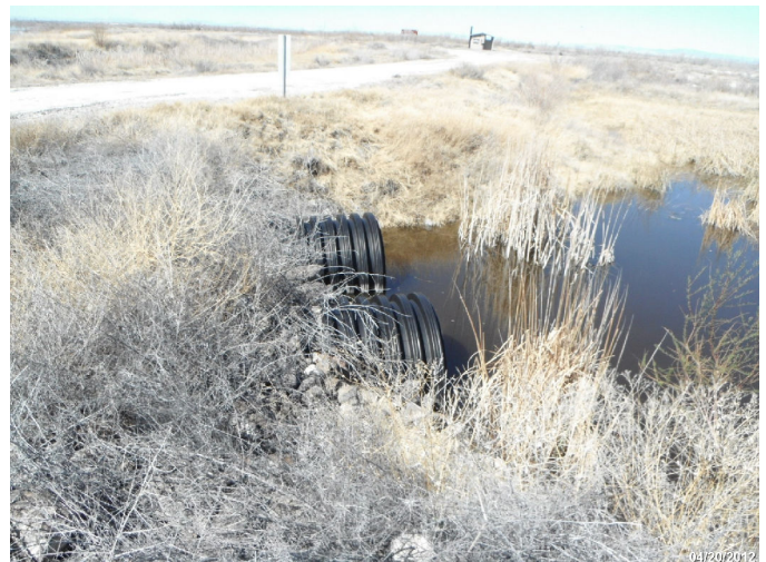
Photo: STIL_C4_1286 Route: 104-004-3.4 Plastic WCS Flap Gate/Full-Round Riser 50ft long 48in dia. 2ft deep Asset# NA
