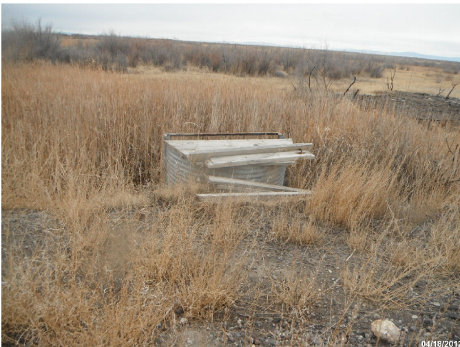
Photo: STIL_C4_1029 Route: 107-002-0.29 Metal WCS Flashboard Riser 40ft long 36in dia. 2ft deep Asset# NA
