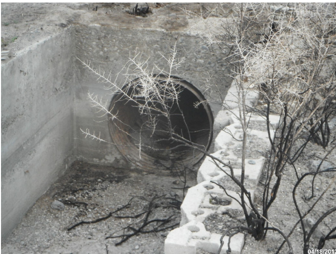
Photo: STIL_C4_1020 Route: 100-003-2.48 Metal WCS Flashboard Riser 50ft long 48in dia. 2ft deep Asset# NA
