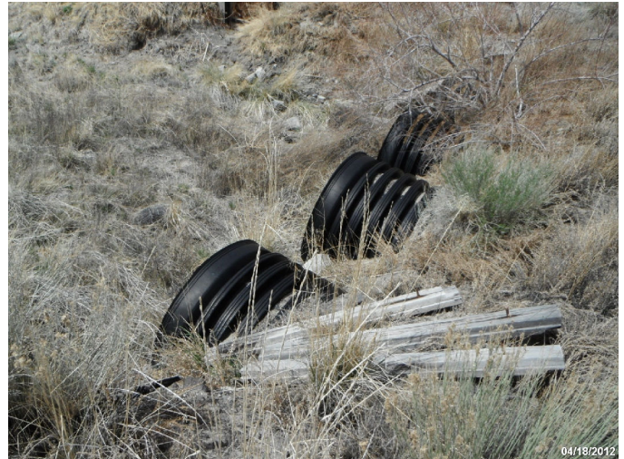
Photo: STIL_C4_1100 Route: 409-001-0.01 Plastic Culvert 30ft long 48in dia. 2ft deep Asset# NA
