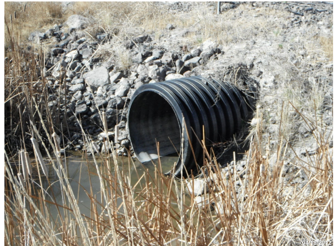
Photo: STIL_C4_1158 Route: 300-001-0.01 Plastic WCS Flap Gate/Full-Round Riser 40ft long 36in dia. 2ft deep Asset# NA
