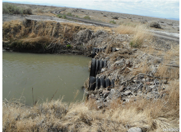
Photo: STIL_C4_1149 Route: 010-007-6.06 Plastic Culvert 40ft long 48in dia. 2ft deep Asset# NA
