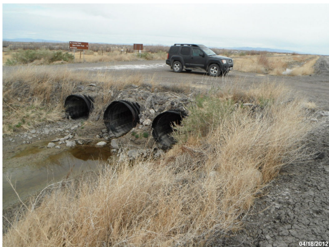
Photo: STIL_C4_1039 Route: 103-005-4.85 Plastic Culvert 40ft long 60in dia. 1ft deep Asset# NA
