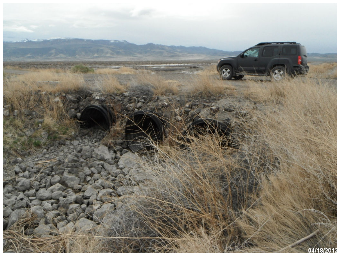
Photo: STIL_C4_1038 Route: 103-005-4.85 Plastic Culvert 40ft long 60in dia. 1ft deep Asset# NA
