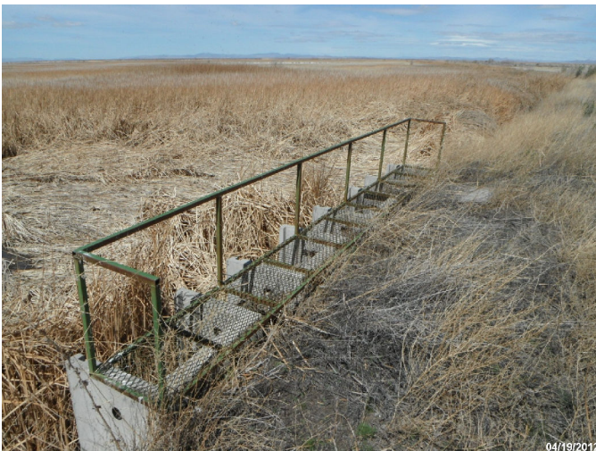
Photo: STIL_C4_1184 Route: 101-004-3.98 Plastic WCS Flashboard Riser 25ft long 24in dia. 2ft deep Asset# NA
