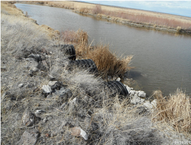
Photo: STIL_C4_1146 Route: 010-005-4.16 Plastic WCS Flap Gate/Full-Round Riser 40ft long 48in dia. 3ft deep Asset# NA
