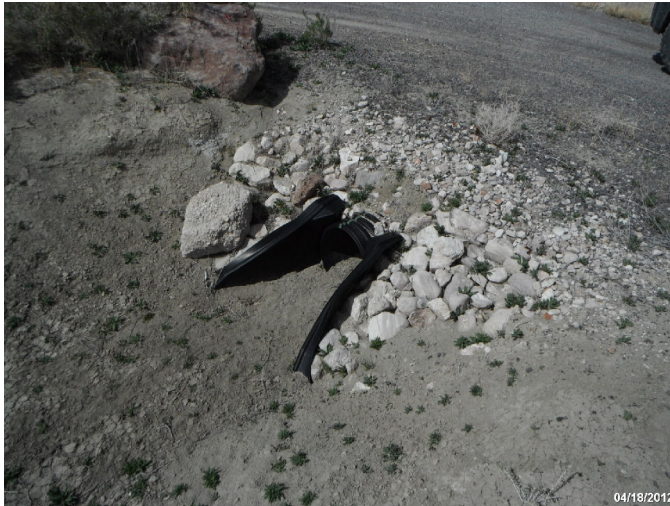
Photo: STIL_C4_1130 Route: 943 Plastic Culvert 30ft long 18in dia. 1ft deep Asset# 10036681
