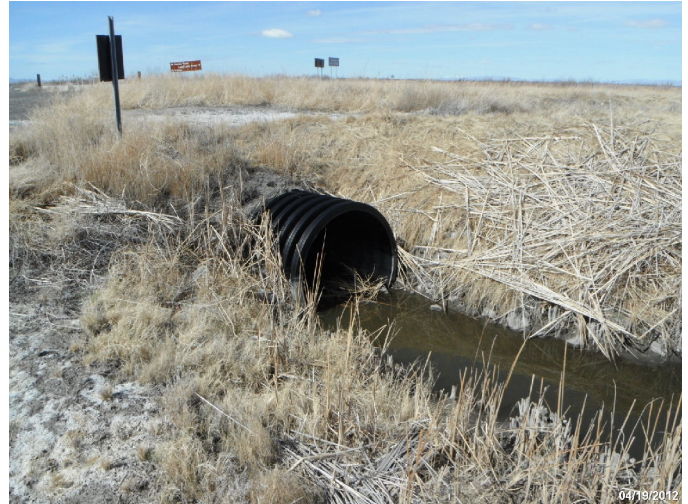
Photo: STIL_C4_1170 Route: 101-001-0.01 Plastic WCS Screw Gate 100ft long 36in dia. 3ft deep Asset# NA
