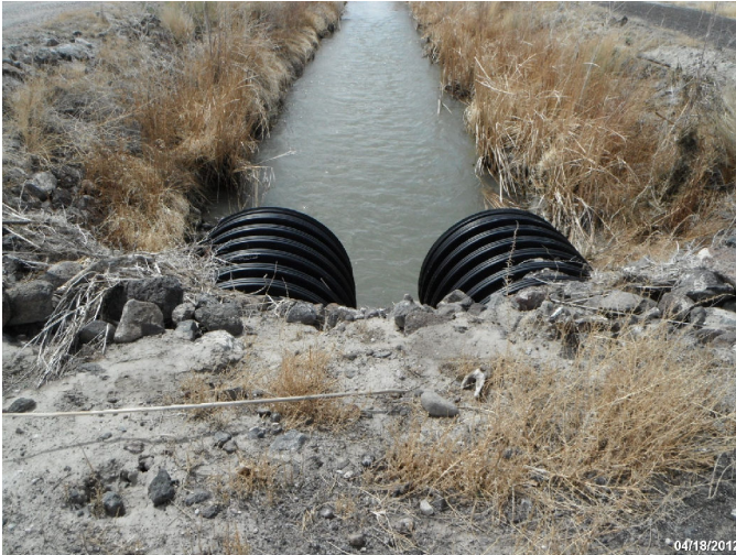
Photo: STIL_C4_1122 Route: 412-006-5.5 Plastic Culvert 120ft long 60in dia. 2ft deep Asset# NA
