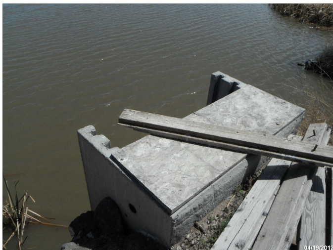
Photo: STIL_C4_1239 Route: 415-001-0.52 Plastic WCS Flashboard Riser 40ft long 48in dia. 1ft deep Asset# NA
