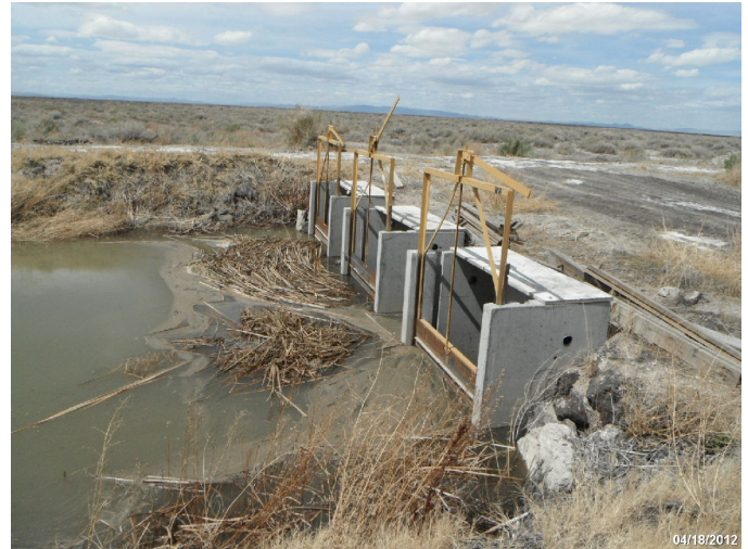
Photo: STIL_C4_1111 Route: 411-001-0.01 Plastic WCS Flap Gate/Full-Round Riser 40ft long 60in dia. 1ft deep Asset# NA
