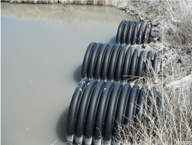
Photo: STIL_C4_1216 Route: 104-009-8.07 Plastic WCS Flashboard Riser 60ft long 36in dia. 2ft deep Asset# NA
