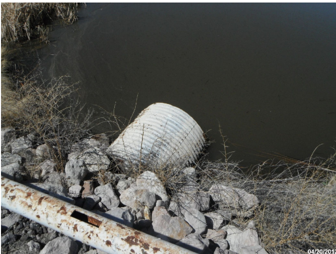
Photo: STIL_C4_1309 Route: 104-008-7.7 Metal Culvert 40ft long 48in dia. 4ft deep Asset# NA
