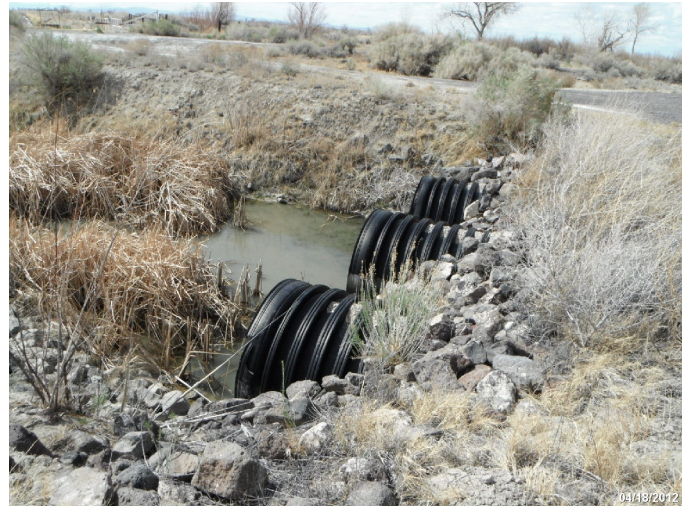
Photo: STIL_C4_1133 Route: 010-001-0.28 Plastic Culvert 40ft long 36in dia. 2ft deep Asset# NA
