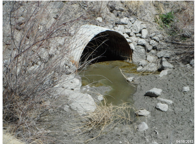
Photo: STIL_C4_1202 Route: 102-004-3.55 Metal Culvert 40ft long 48in dia. 3ft deep Asset# NA
