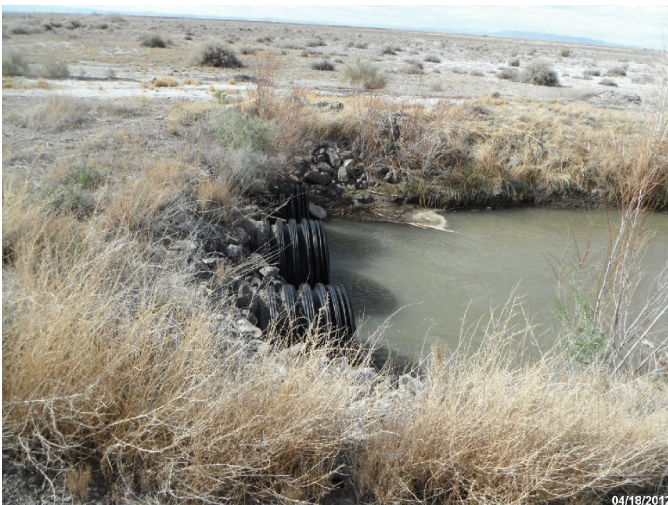
Photo: STIL_C4_1150 Route: 010-007-6.06 Plastic Culvert 40ft long 48in dia. 2ft deep Asset# NA
