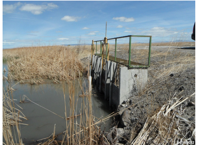
Photo: STIL_C4_1187 Route: 101-005-4.06 Plastic WCS Flap Gate/Full-Round Riser 30ft long 24in dia. 4ft deep Asset# NA
