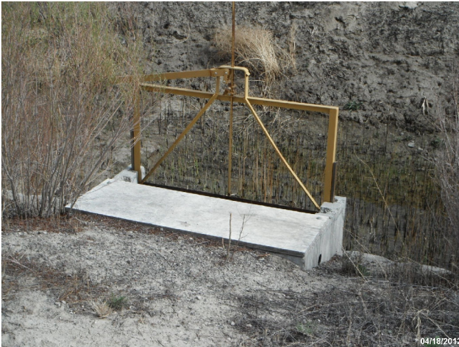
Photo: STIL_C4_1138 Route: 010-003-2.7 Plastic WCS Flap Gate/Full-Round Riser 40ft long 60in dia. 4ft deep Asset# NA
