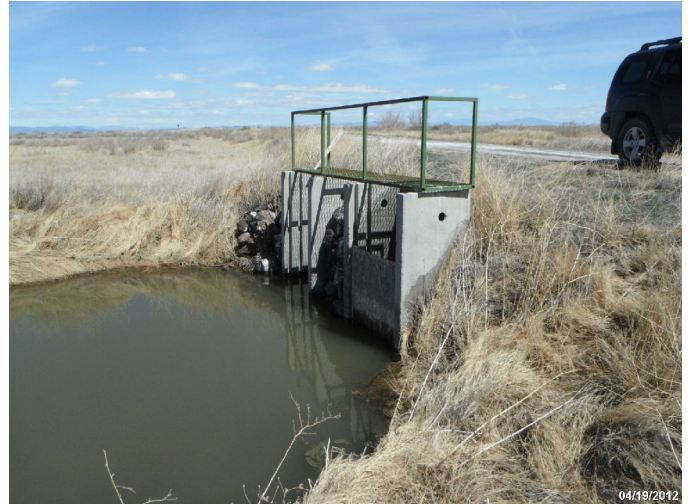
Photo: STIL_C4_1192 Route: 101-005-4.79 Plastic WCS Flashboard Riser 40ft long 24in dia. 4ft deep Asset# NA
