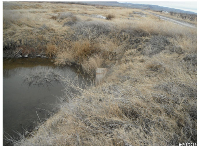
Photo: STIL_C4_1030 Route: 107-002-0.29 Metal WCS Flashboard Riser 40ft long 36in dia. 2ft deep Asset# NA 8-023
