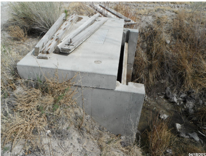
Photo: STIL_C4_1123 Route: 412-006-5.51 Concrete WCS Flashboard Riser 50ft long 48in dia. 3ft deep Asset# NA
