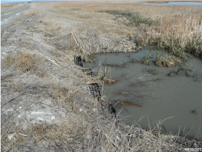
Photo: STIL_C4_1188 Route: 101-005-4.06 Plastic WCS Flap Gate/Full-Round Riser 30ft long 24in dia. 4ft deep Asset# NA
