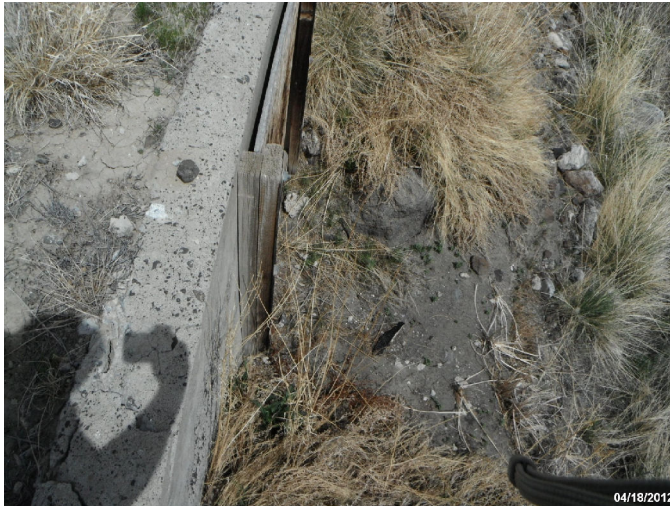
Photo: STIL_C4_1091 Route: 408-003-2.55 Metal WCS Flashboard Riser 30ft long 36in dia. 3ft deep Asset# NA
