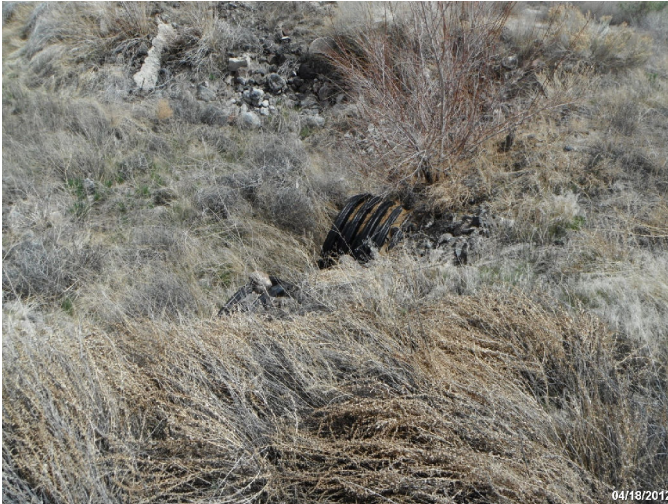
Photo: STIL_C4_1101 Route: 409-001-0.01 Plastic Culvert 30ft long 48in dia. 2ft deep Asset# NA
