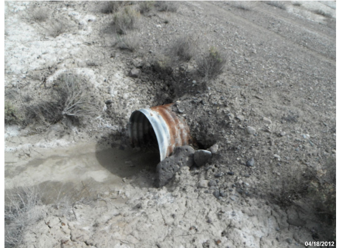
Photo: STIL_C4_1062 Route: 404-001-0.24 Metal Culvert 20ft long 24in dia. 1ft deep Asset# NA
