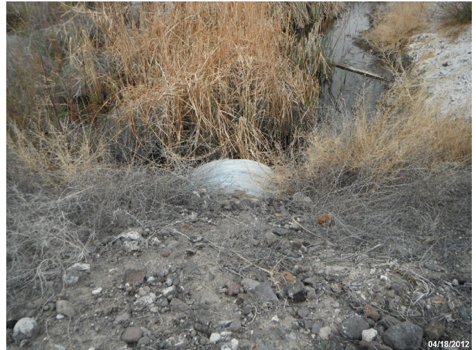
Photo: STIL_C4_1036 Route: 107-003-1.96 Metal Culvert 40ft long 60in dia. 2ft deep Asset# NA
