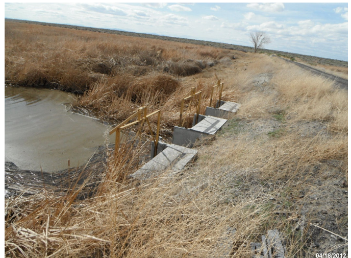
Photo: STIL_C4_1145 Route: 010-005-4.16 Plastic WCS Flap Gate/Full-Round Riser 40ft long 48in dia. 3ft deep Asset# NA
