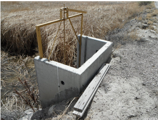
Photo: STIL_C4_1107 Route: 410-002-1.87 Plastic WCS Flap Gate/Full-Round Riser 30ft long 60in dia. 2ft deep Asset# NA
