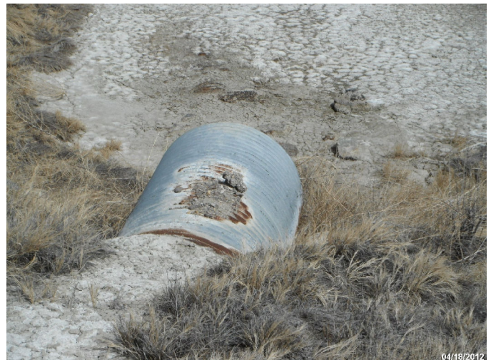
Photo: STIL_C4_1064 Route: 404-001-0.58 Metal WCS Flashboard Riser 50ft long 36in dia. 6ft deep Asset# NA 8-038
