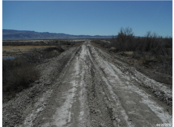
Photo: STIL_C4_1297 Route: 109-003-2.11 Other this is one of the problem areas. The alkali is flowing up and making the road impassable in wet weather photos 1297 - 1298
