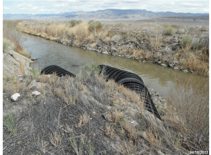
Photo: STIL_C4_1125 Route: 412-006-5.5 Plastic Culvert 120ft long 60in dia. 2ft deep Asset# NA
