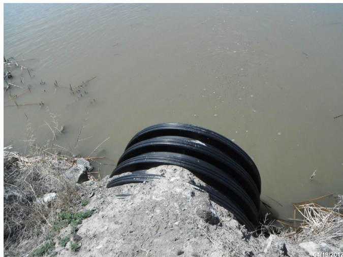
Photo: STIL_C4_1238 Route: 415-001-0.52 Plastic WCS Flashboard Riser 40ft long 48in dia. 1ft deep Asset# NA
