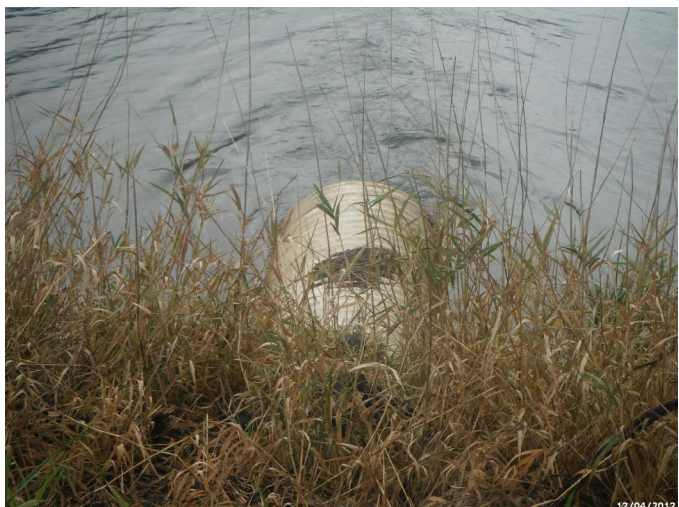
Photo: PIER_C4_4439 Route: 400-004-0.46 Metal WCS Flashboard Riser 60ft long 36in dia. 6ft deep
