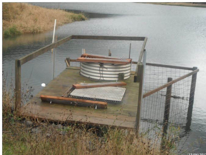
Photo: PIER_C4_4440 Route: 400-004-0.46 Metal WCS Flashboard Riser 60ft long 36in dia. 6ft deep
