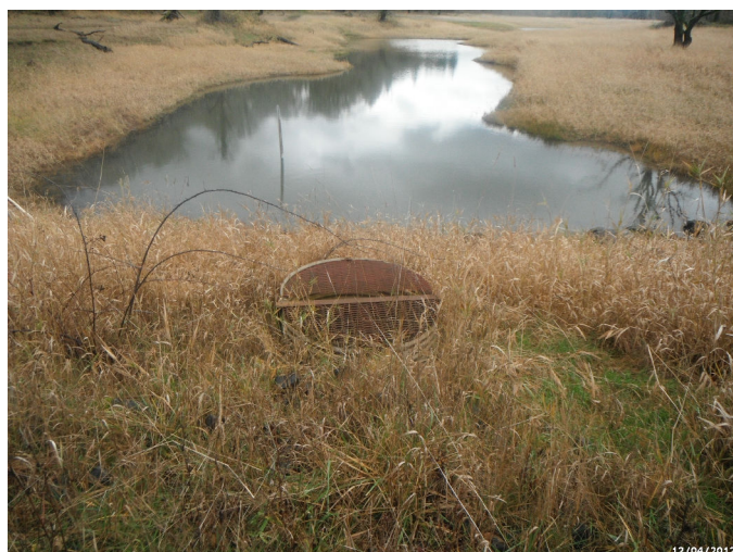
Photo: PIER_C4_4446 Route: 400-006-0.56 Metal WCS Flap Gate/Full-Round Riser 75ft long 36in dia. 10ft deep
