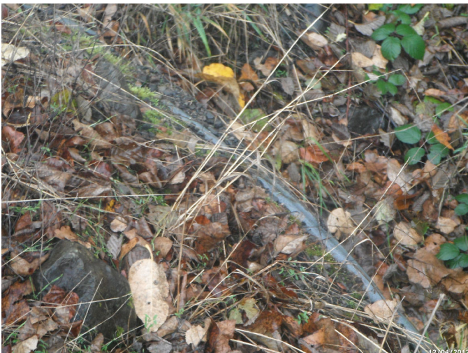
Photo: PIER_C4_4433 Route: 400-001-0.22 Metal Culvert 30ft long 72in dia. 2ft deep
