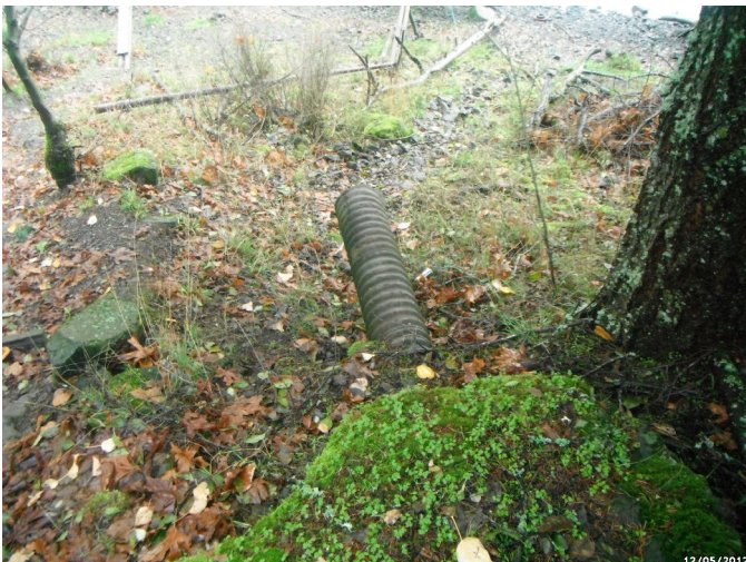
Photo: LISA_C4_4457 Route: 010-001-0.65 Metal Culvert 50ft long 12in dia. 2ft deep
