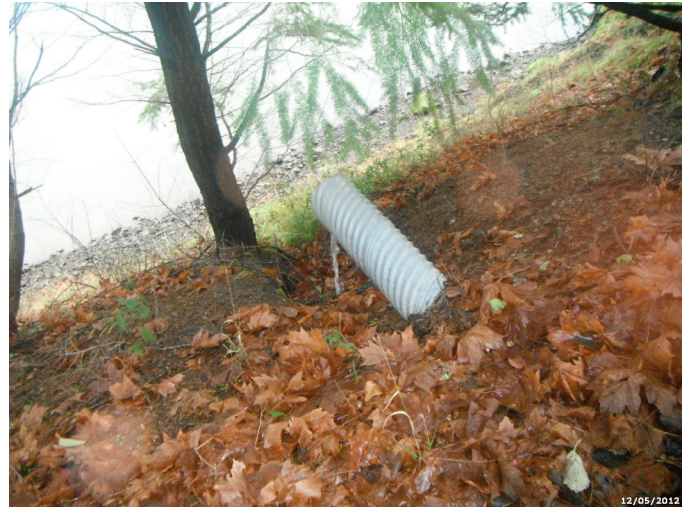
Photo: LISA_C4_4454 Route: 010-001-0.57 Metal Culvert 40ft long 6in dia. 1ft deep
