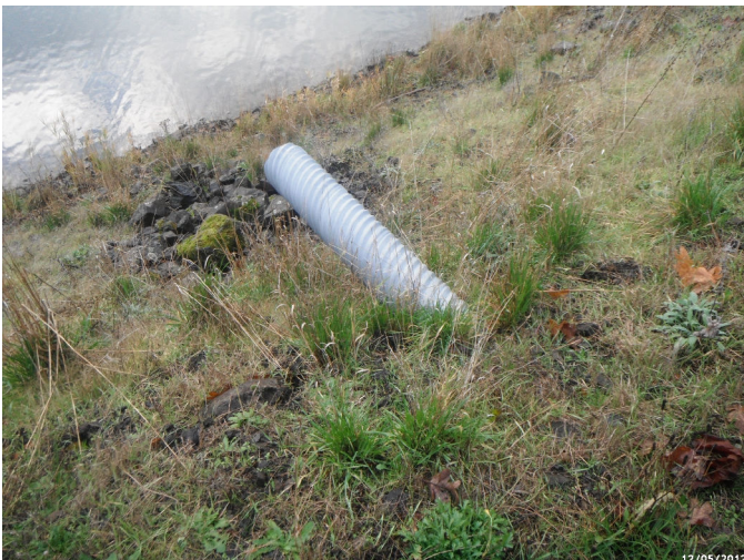
Photo: LISA_C4_4463 Route: 010-001-0.77 Metal Culvert 40ft long 6in dia. 2ft deep
