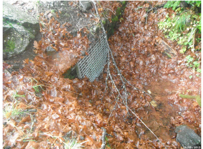
Photo: LISA_C4_4460 Route: 010-001-0.72 Metal Culvert 60ft long 18in dia. 2ft deep
