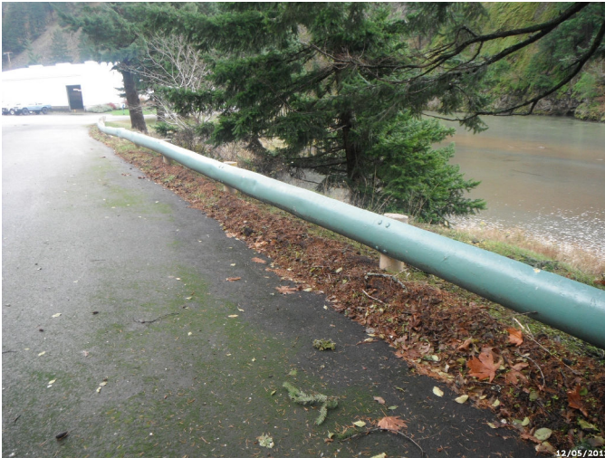
Photo: LISA_C4_4475 Route: 010-001-0.82 Guard_Guide_Rail Guardrail Galvanized_Steel 110.0 ft long Asset# 10038138
