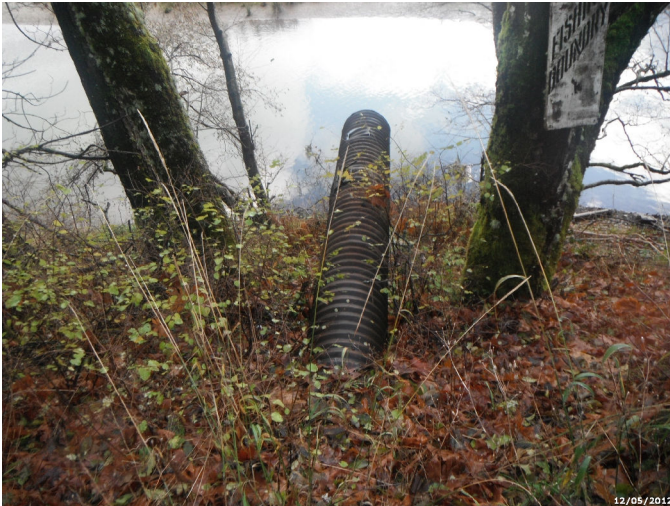
Photo: LISA_C4_4459 Route: 010-001-0.69 Metal Culvert 50ft long 12in dia. 2ft deep
