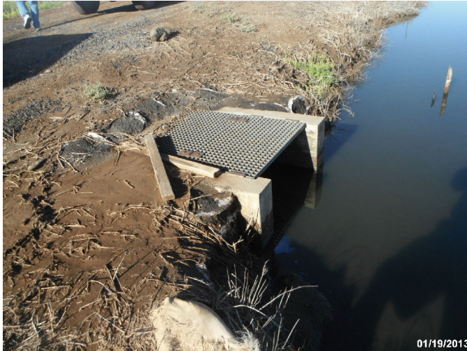
Photo: PEHA_C4_1061 Route: 400-001-0.36 Concrete WCS Flashboard Riser 22ft long 18in dia. 2ft deep Asset# NA
