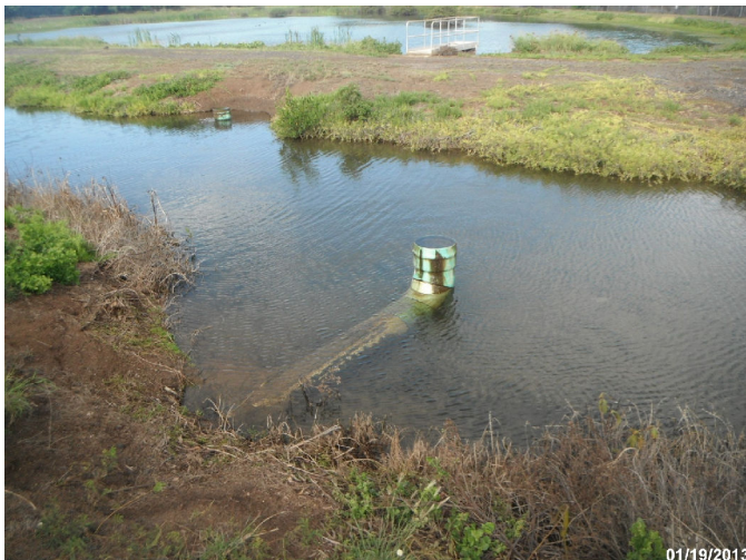
Photo: PEHA_C4_1074 Route: 401-001-0.6 Plastic WCS Flashboard Riser 40ft long 18in dia. 2ft deep Asset# NA
