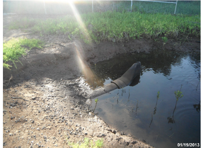
Photo: PEHA_C4_1062 Route: 400-001-0.36 Concrete WCS Flashboard Riser 22ft long 18in dia. 2ft deep Asset# NA
