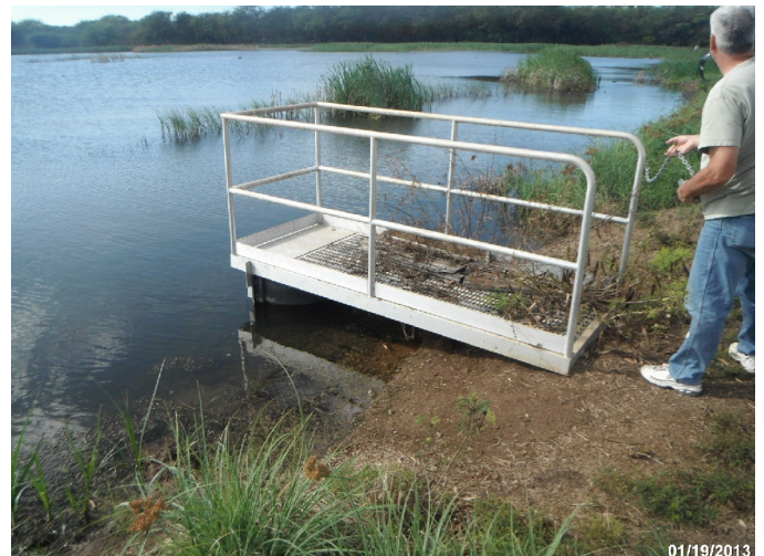
Photo: PEHA_C4_1075 Route: 401-001-0.6 Plastic WCS Flashboard Riser 40ft long 18in dia. 2ft deep Asset# NA 8-003
