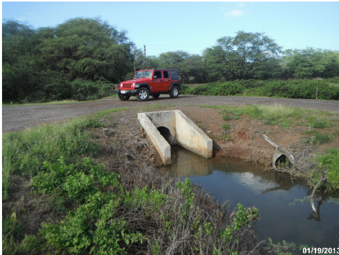
Photo: PEHA_C4_1072 Route: 401-001-0.06 Concrete Culvert 30ft long 36in dia. 2ft deep Asset# NA
