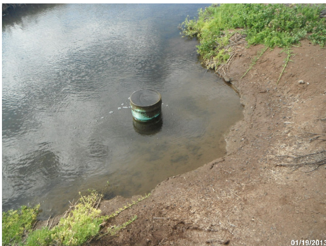
Photo: PEHA_C4_1080 Route: 401-002-0.15 Plastic WCS Flashboard Riser 45ft long 18in dia. 3ft deep Asset# NA
