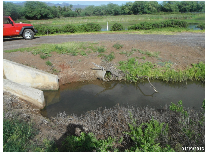
Photo: PEHA_C4_1077 Route: 401-002-0.06 Concrete Culvert 40ft long 18in dia. 3ft deep Asset# NA
