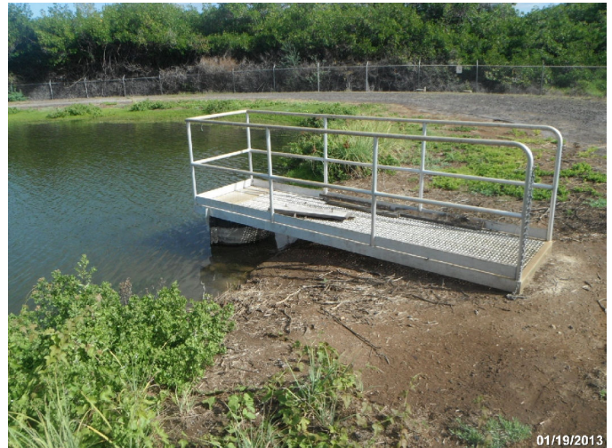
Photo: PEHA_C4_1079 Route: 401-002-0.15 Plastic WCS Flashboard Riser 45ft long 18in dia. 3ft deep Asset# NA
