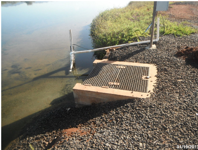
Photo: PEHA_C4_1065 Route: 400-002-0.29 Concrete WCS Flashboard Riser 25ft long 18in dia. 1ft deep Asset# NA
