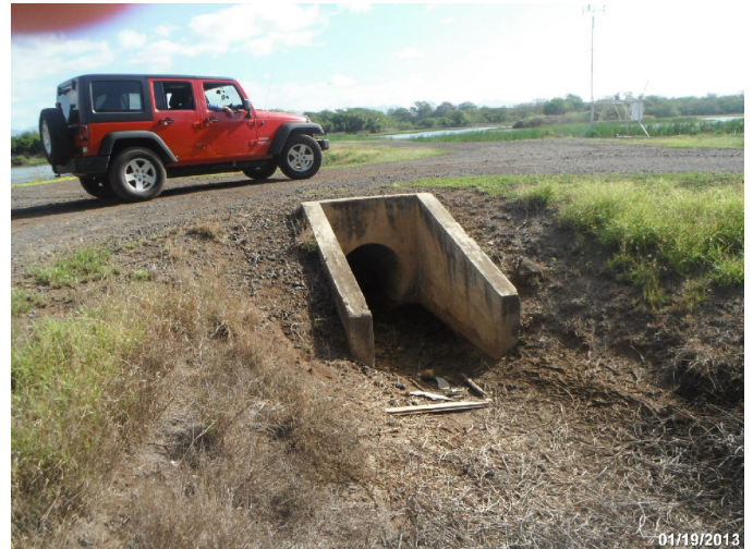
Photo: PEHA_C4_1073 Route: 401-001-0.06 Concrete Culvert 30ft long 36in dia. 2ft deep Asset# NA
