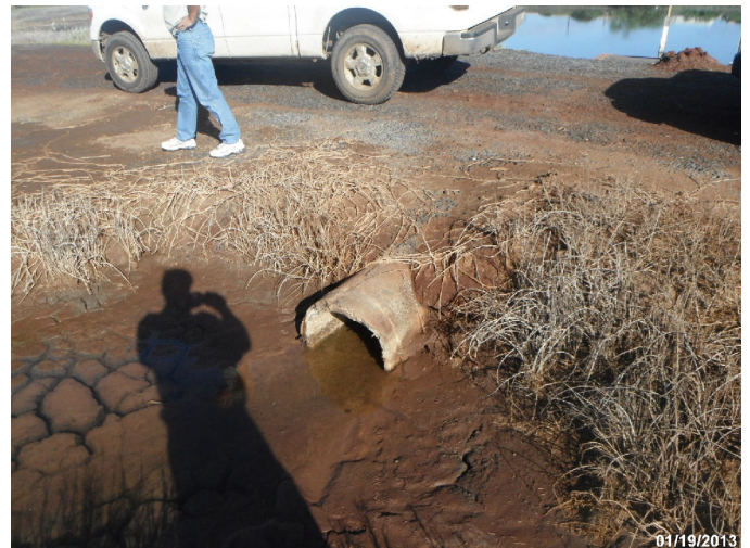
Photo: PEHA_C4_1064 Route: 400-002-0.29 Concrete WCS Flashboard Riser 25ft long 18in dia. 1ft deep Asset# NA 8-001
