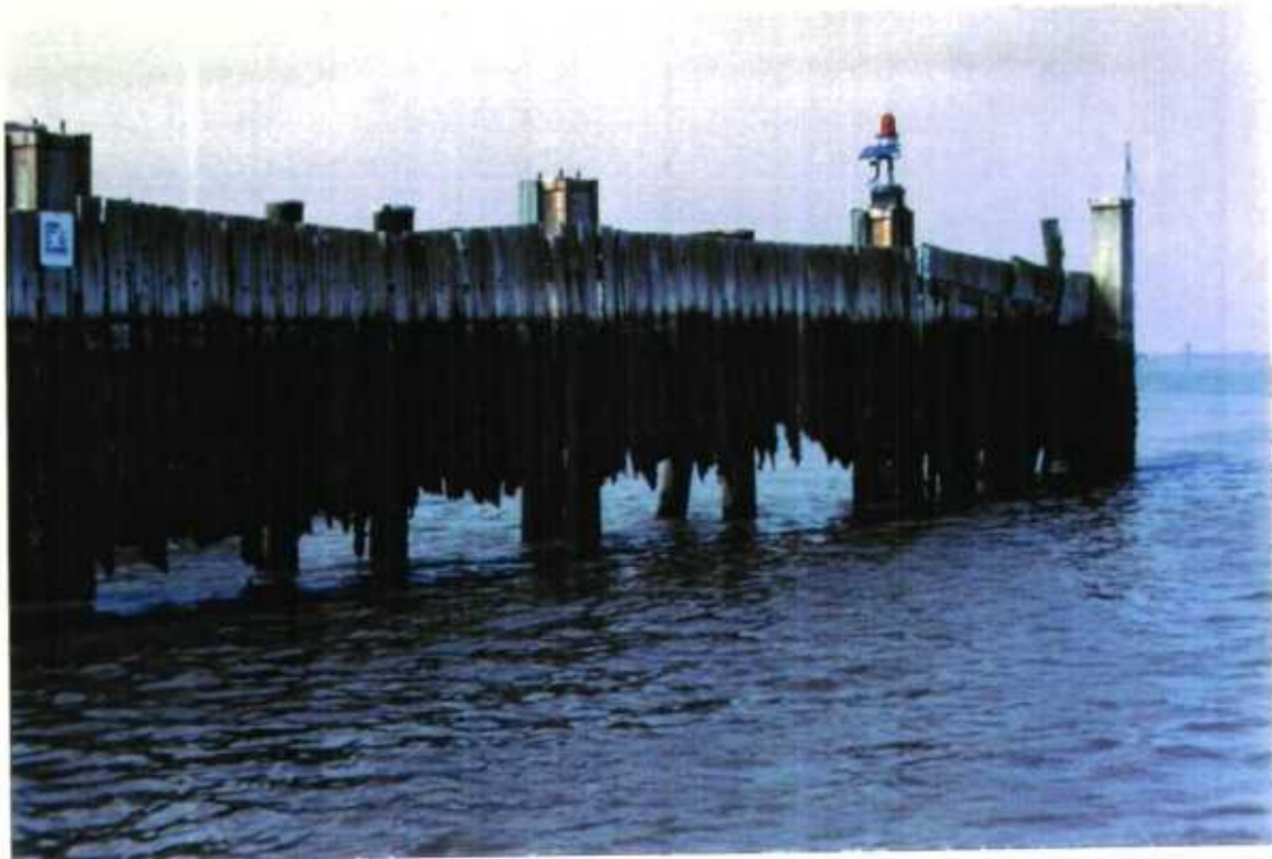
The pier breakwall was replaced due to deterioration by saltwater, before...
