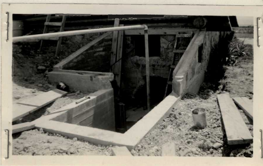
Showing pump in pit and opening partially cut thru wall Roll # 8, Exp. # 2, taken 7/19/42
