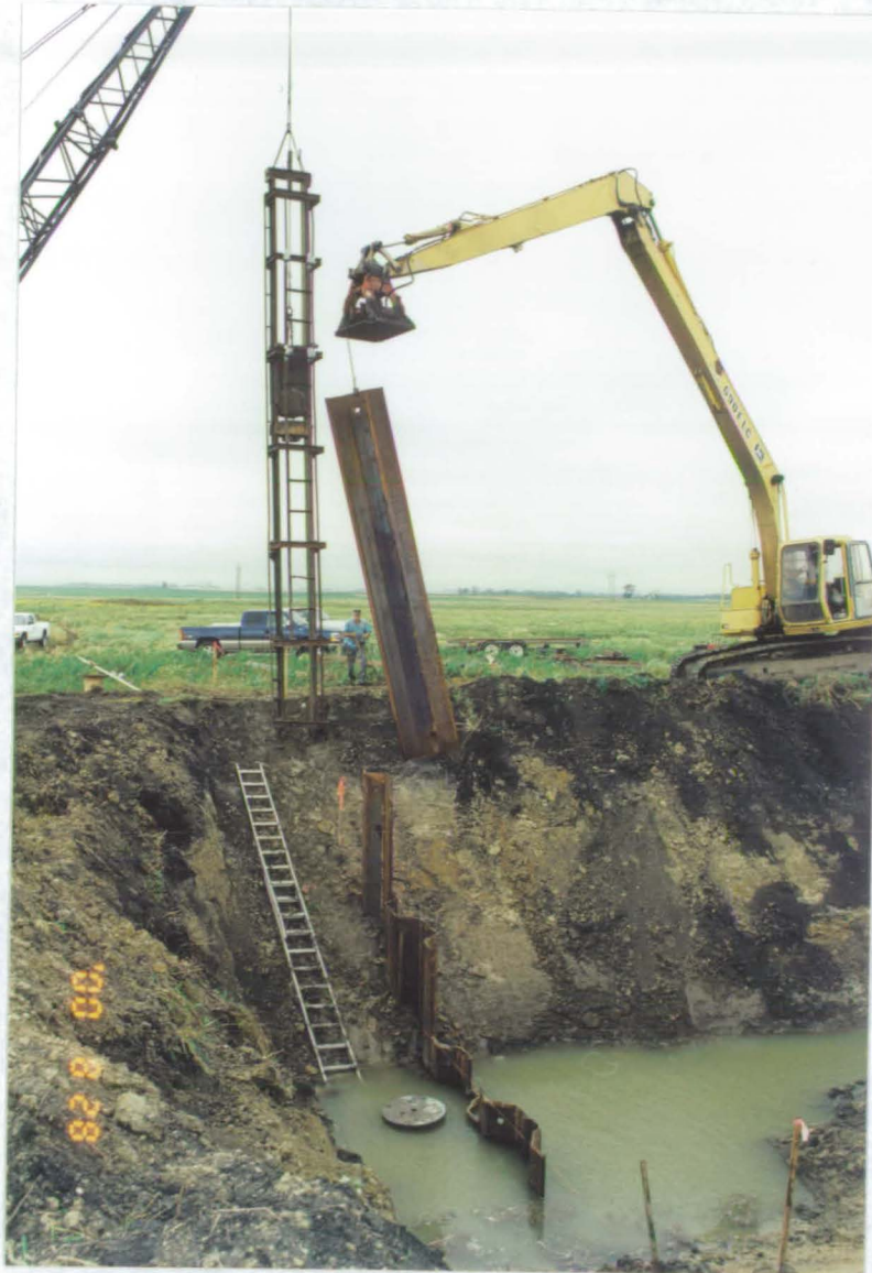
#00-25-19. Sheet metal pilings being driven for Bisson Lake structure. (MTM 9/00)
