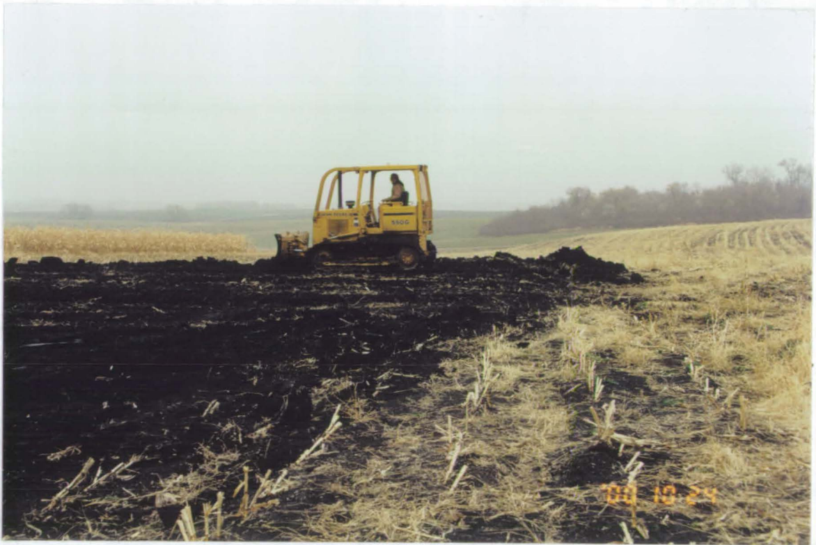
#00-30-19. Tamarac EO Tom Franklin building a ditch plug on the south end of the refuge. (MTM 10/00)
