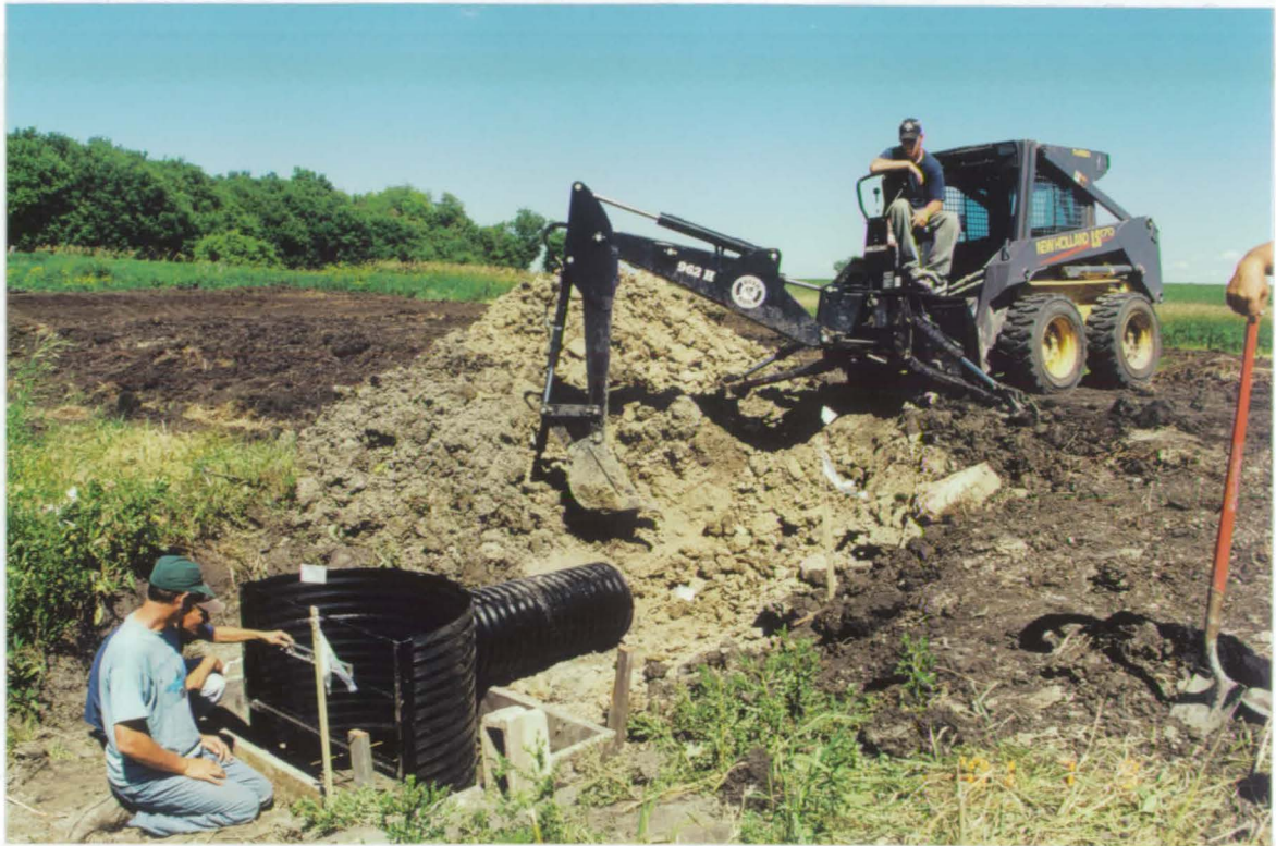
#01-12-24. SWCD personnel assisting contractor with installation of school's water control structure. (MTM 07/01)
