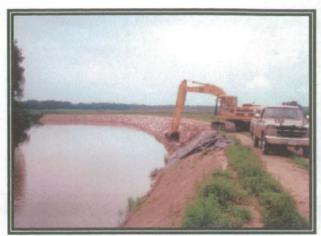
A total of 1,500 linear feet of Pool 1A dike was resloped and fortified with riprap. 8/9/99
