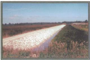
Pool 2 dike improvements included elevating the dike and riprap placement on the slopes 8/18/99 EPD
