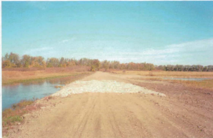
North Marsh dike and spillway following renovation. (EPD 10/2000)
