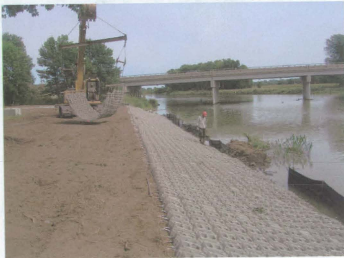
Engineering Equipment Operator Butch Nowosatko and Tractor Operator David Peters prepared the area before they installed the woven mats of concrete.
