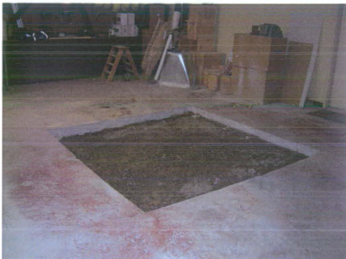
Floor drains removed from two buildings to eliminate potential for contaminant run-off. Photo by ED.
