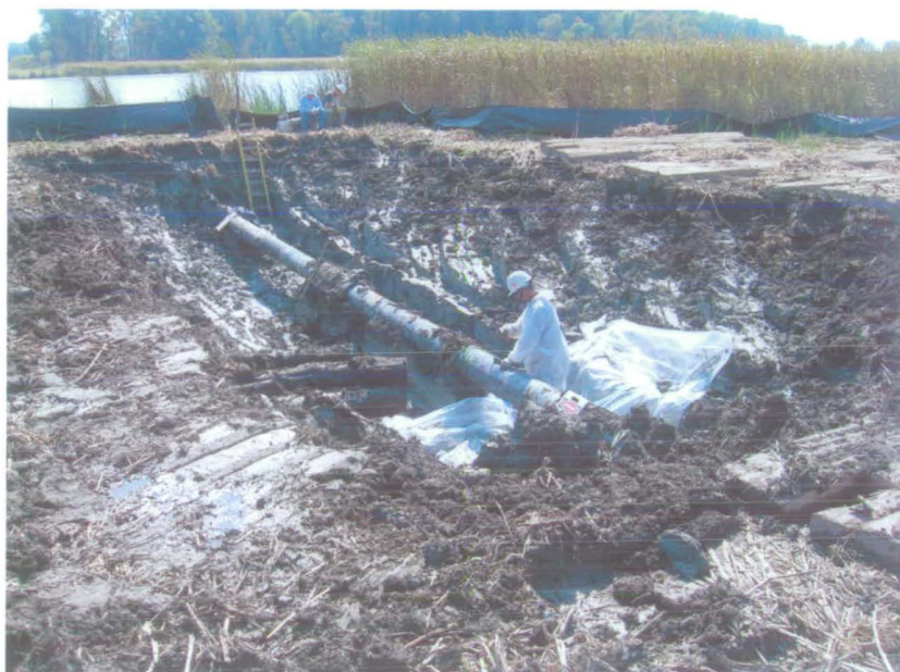
Consumers Energy pipeline repair on North side of Shiawassee River. Photo by EPD, 09/18/07.
