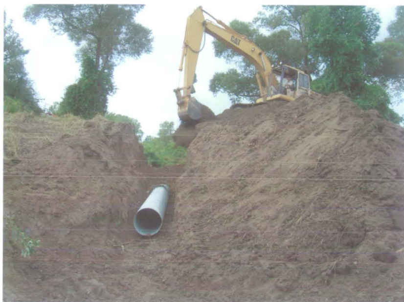
Culvert replacement on the Ferguson Bayou Nature Trail. Photo by EPD, 08/23/07.
