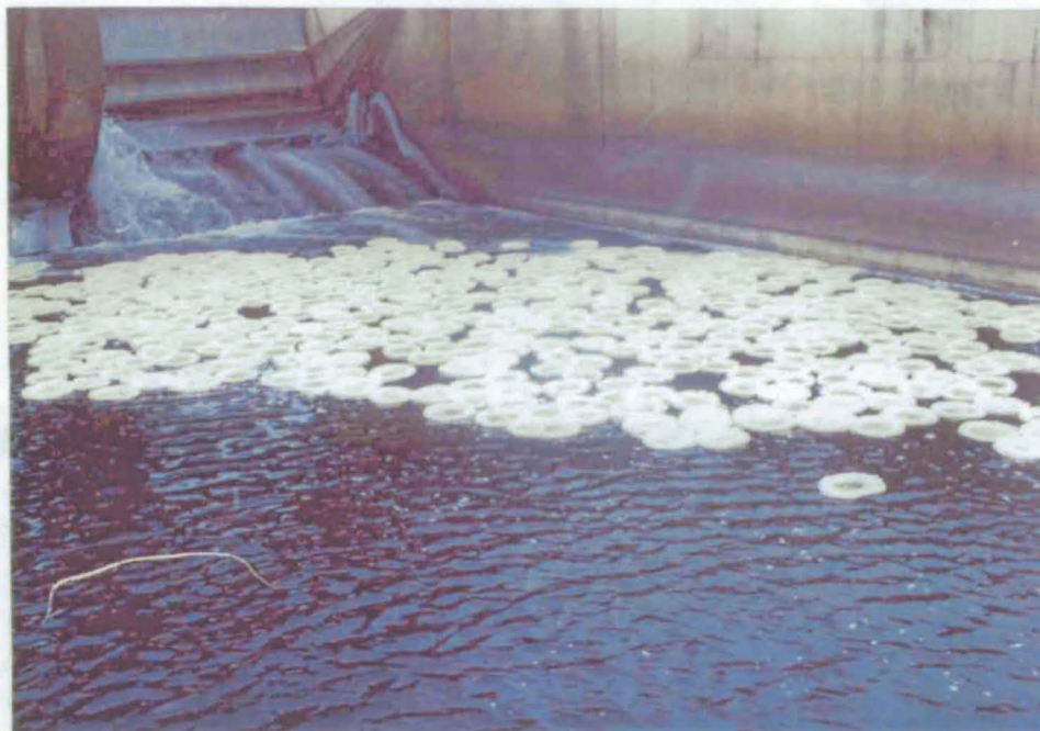
Pancake ice downstream of radial gates at St. Francis Pool (AR 4/03)
