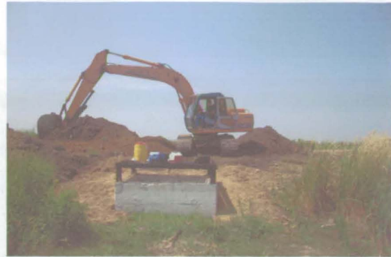
Repair included clay and rip rap being totally placed around box riser.
