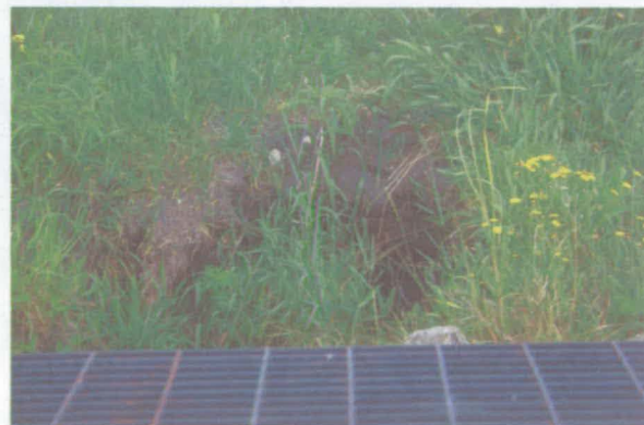
Washout of culvert in wetland 12-1. Notice no rip rap on slope.
