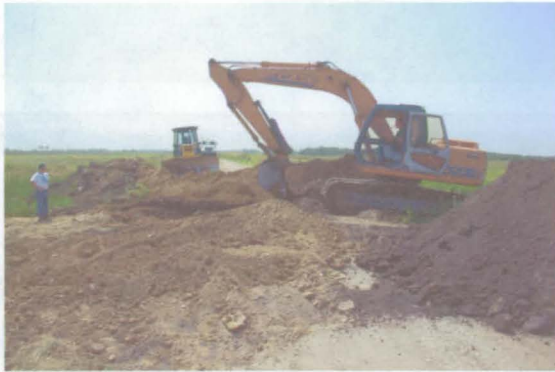
Complete embedding of pipe with clay was needed to replace sand.
