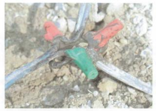
Diamond Traffic Products recommended tar to seal the splice. JB Weld Quickset epoxy or similar flexible epoxy was used to seal the splice. It provided a cleaner and quicker method than tar. After the two parts of the epoxy were mixed you had approximately 5 minutes to seal the splice before the epoxy set. The photo shows the sealed splice for the counter at Lisbon. Wire nuts were used in this case but butt splices were more effective and easier to tape after
