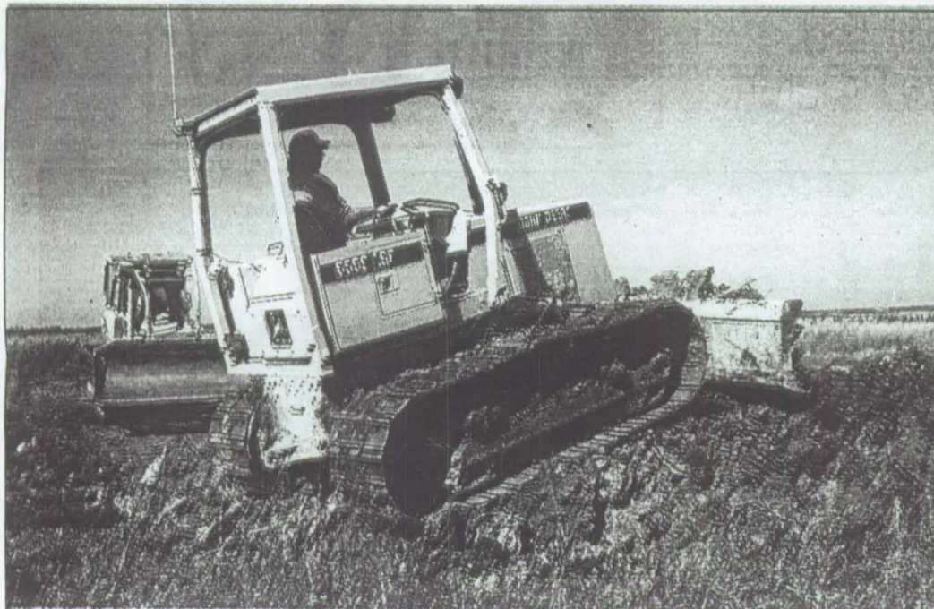
▲ Ralph McKeever (front), a heavy equipment contractor from Middle River, Minn., and Dave Myhrer , who runs heavy equipment for Agassiz National Wildlife Refuge, construct a ditch plug to restore a wetland at a site in Marshall County.
