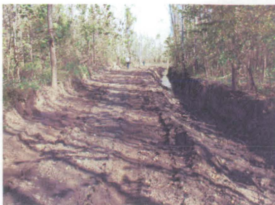
Condition of the access road to Jameson Island Chute in October, 2007 (left), and July 2008 (right). The road became a stream channel during the flooding in July.
