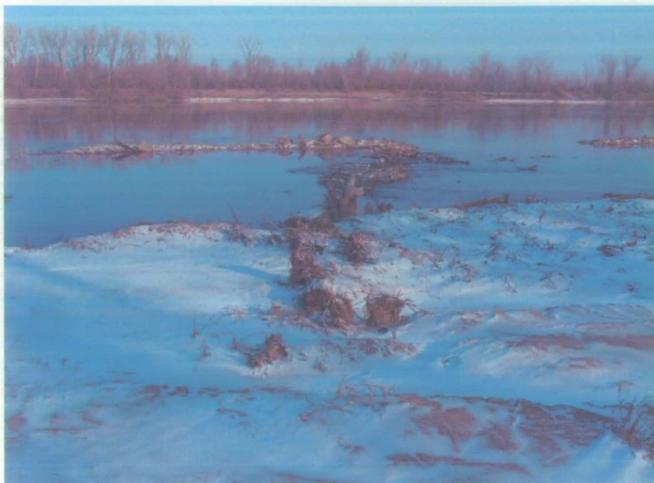
Partially complete bank notch at RM 300.4
