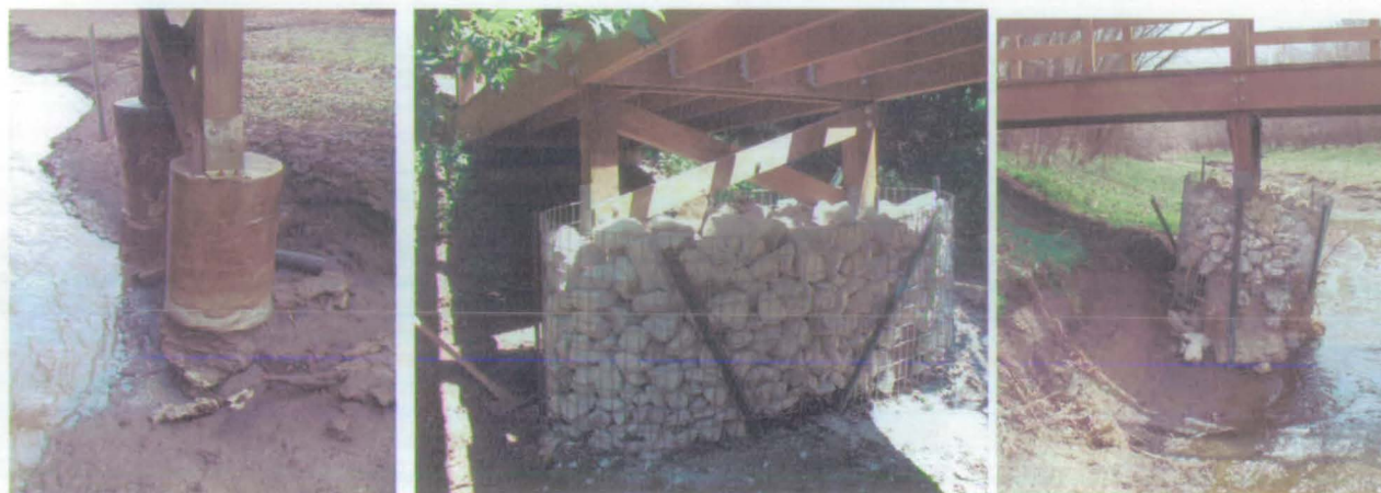
The center piers of the bridge for the Arrow Rock Historic Landing Trail started to erode as shown in pictures from July 2007 (left), March 2008 (center), and September 2008 (right).
