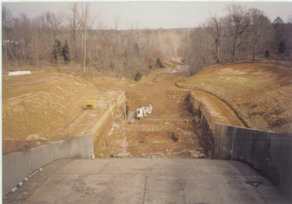
In order to minimize the risk of a dam failure major reconstruction work was initiated on the Little Grassy Dam and stilling basin.
