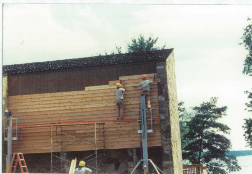
The Refuge administrative office was resided this year. Because the old siding was warped and not properly installed, the building developed water leaks.
