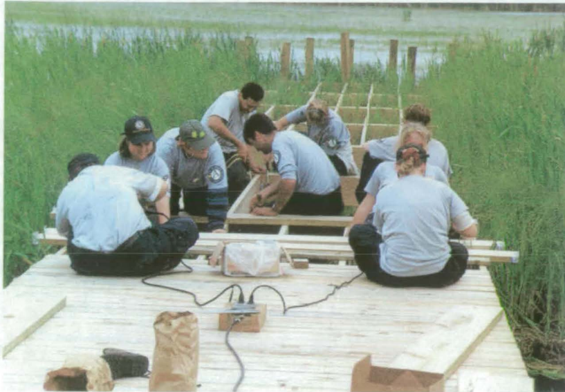
AmeriCorps Crew installing deck boards on the boardwalk.
