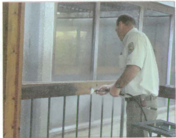
Cedar wood siding of Visitor Center was pressure washed and then treated with stain sealer. Rex Stambaugh applying stain sealer PHOTO: USFWS\staff photo
