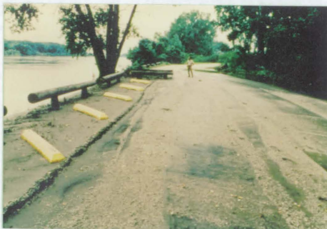
At the new Missouri River Overlook, only light siltation and erosion occurred, whereas, in the flooded woods, the deposits were much heavier. 27-100-93 GG
