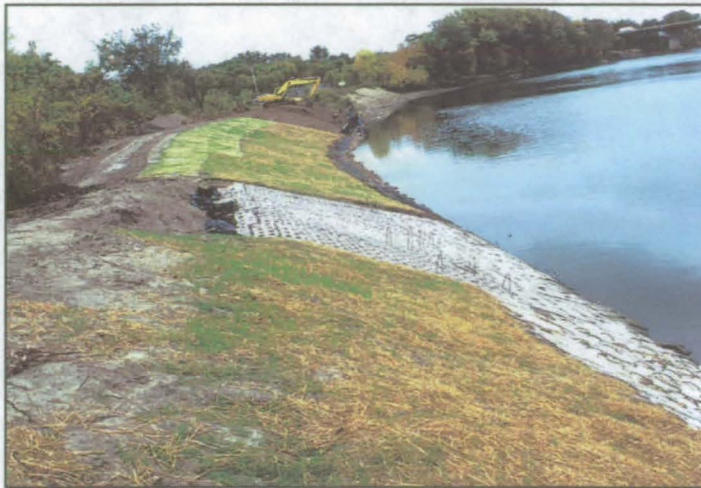
Photo 10. Bank stabilization on the Black Dog Unit. Photo by T. Schreiner.
