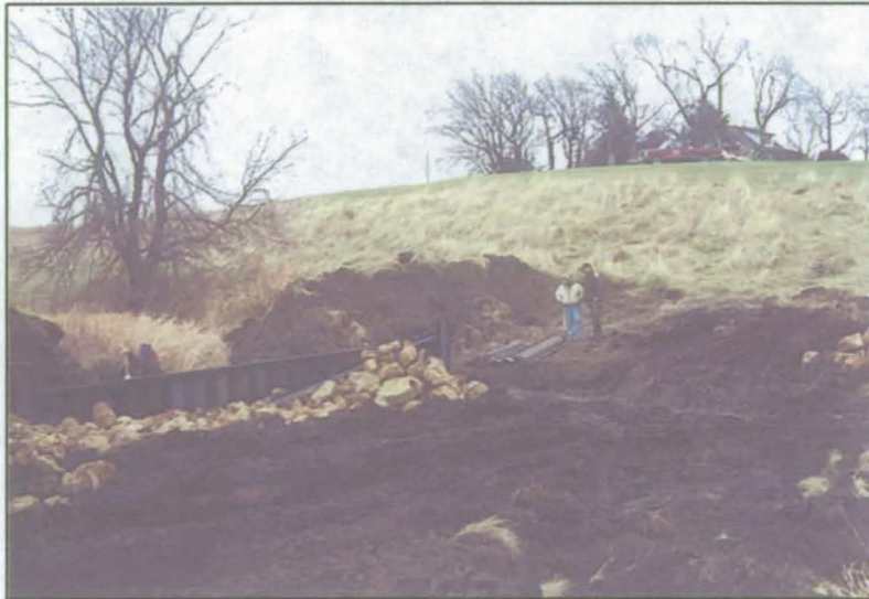
Photo 4. Sheet pile structure being installed at Cihak habitat easement. Photo by M. Malling.
