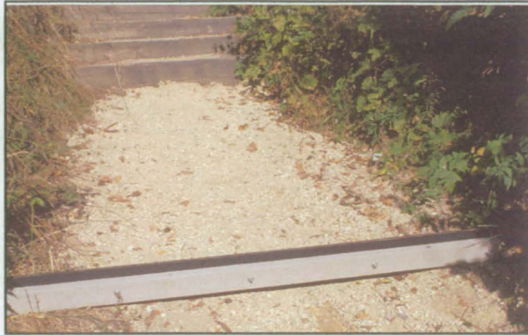
Photo 15. Water bars installed on Hillside trail before backfilling to grade. Photo by T. Schreiner.
