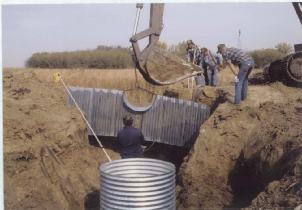
Setting the drop-inlet water control structure on the Roger Granberg restoration. 92-25 10/92 Dennis Hall
