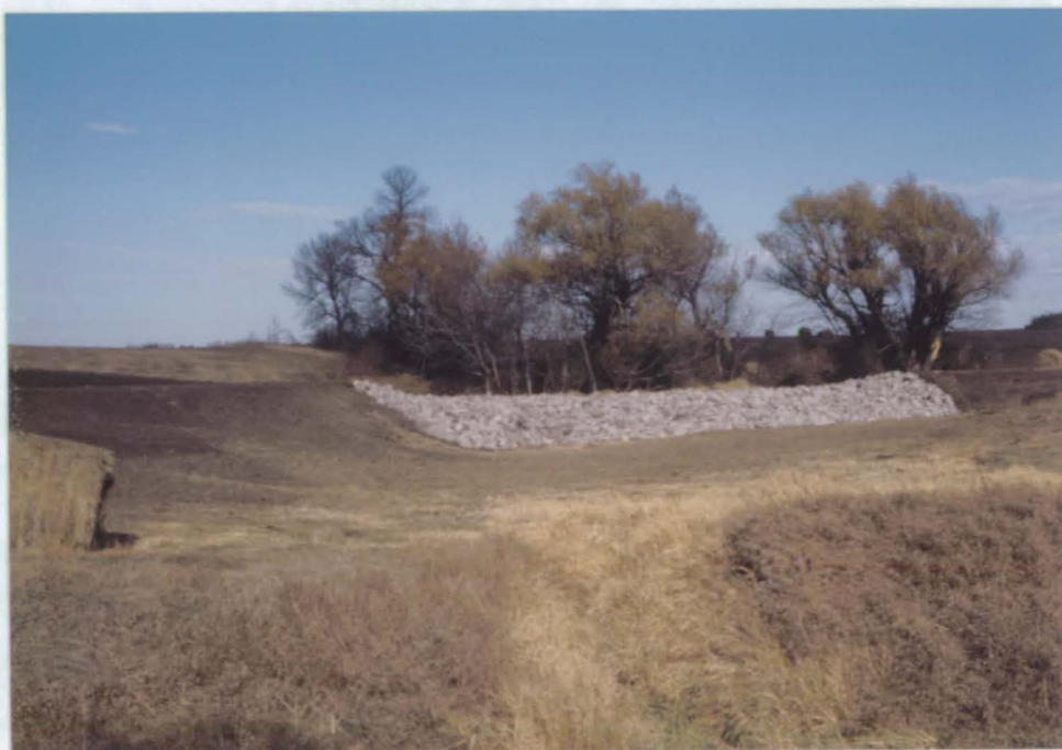
A rock spillway instead of a deep inlet water control structure was used on the Louis Paulson restoration because of the large watershed and limited water storage area.
