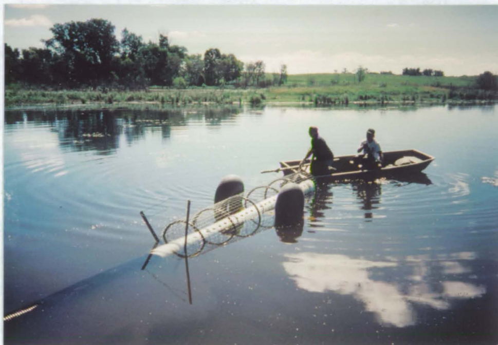
Installing a Clemson Beaver Pond Leveler. 95-19 7/95 DDH
