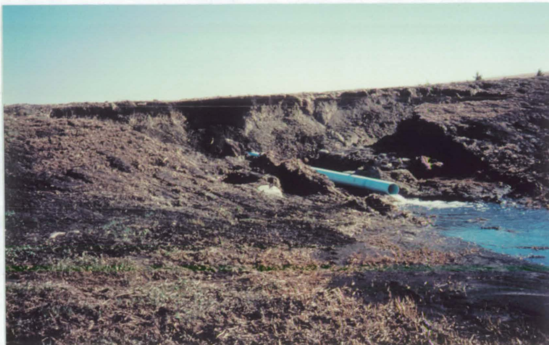
Washout on the John Scharf restoration following the spring flood. 97-8 4/97 BLA
