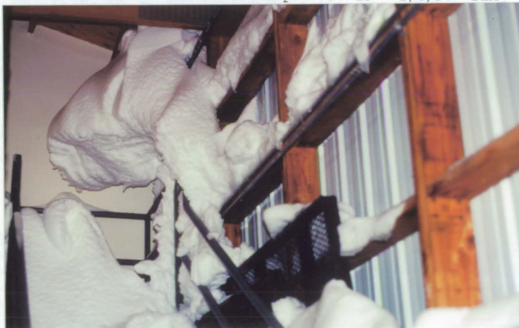
Snow blown into building through damaged soffit. 97-30 1/17/97 BLA
