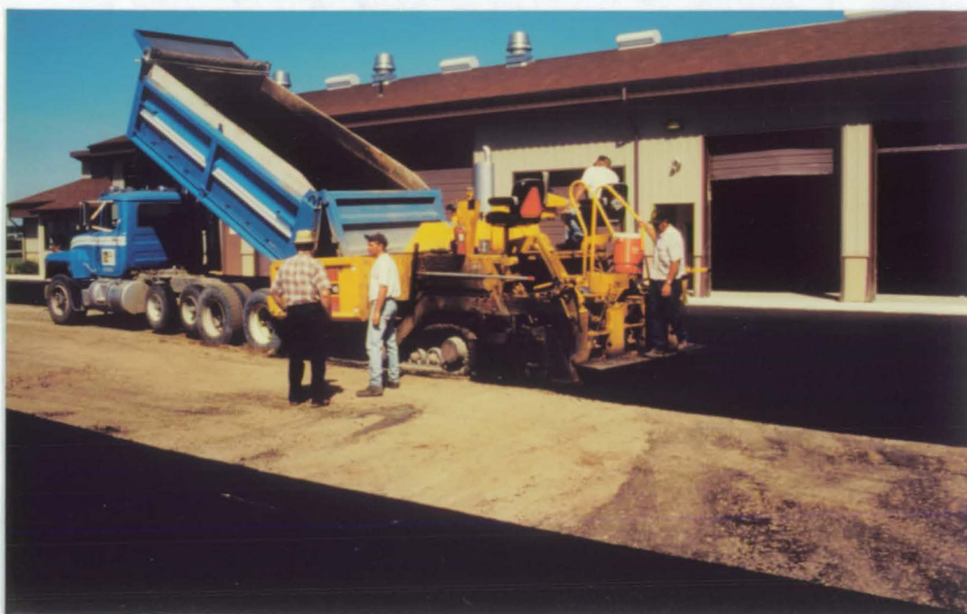
Re-surfacing shop parking area after tile drainage system was installed. 97-26 8/7/97 BLA
