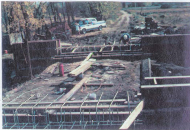
Forms for construction for concrete pouring on new bridge at the Louisville Unit. Photo: Terry Schreiner.
