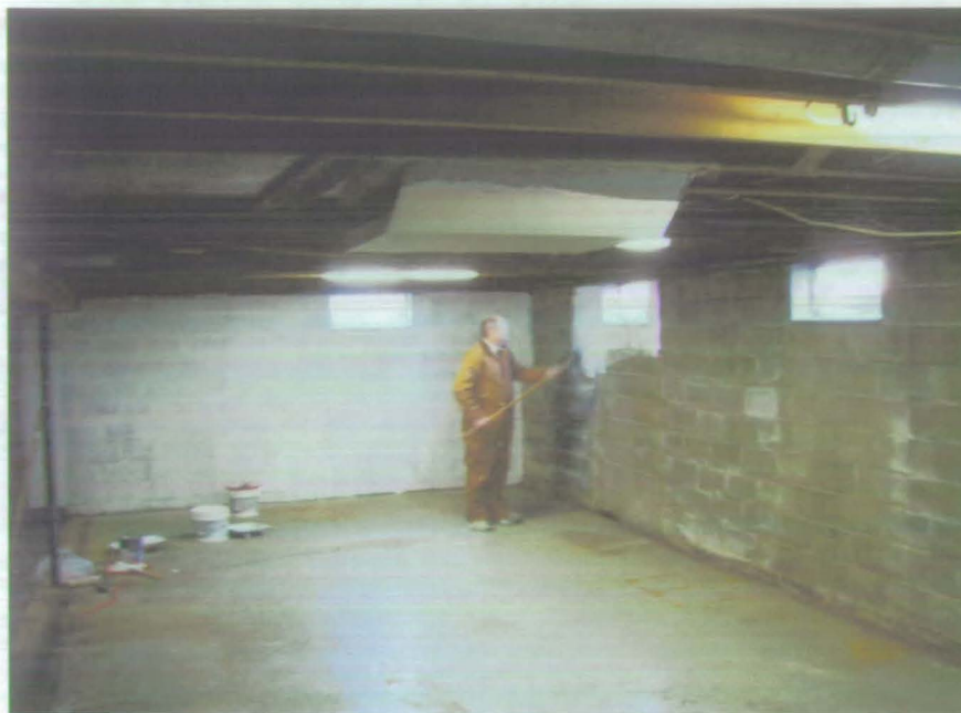
ASA Rarey sealing the walls and floor. Credit: T. Dailey
