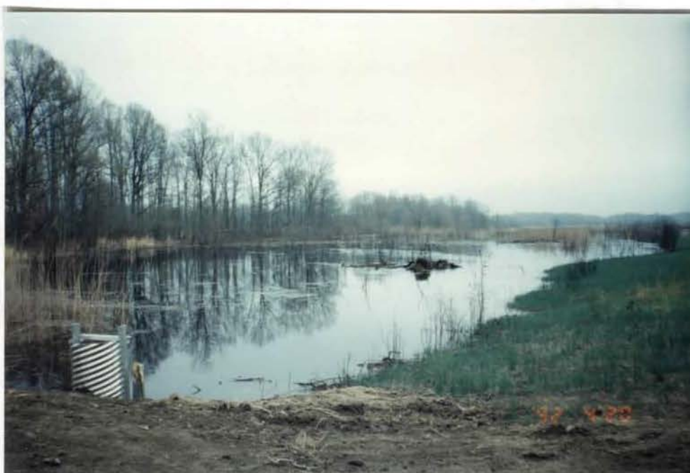
#29 After installation of the new culvert/WCS and repairs to the low levee on the east side of Pool A, fresh water can be pumped into the 12 acre pool with excellent results (view to south). 4/92 Daly
