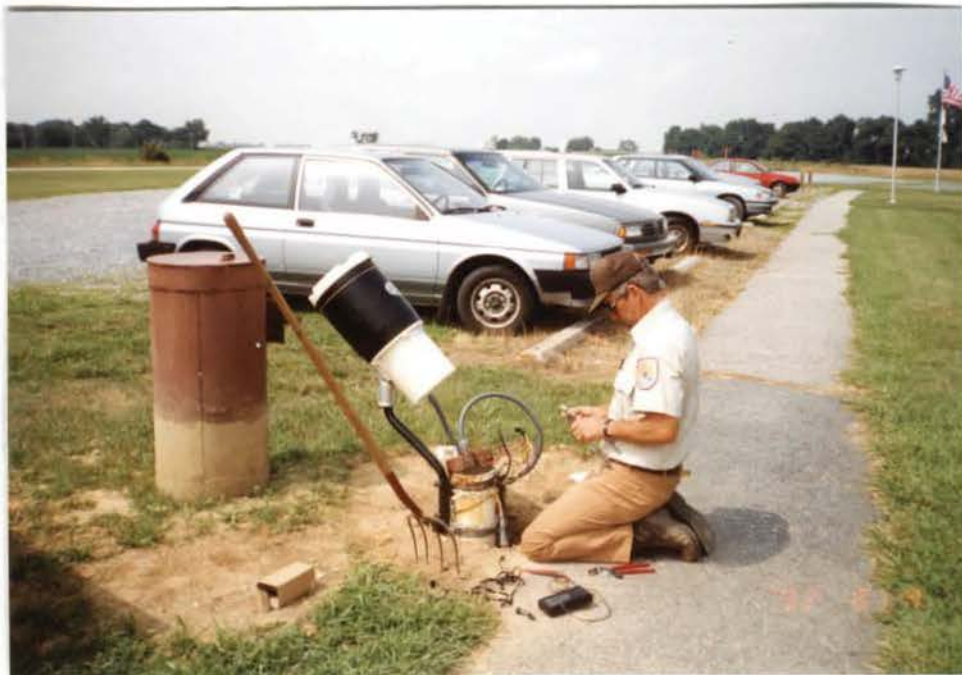
#1 Maintenance Worker Straughn installs the new automatic chlorinator at the Headquarters Building well. 8/92 Daly
