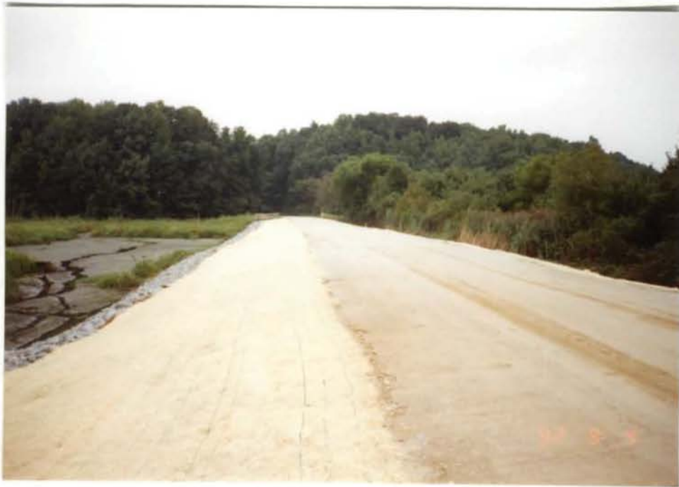
#25 Finally, grass seed was sown on the slopes and mulch was placed down. Gravel was then spread on the dike (roadway) top.
