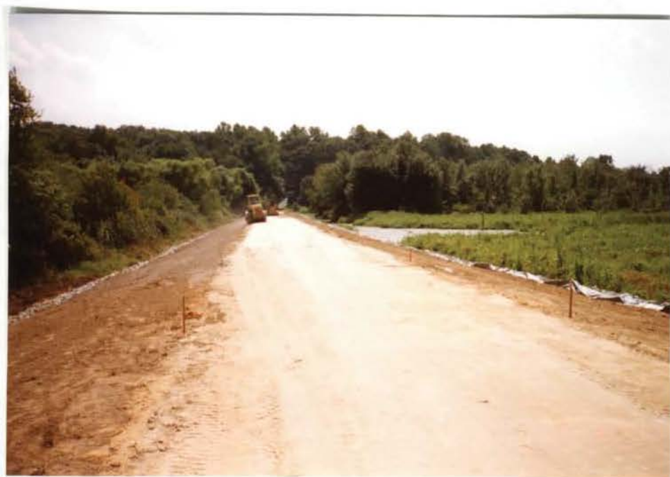
#24 The dike was raised with material hauled in from offsite, slopes were graded, and both dike toes were rip-rapped.
