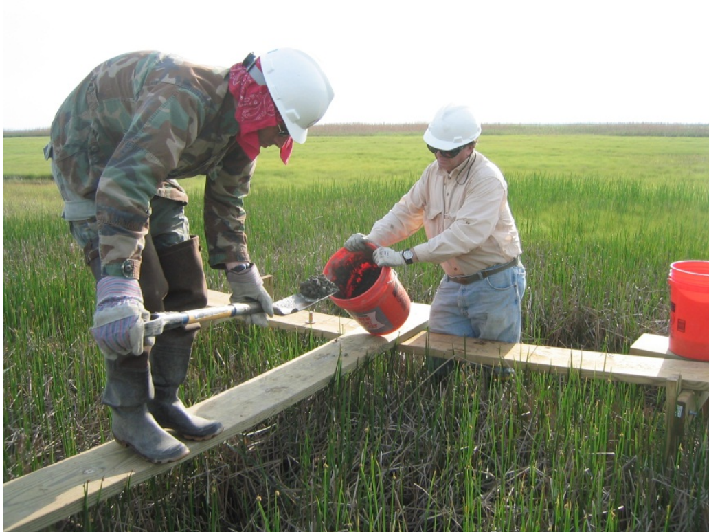
Figure 3.26. Adding cement (Fishing Bay WMA, MD, USA).
