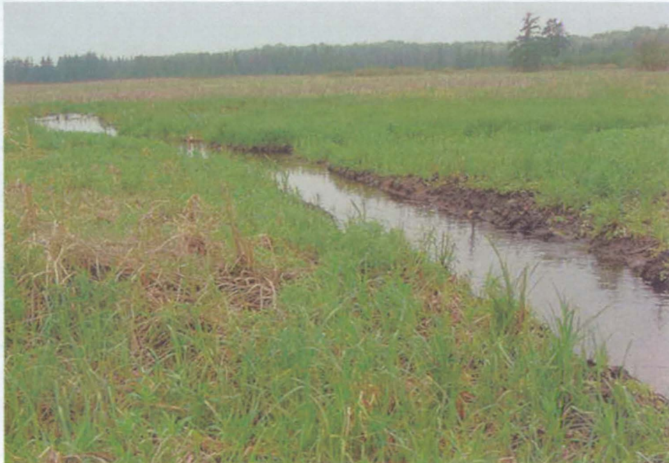
Pilot channel used to re-establish historic course of Eggleston Creek and restore 70 acres of Refuge wetlands (5/20/04).
