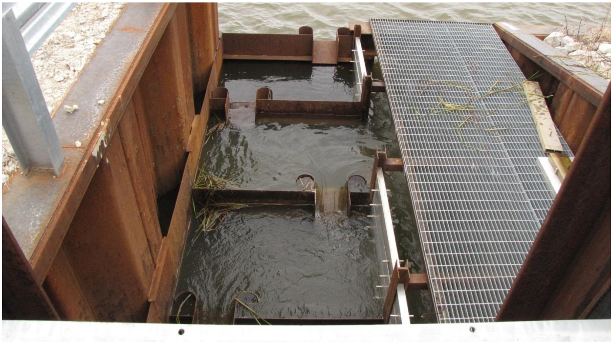
Figure 23 Ottawa NWR Complex, Blausey Unit fish ladder in operation. Stop logs allow wetland unit to be managed at a variety of water levels while maintaining connectivity for fish.
